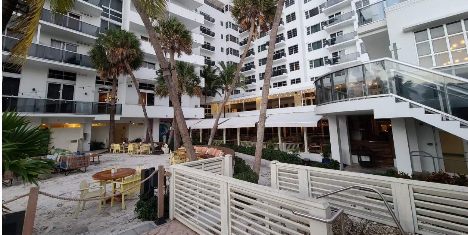
SECOND FLOOR ACCESS
