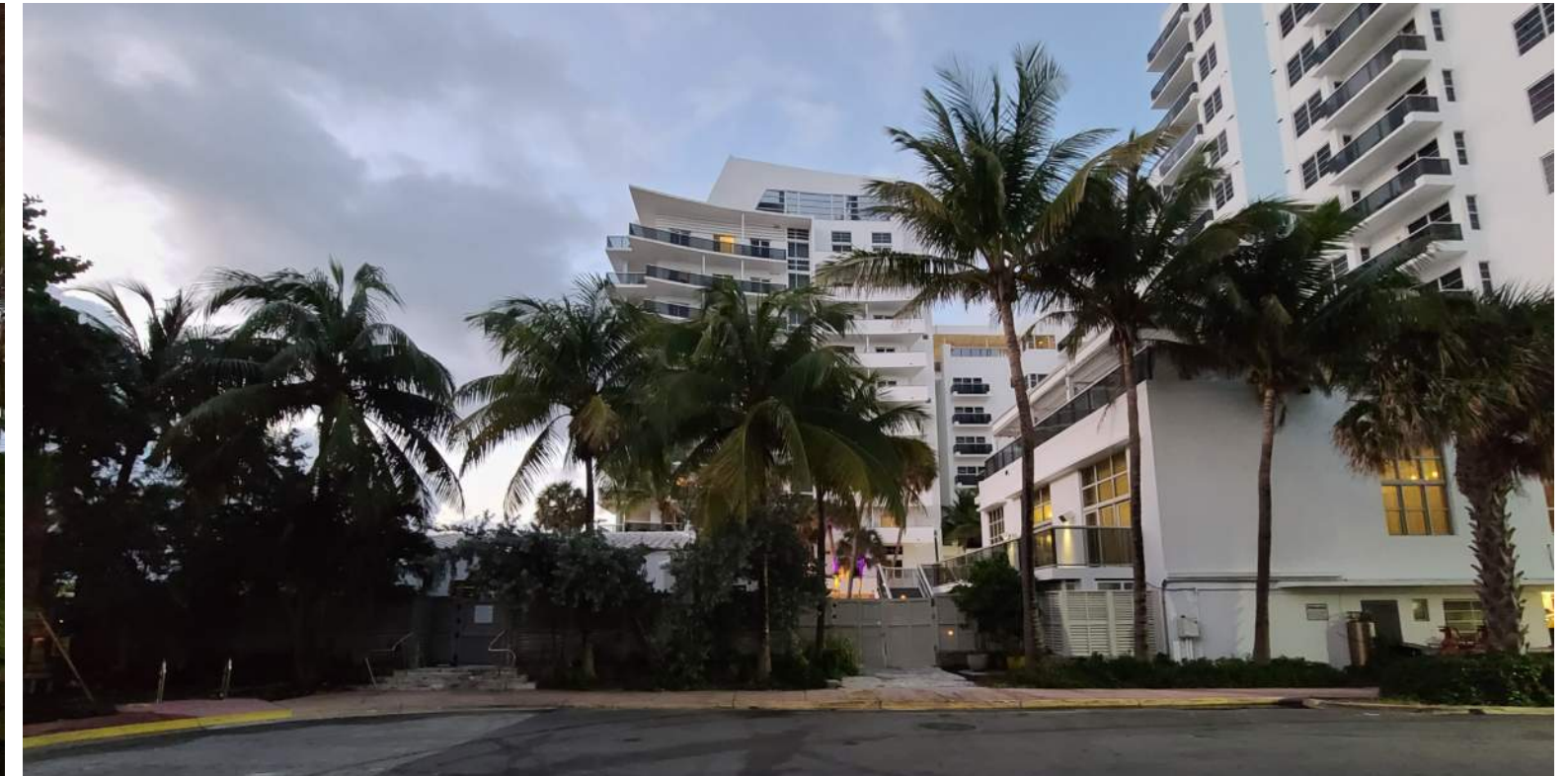
NORTH FACADE 1930'S HOUSE ENTRANCE AND EGRESS EXIT TO 41ST STREET
