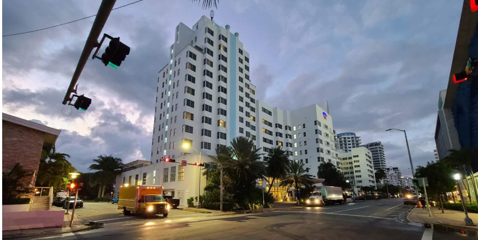
NORTH WEST FACADE
