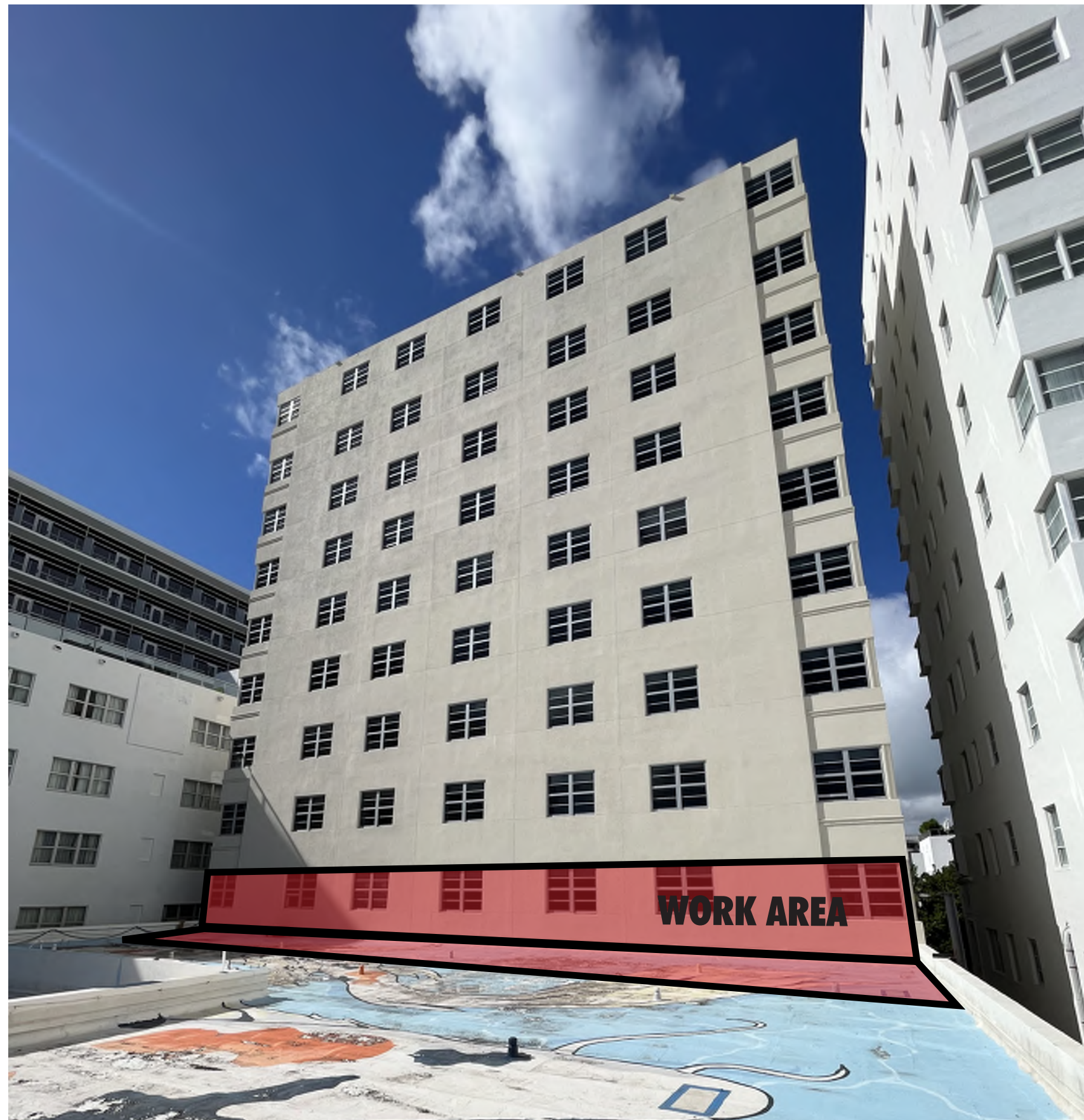
PHOTO AT 3RD FL. ROOF LEVEL
