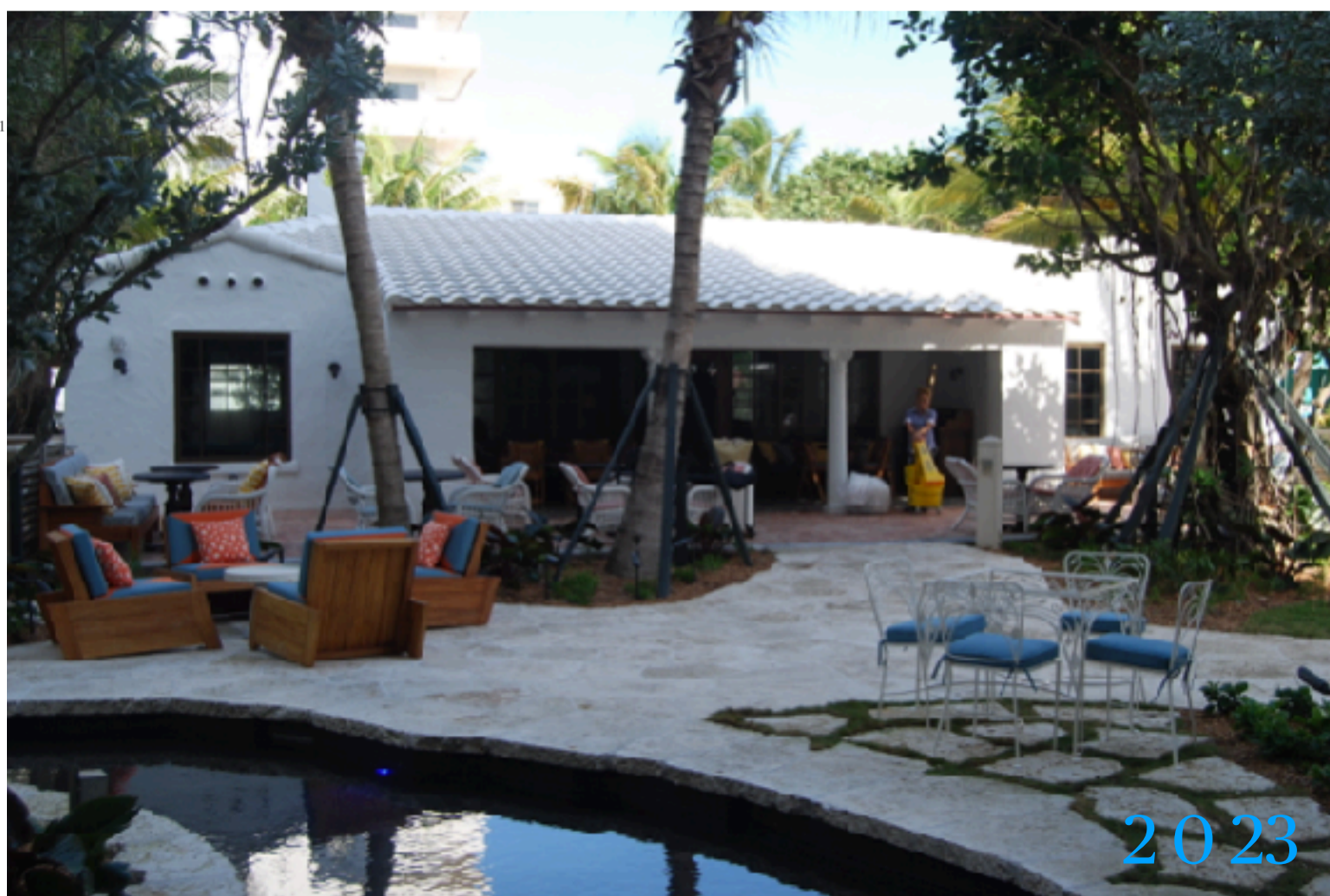
SOUTH ELEVATION OF HISTORIC COTTAGE. (7)
