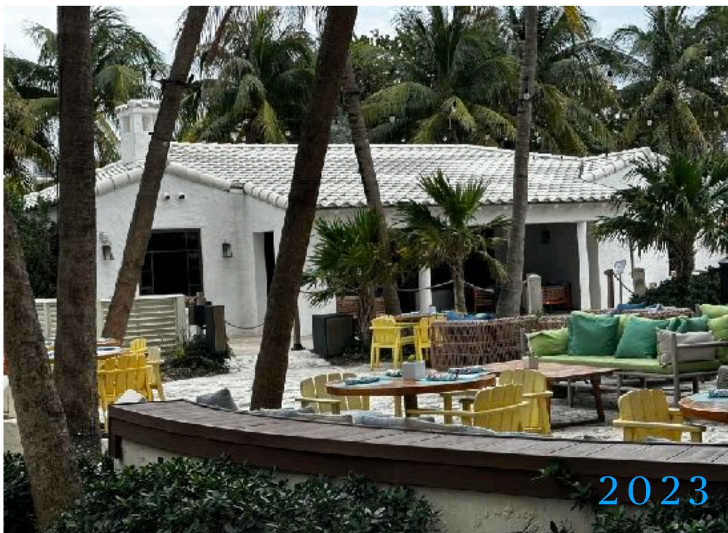
VIEW ACROSS COURTYARD TO SOUTH ELEVATION OF HISTORIC COTTAGE. (7)
