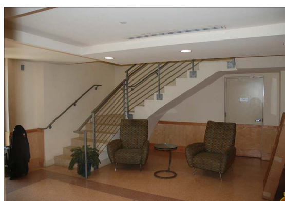
1940s ENTRY LOBBY - EXISTING CONDITIONS - PICTURES
