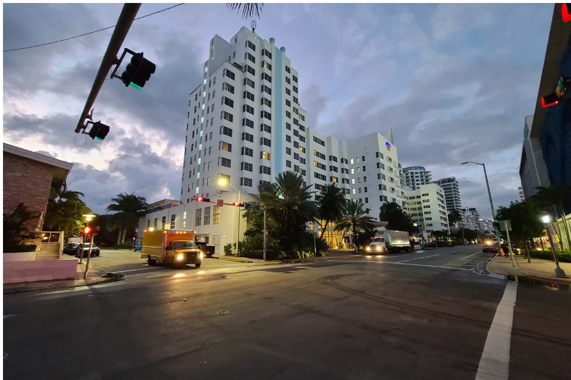
NORTH WEST FACADE
