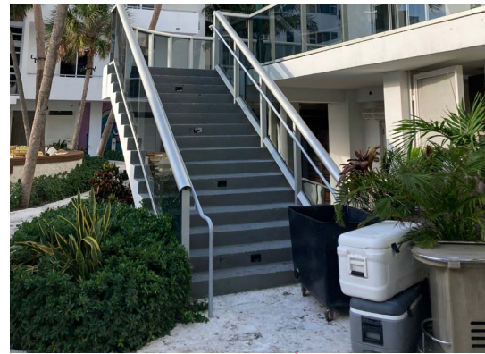
2ND FLOOR ACCESS
