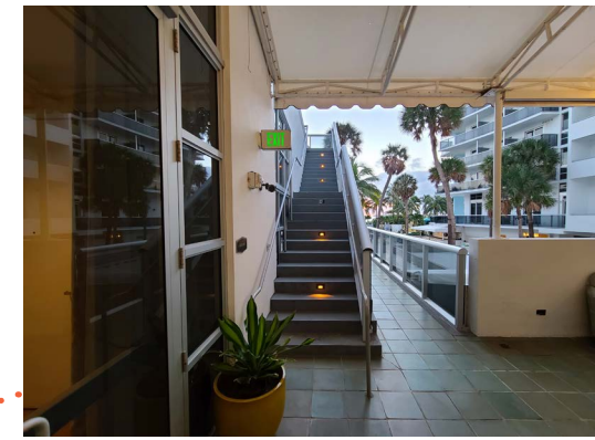
STAIRS TO 4TH FLOOR
