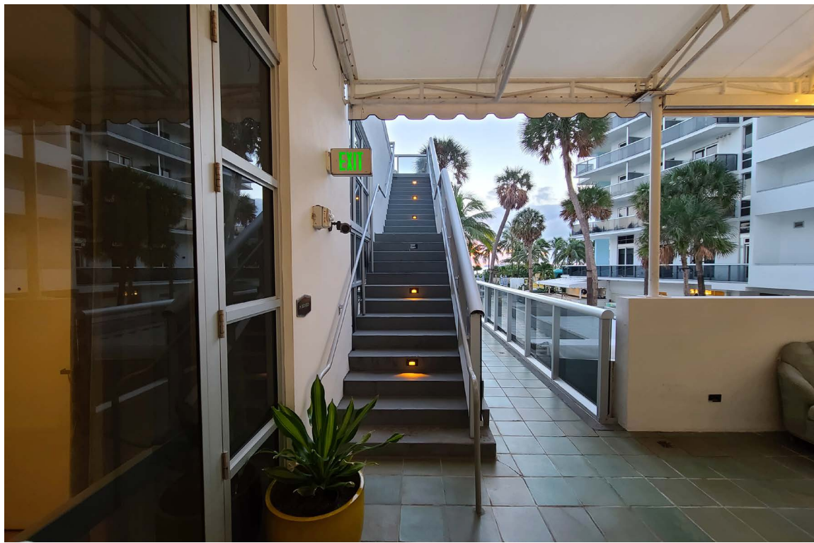
STAIRS TO 4TH FLOOR
