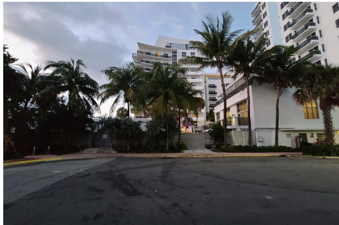
NORTH FACADE 1930'S HOUSE ENTRANCE AND EGRESS EXIT TO 41ST STREET
