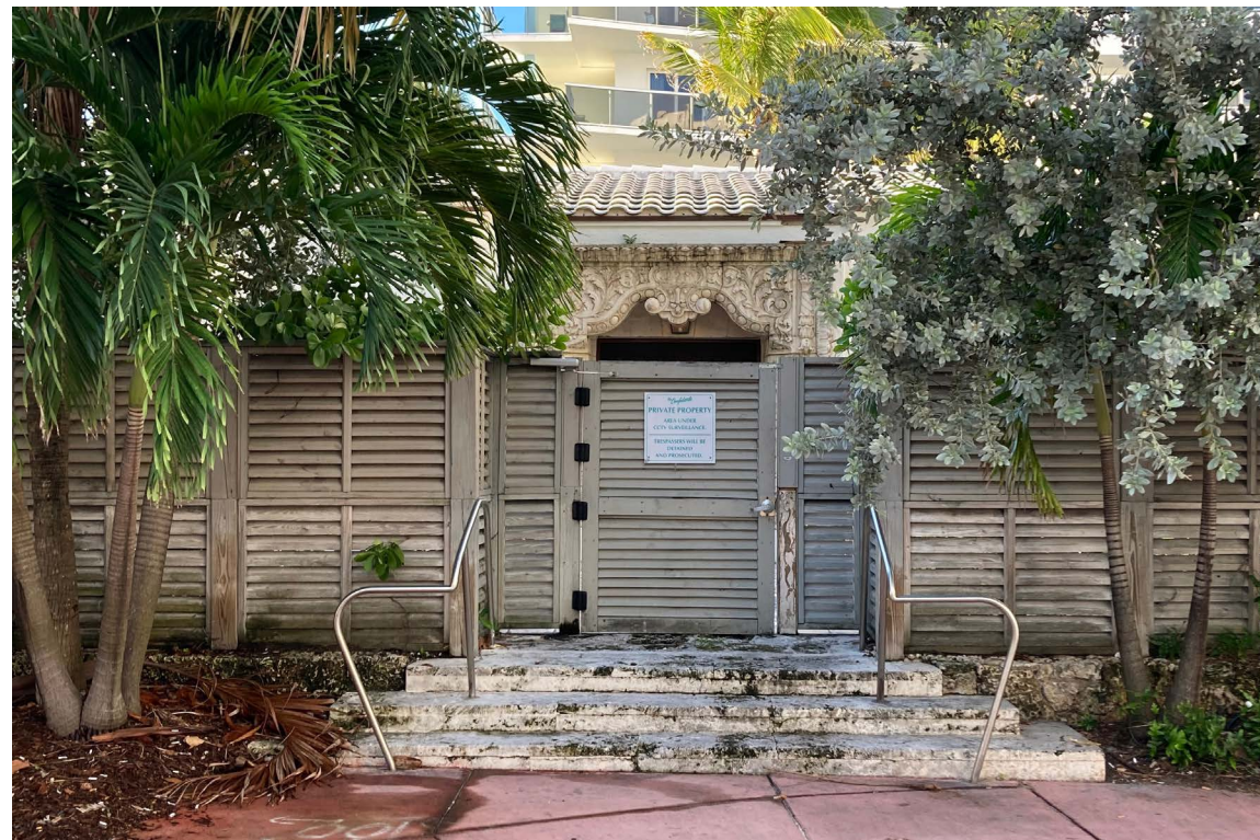
NORTH STREET ACCESS
