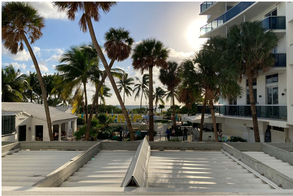
SECOND FLOOR CORRIDOR VIEW
