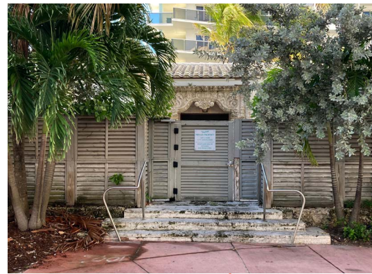
NORTH STREET ACCESS
