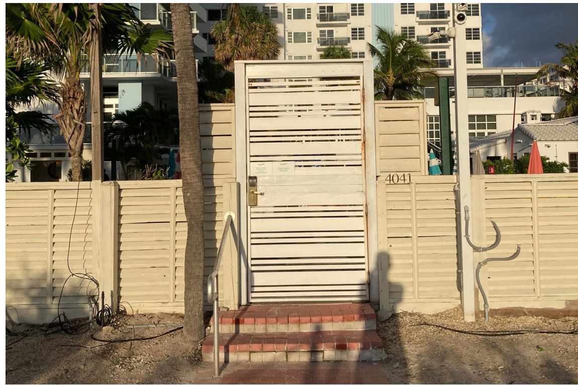
BEACH ACCESS IN EAST FACADE
