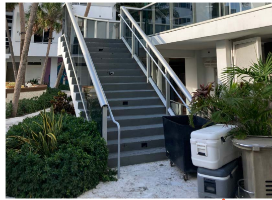
SECOND FLOOR STAIR VIEW
