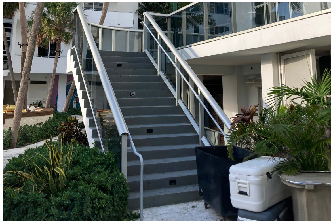
2ND FLOOR ACCESS
