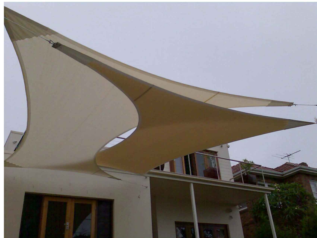
TENSILE CLOTH SHADE STRUCTURE
