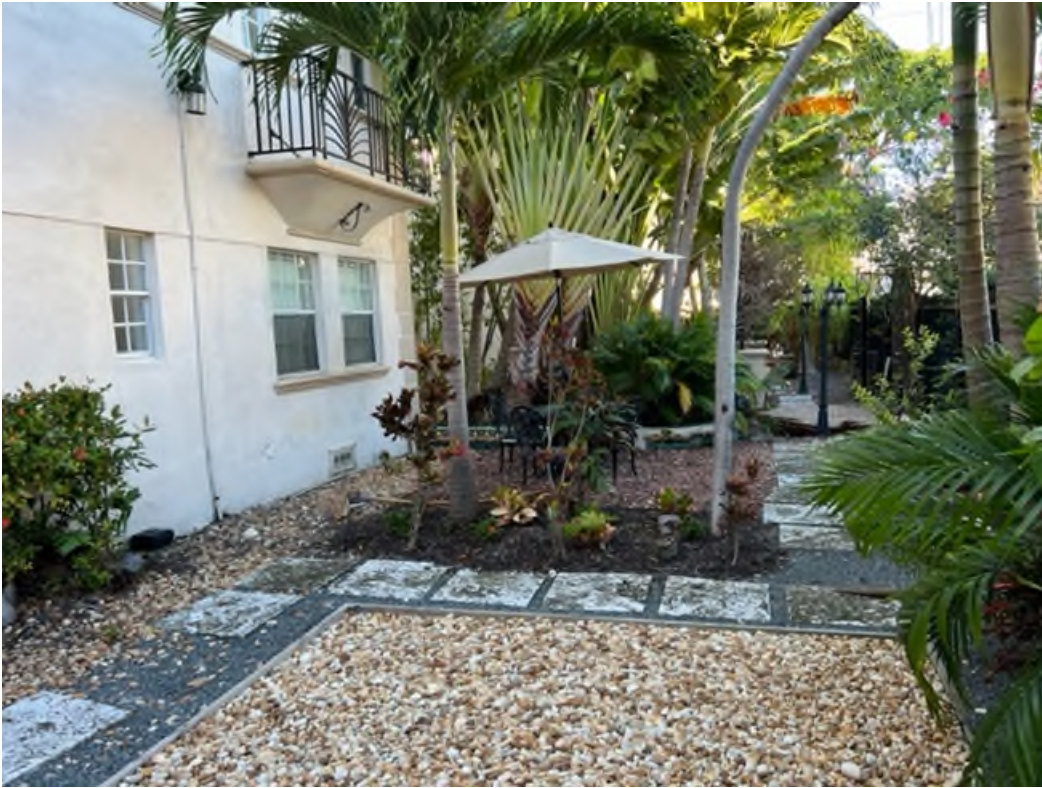
Photos of 1620 Pennsylvania Avenue
