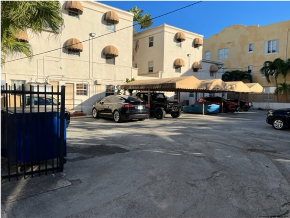
Photos of 1620 Pennsylvania Avenue
