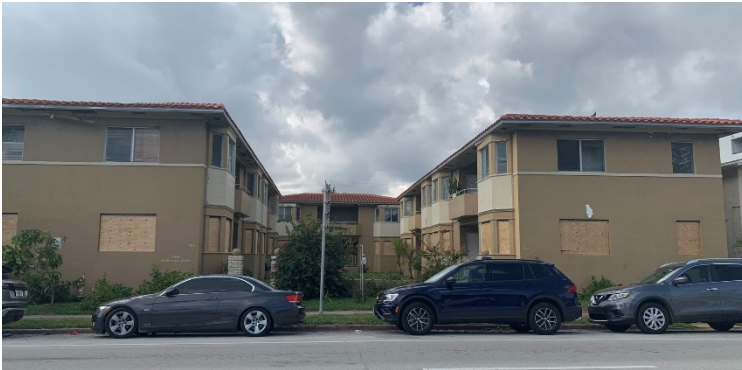
Fig. 24. View of the site looking east from Harding Avenue, January 2022.
