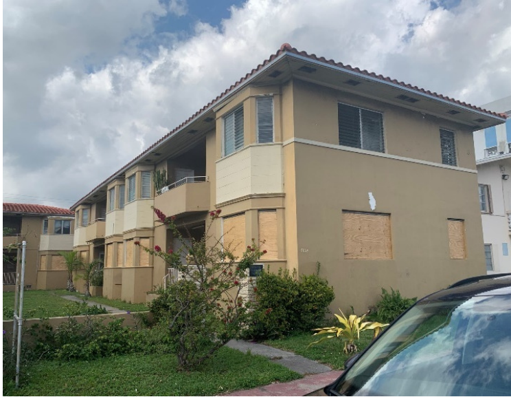
Fig. 26. View of the north building looking east from Harding Avenue, January 2022.
