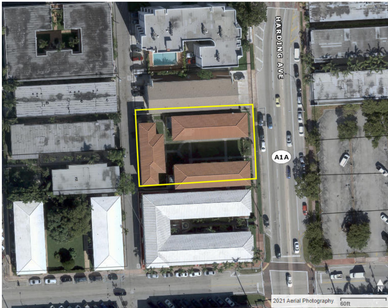
Fig. 9. Aerial showing property at 7418 Harding Ave. Current (Google Maps).
