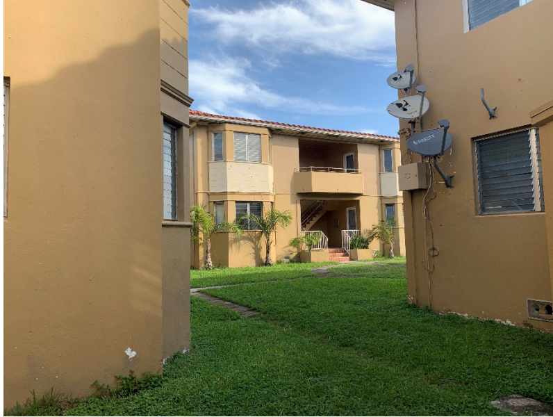
Fig. 30. View of the open area side of the north building, January 2022.
