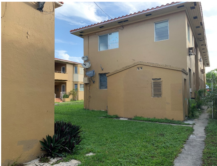
Fig. 28. View of the south building from its rear side, January 2022.
