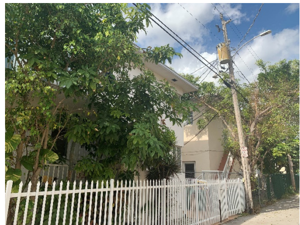
Fig. 21. Building across back alley south of building showed in Fig 10, January 2022.
