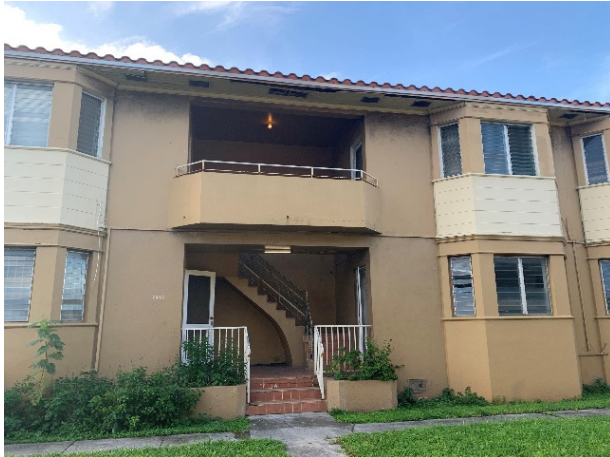
Fig. 31. North façade of south site building, January 2022.
