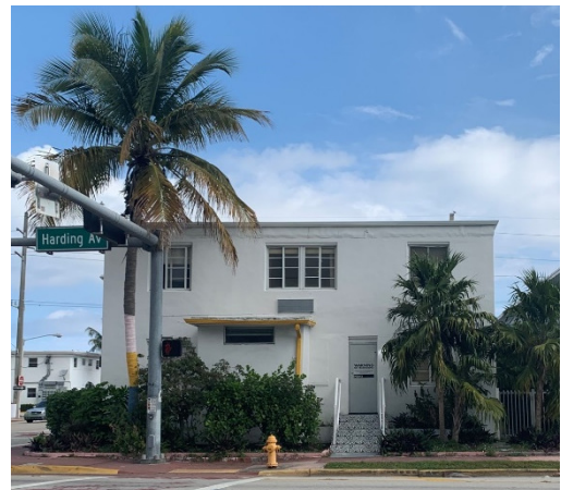
Fig. 17. Building across Harding Avenue, north of building showed in Fig. 16, January 2022
