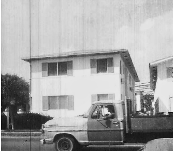
Fig. 5. View of the north building from Harding Ave, January 1963 (Office of the Property Appraiser, Miami-Dade County).
