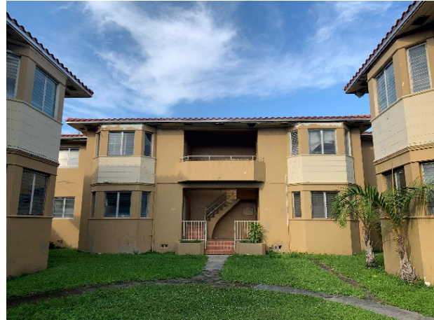
Fig. 32. East façade of West site building, January 2022.
