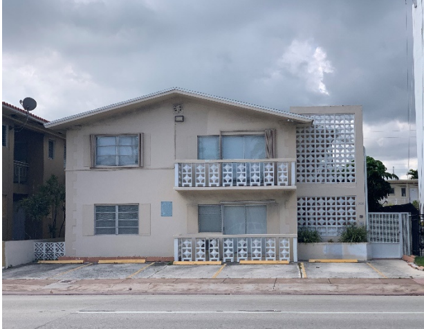
Fig. 10. Building facing Harding Avenue, north of the site, January 2022.
