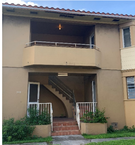
Fig. 34. Detail of outdoor staircases with inset balcony.
