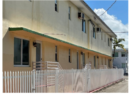
Fig. 19. Building facing back alley, south of the site, January 2022.
