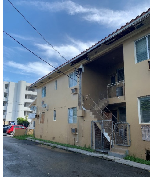
Fig. 27. View of the East building from back alley, January 2022.
