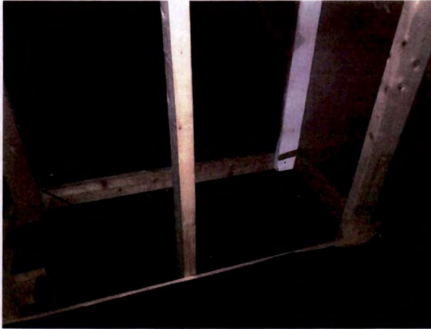
Photograph No. 35 – Wood-framed staircase (East Cinema Theater)
