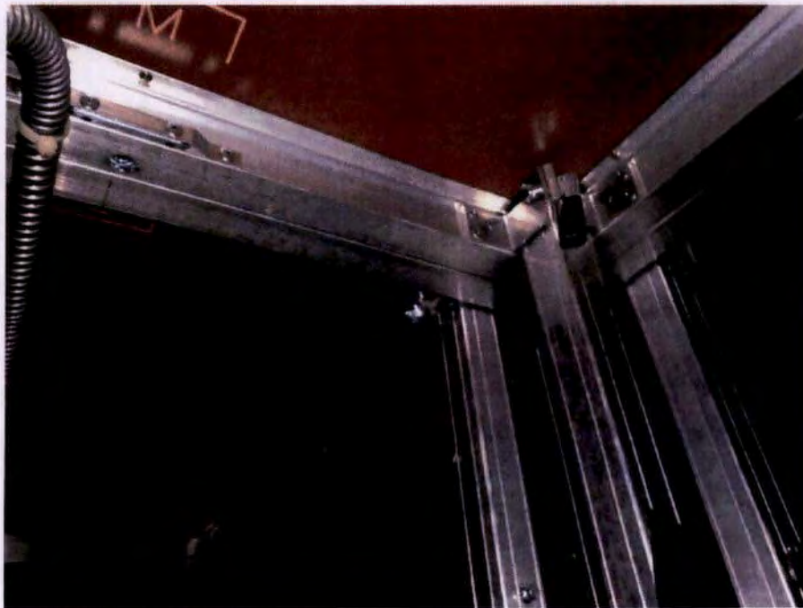
Photograph No. 8 - Aluminum-framed Stage Platform for East Cinema Theater
