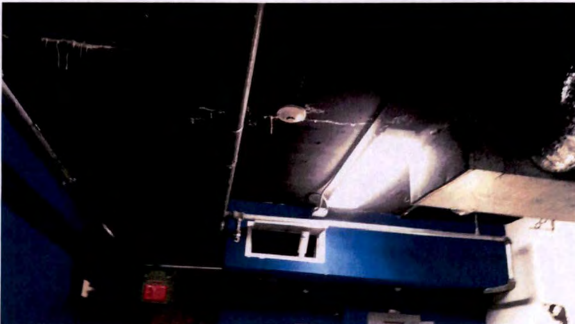
Photograph No. 28 – Efflorescence in Concrete Slab above Projection Room (East Side)
