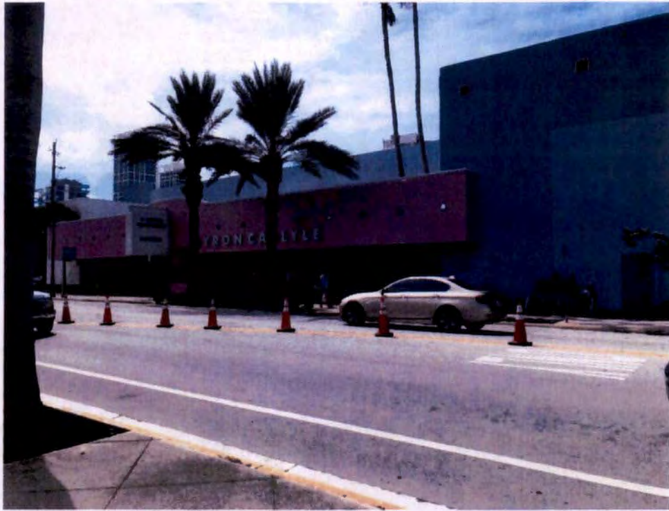
Photograph No. 1 - Overall Photograph of the Building
