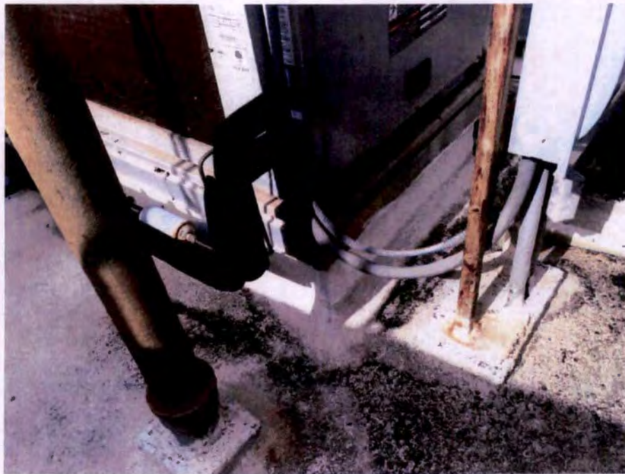
Photograph No. 58 - Lower roof at east side of the building
