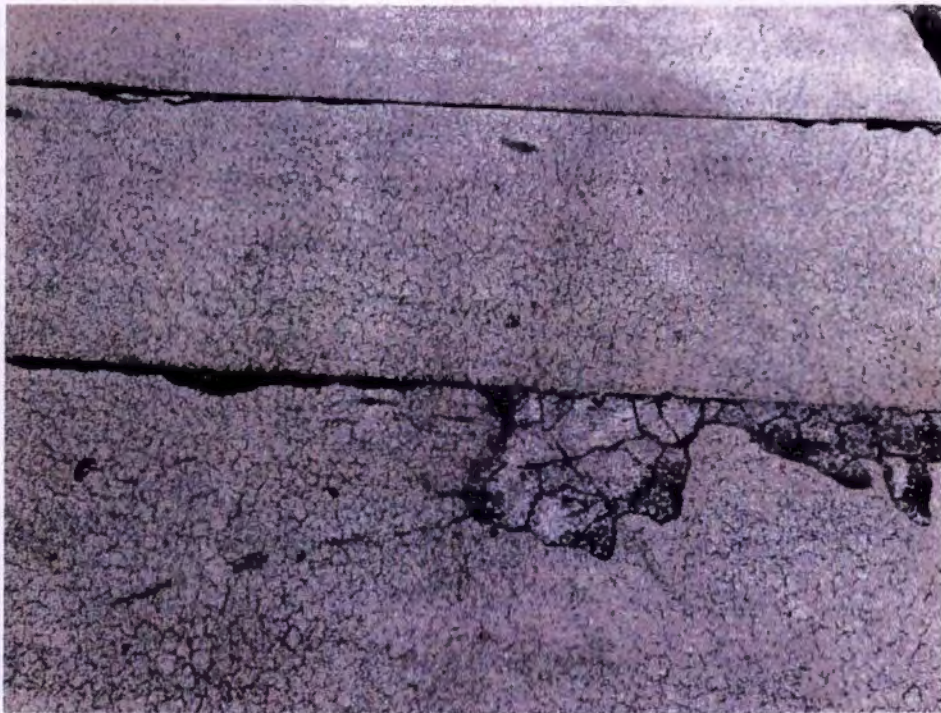
Photograph No. 26 – Deteriorated roofing at Western Upper Roof
