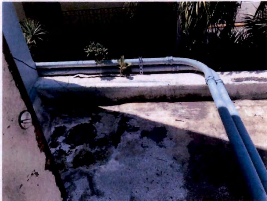
Photograph No. 70 – Low roof at the second floor
