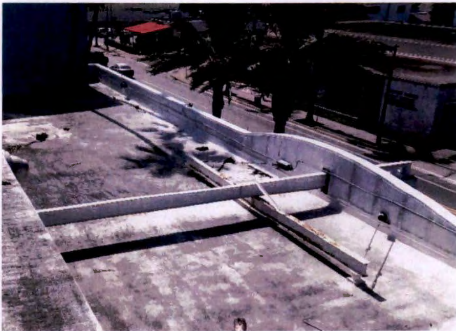
Photograph No. 10 – Structural Steel supporting Theater Sign at North Façade
