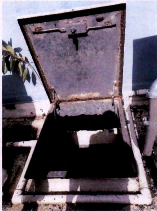
Photograph No. 29 – Roof Access Hatch (Lower Roof at East Side)
