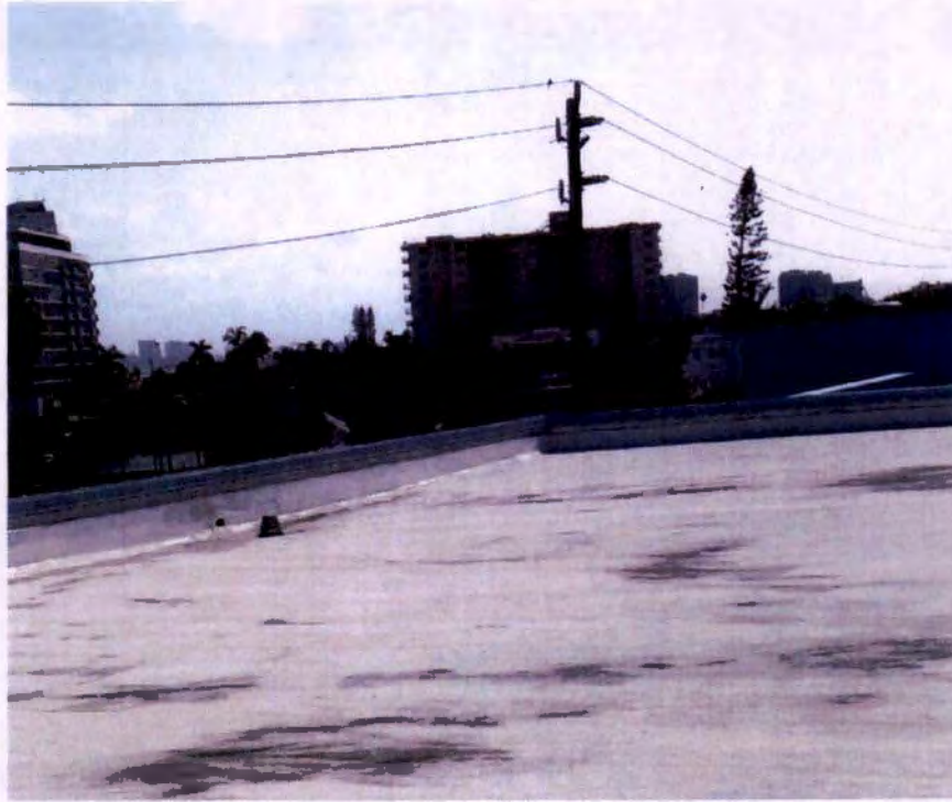
Photograph No. 67 – Eastside upper roof
