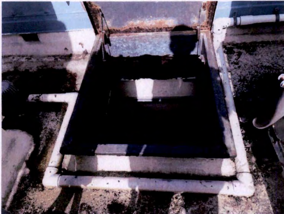
Photograph No. 68 – Low roof at east side of building
