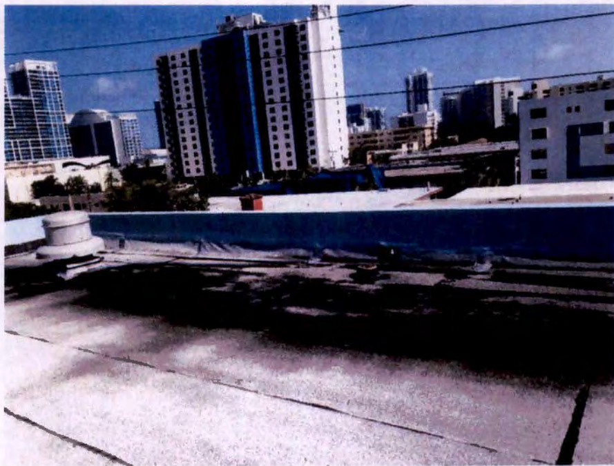
Photograph No. 66 – Westside upper roof
