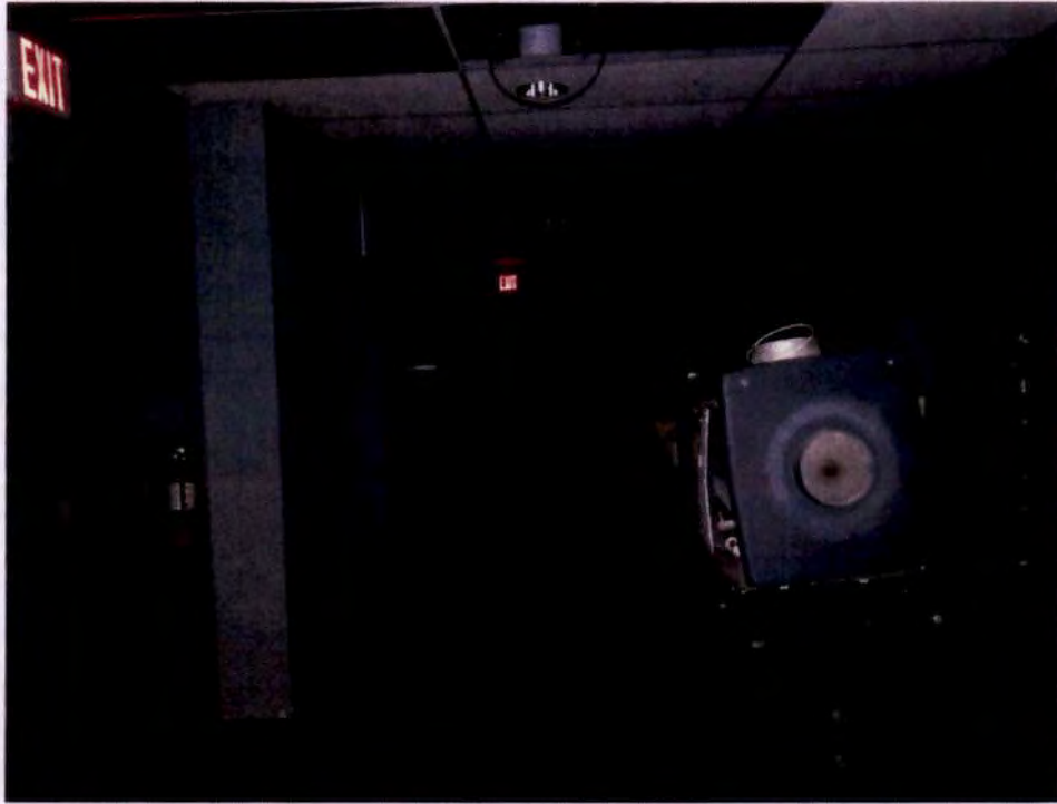
Photograph No. 3 - Projection Room for West Cinema Theaters
