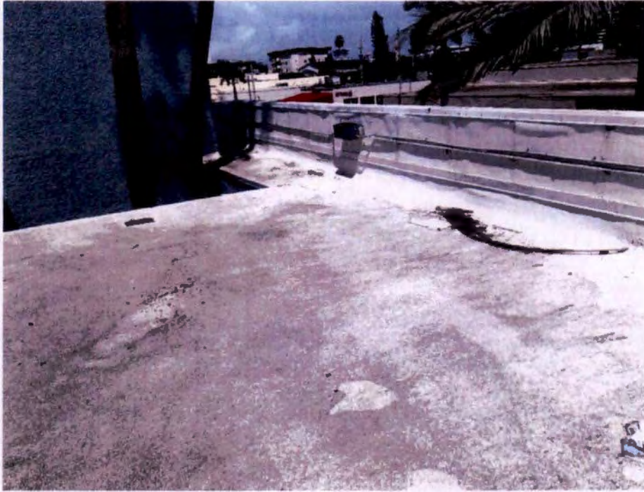
Photograph No. 73 – Low roof at the second floor (north)
