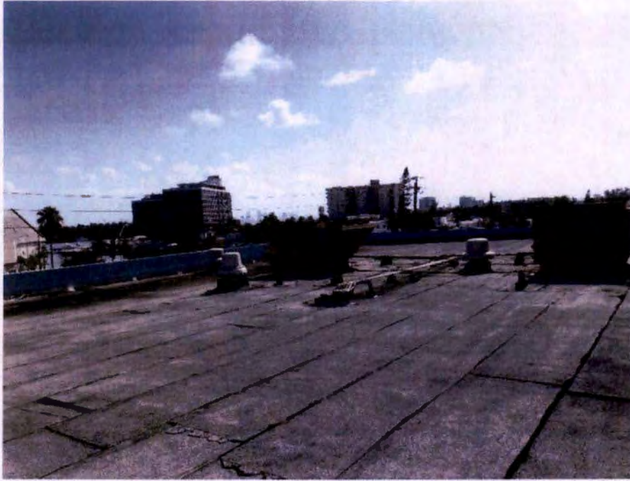
Photograph No. 43– Upper Roof of West Cinema Theater
