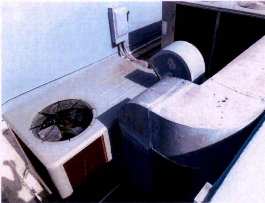
Photograph No. 53 – Low Roof at East Side of Building
