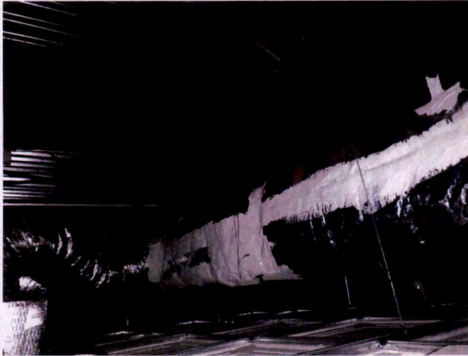
Photograph No. 49 – Underside of Low Roof at Second Level in North Portion of Building
