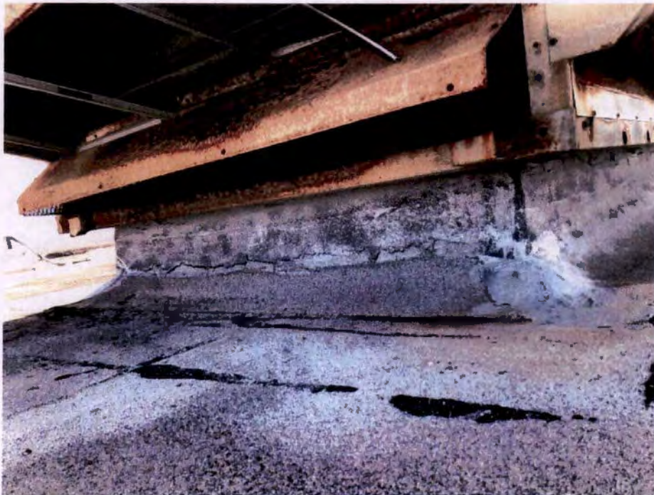
Photograph No. 22 - Rooftop Package Unit at Western Upper Roof
