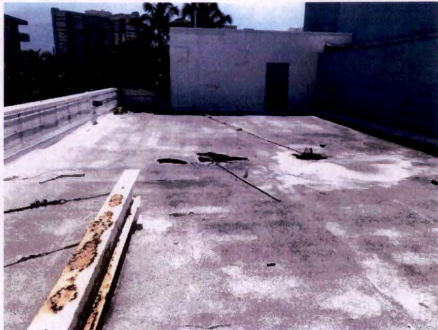
Photograph No. 72 – Low roof at the second floor (north)
