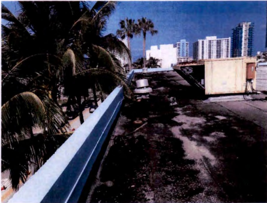
Photograph No. 57 - Upper roof at west side of the building
