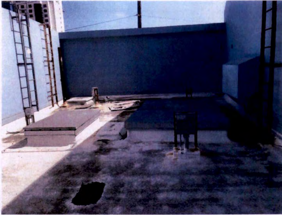
Photograph No. 61 – Covered Opening at Low Roof between East and West
