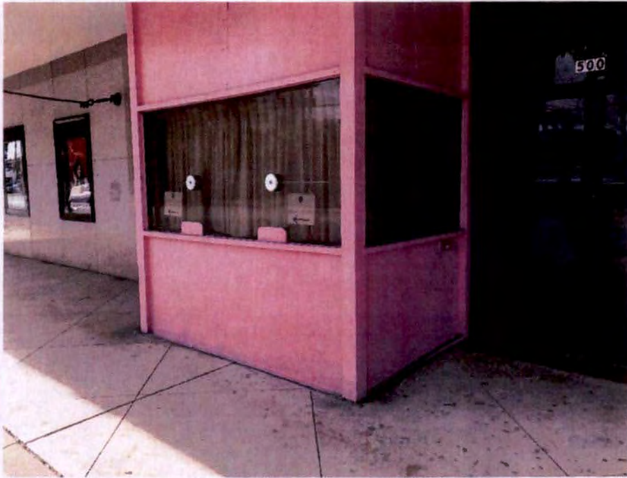
Photograph No. 85 – Ticket Box Office at North Façade
