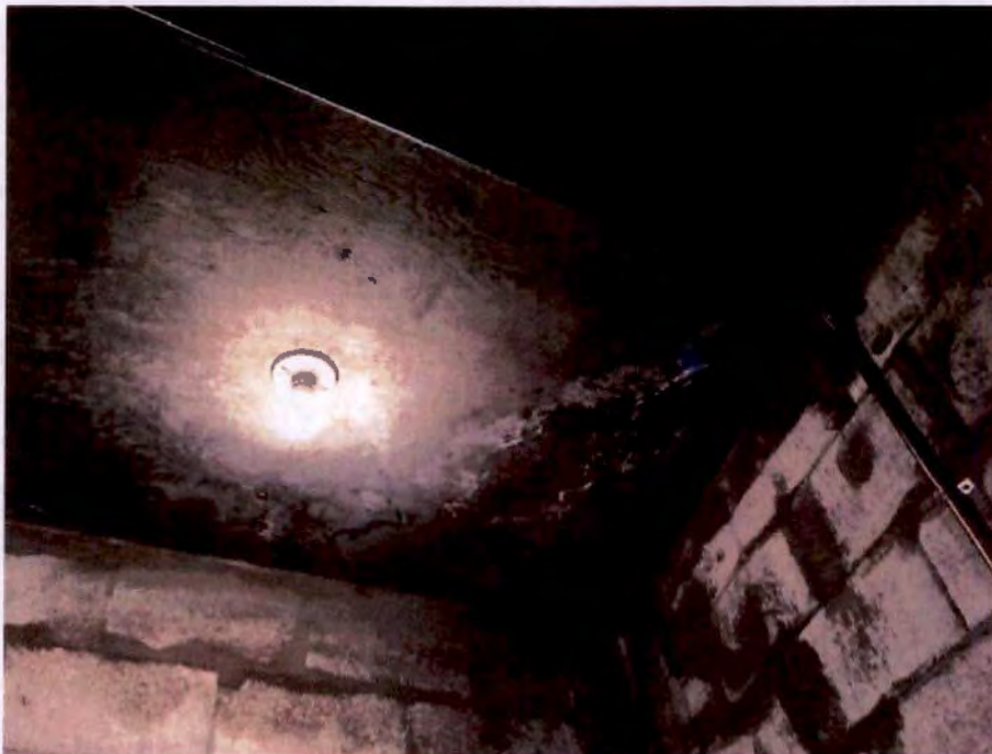
Photograph No. 56 – Underside of Low Roof at East Side of Building
