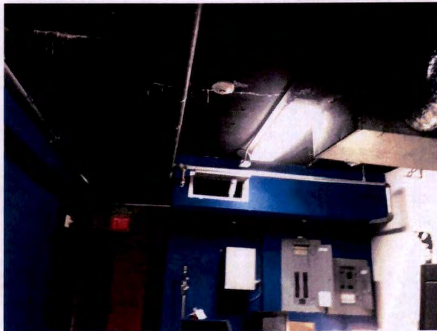
Photograph No. 54 – Underside of Low Roof at East Side of Building
