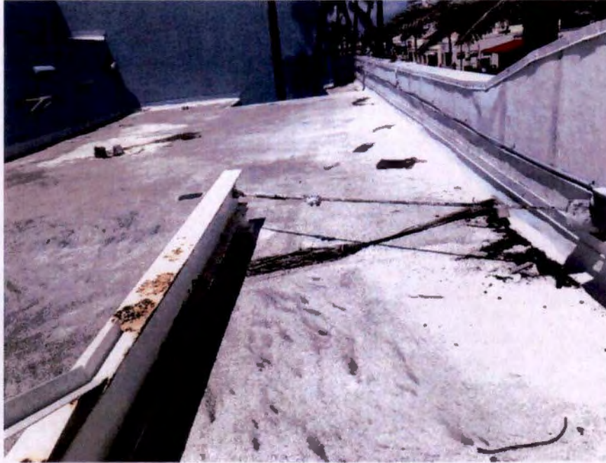
Photograph No. 71 – Low roof at the second floor (north)
