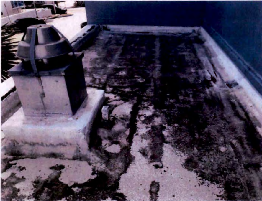
Photograph No. 55 – Low Roof at East Side of Building
