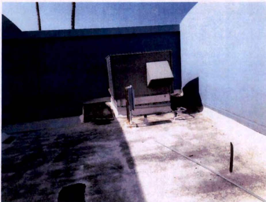
Photograph No. 60 – Covered Opening at Low Roof between East and West
