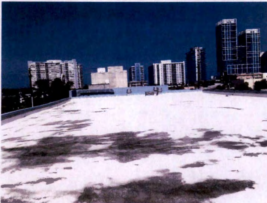
Photograph No. 42– Upper Roof of East Cinema Theater
