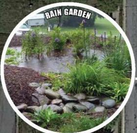
Meandering rain garden / ephemeral stream channel planted with pollinators to collect runoff from drive via curb cut and flume
