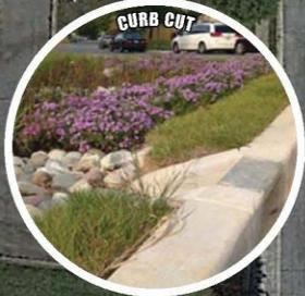
Curb cuts divert parking lot runoff to infiltration trench to increase soil moisture for new tree plantings.
