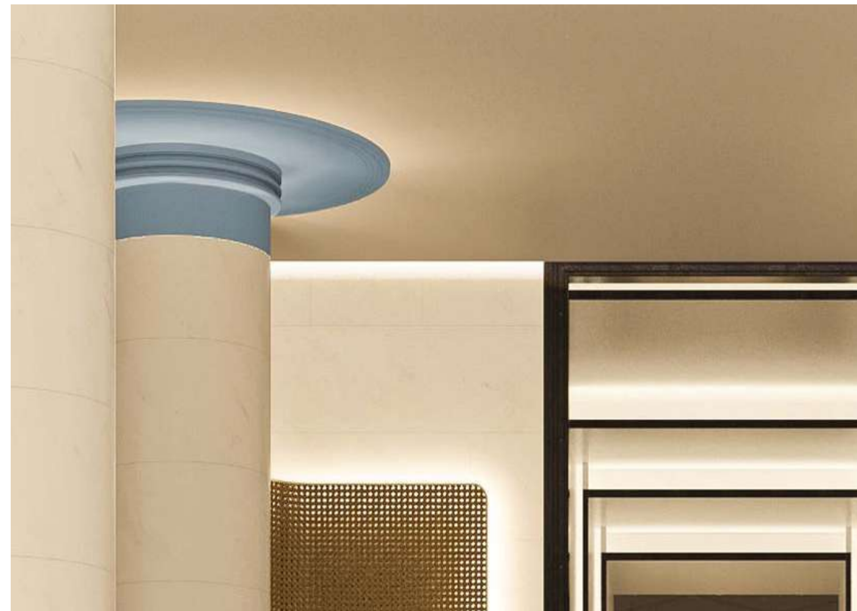
Cove lighting at perimeter interior walls
