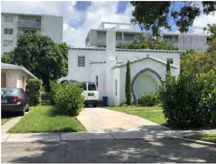
Building A 2 Story
