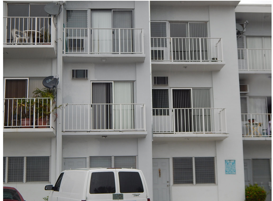
New PTAC units at Unit 215 BREV160069
