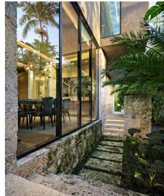
STONE TILE CLADDING
