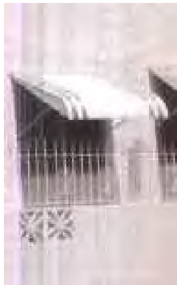
Aluminum fold down awnings installed in 1974 for privacy and solar protection
