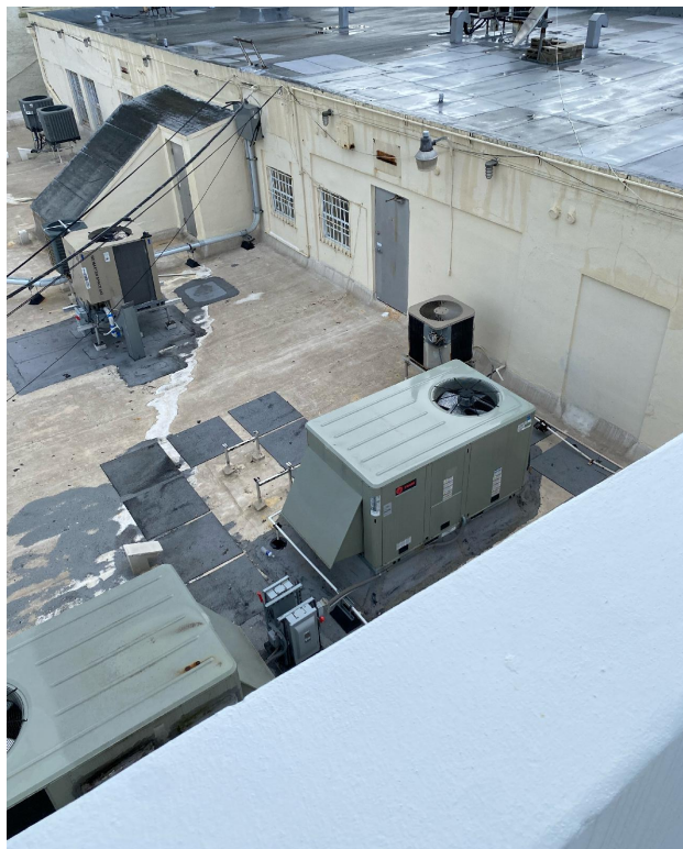
3 818 LINCOLN RD. BUILDING 3RD FLOOR LEVEL TERRACE
