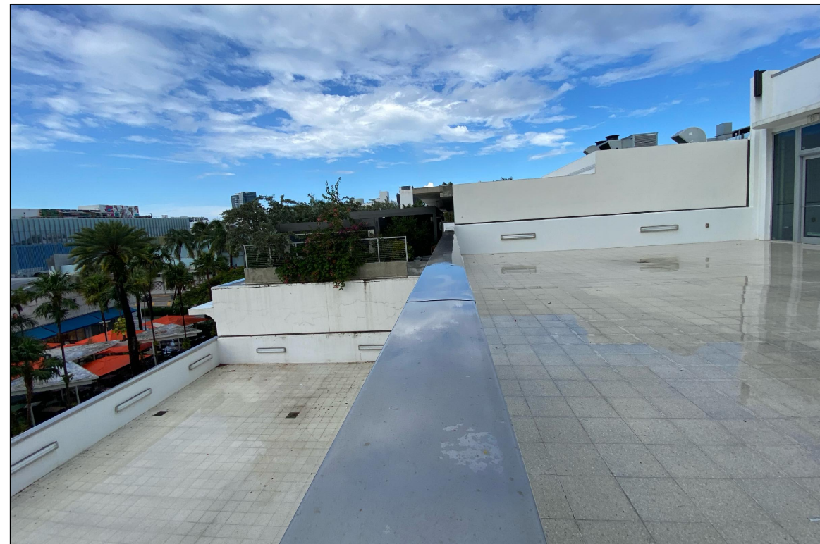
5 818 LINCOLN RD. BUILDING 3RD FLOOR LEVEL TERRACE
