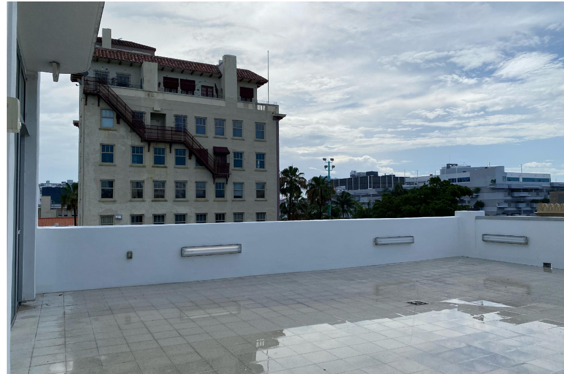
2 818 LINCOLN RD. BUILDING 3RD FLOOR LEVEL TERRACE
