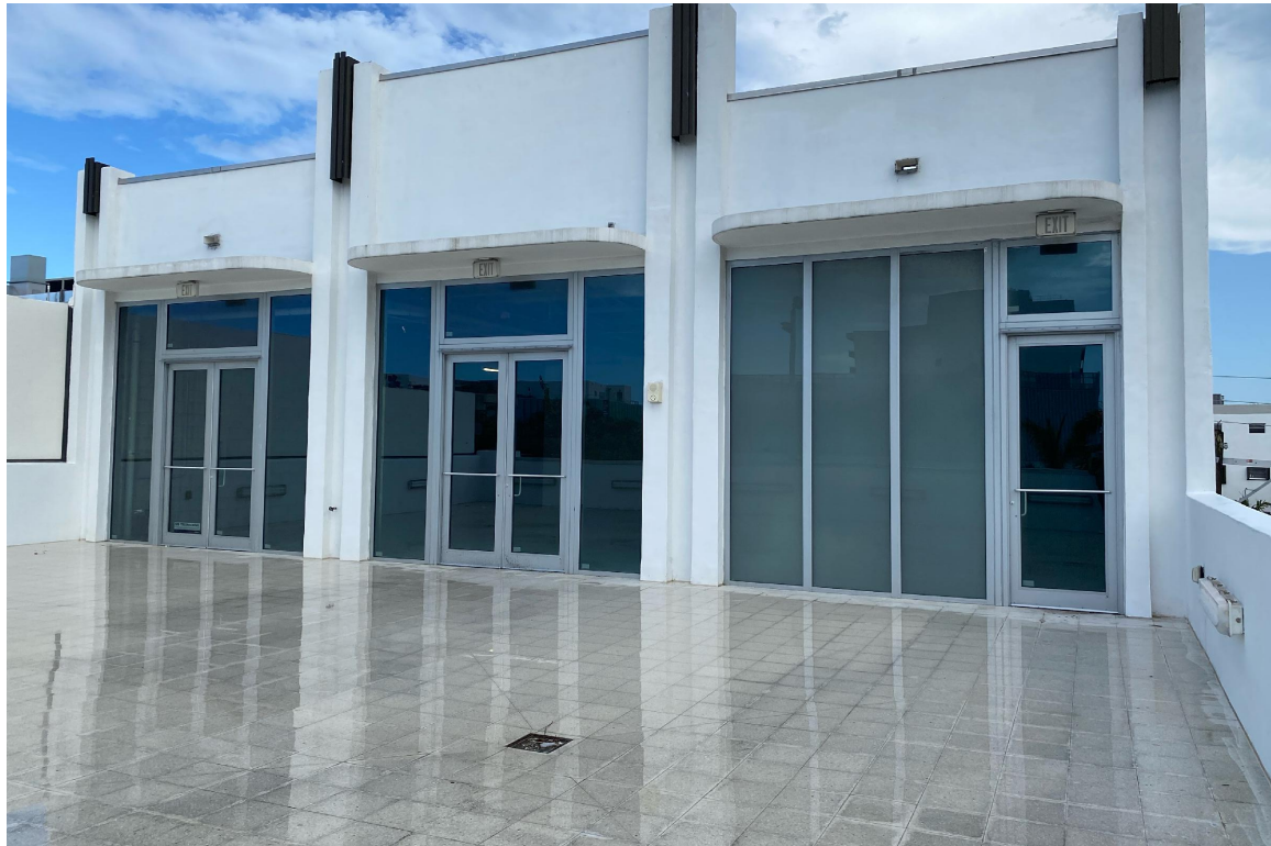
1 818 LINCOLN RD. BUILDING 3RD FLOOR LEVEL TERRACE
