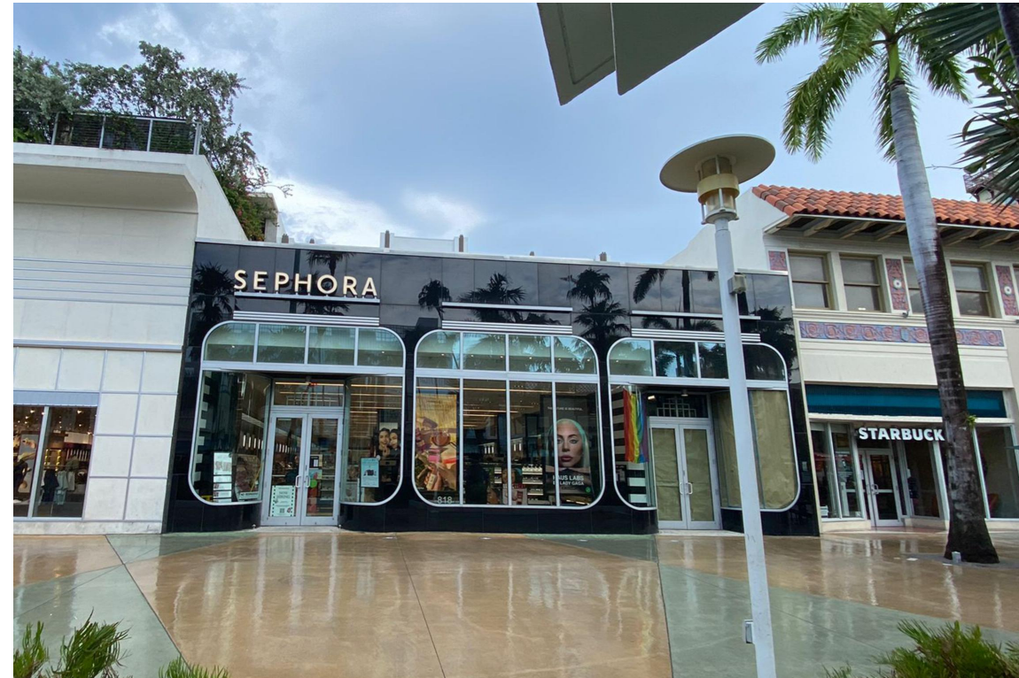
2 818 LINCOLN RD. BUILDING NORTH FACADE
