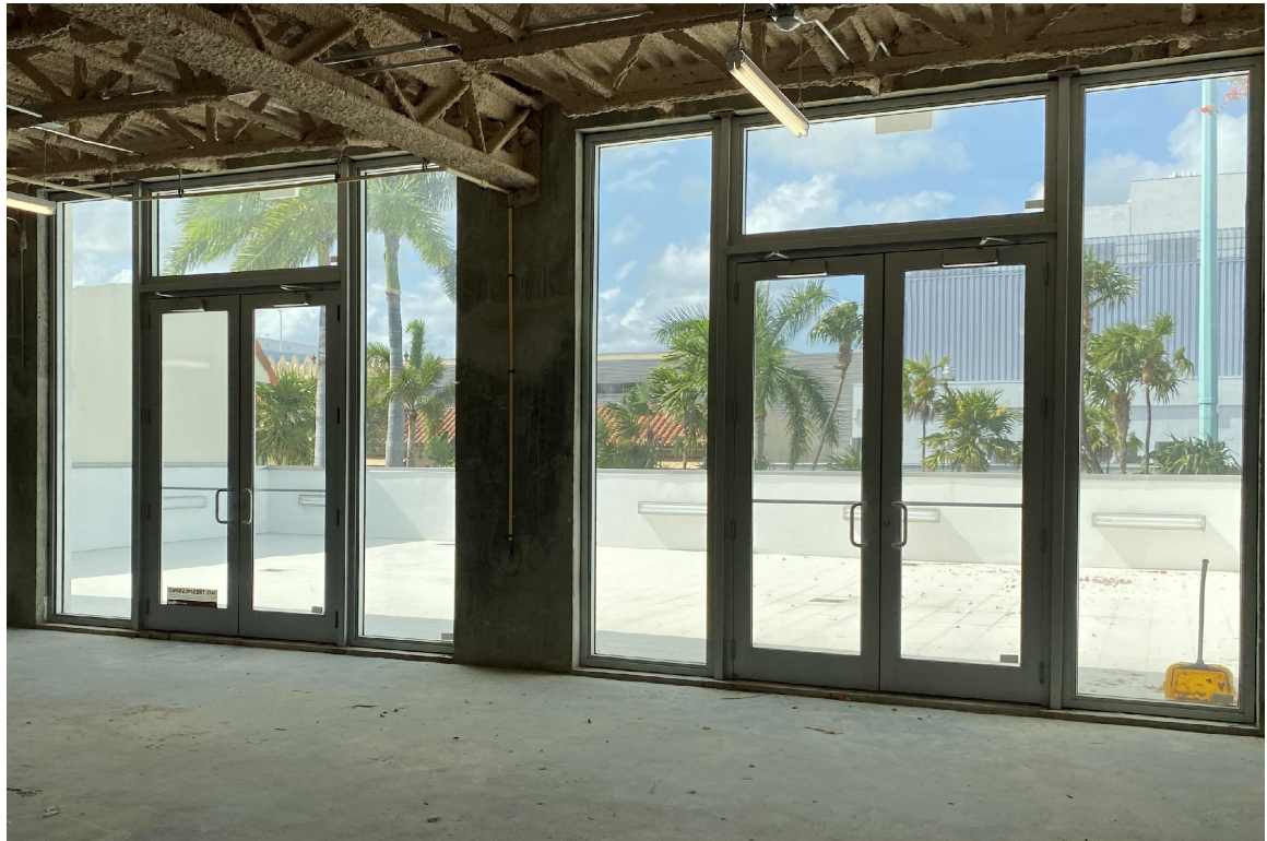
1 818 LINCOLN RD. BUILDING 2ND FLOOR LEVEL TERRACE
