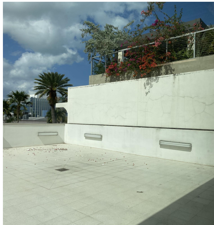
5 818 LINCOLN RD. BUILDING 2ND FLOOR LEVEL TERRACE
