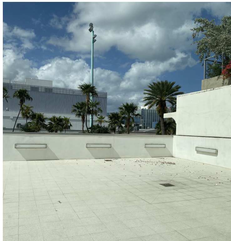
4 818 LINCOLN RD. BUILDING 2ND FLOOR LEVEL TERRACE
