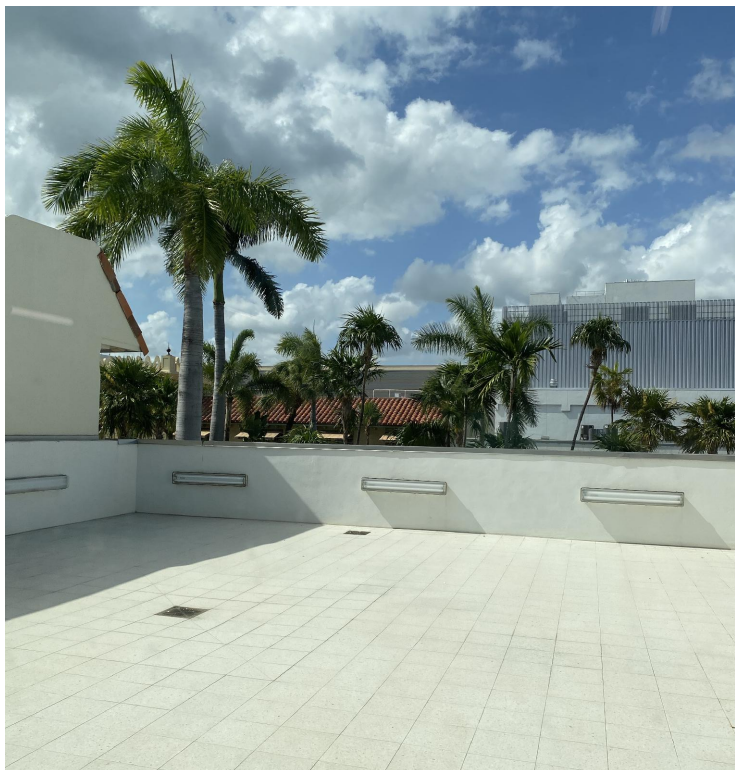
3 818 LINCOLN RD. BUILDING 2ND FLOOR LEVEL TERRACE
