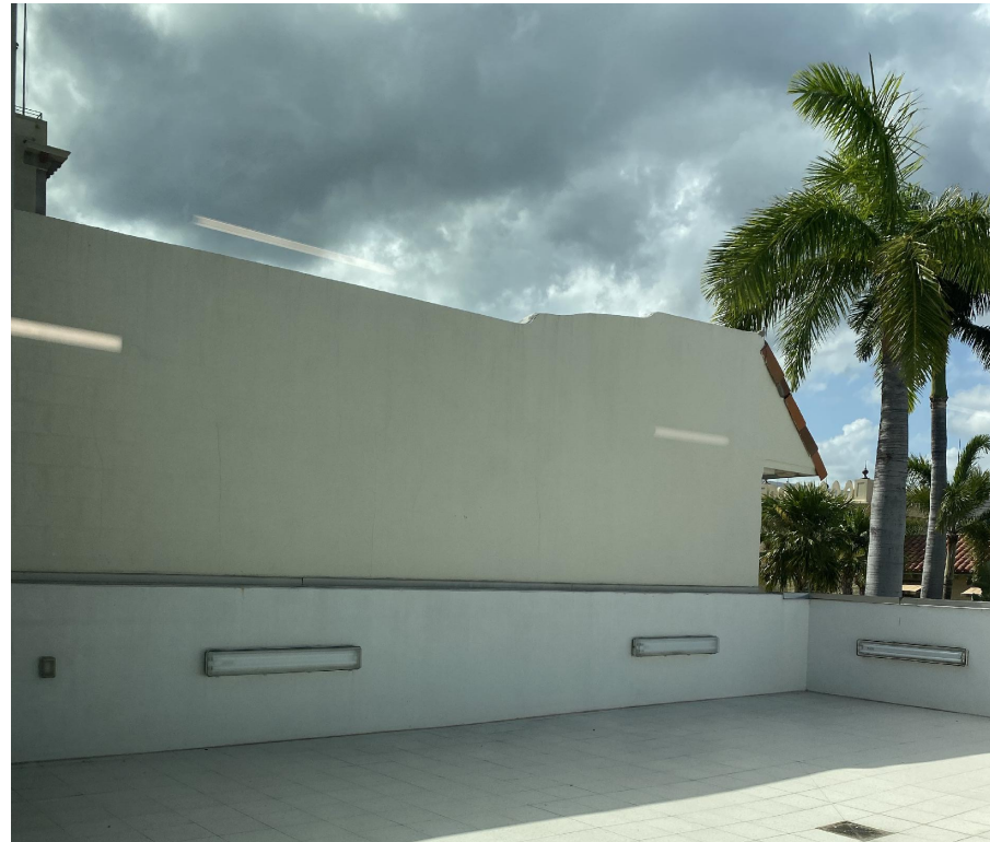
2 818 LINCOLN RD. BUILDING 2ND FLOOR LEVEL TERRACE
