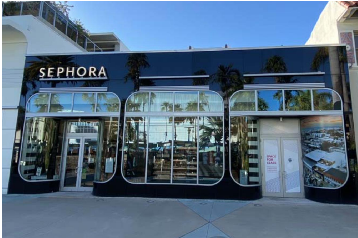
1 818 LINCOLN RD. BUILDING NORTH FACADE
