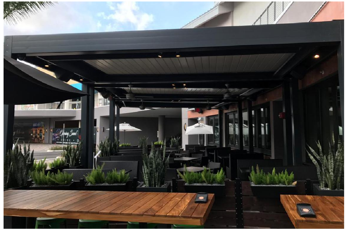
2 RETRACTABLE LOUVERED SYSTEM INSTALLED IN DORAL CITY PLACE
