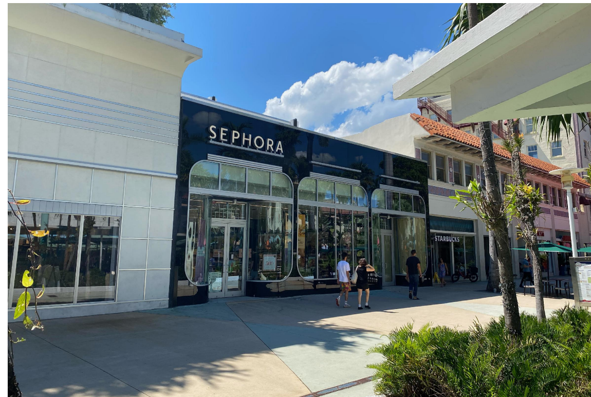
4 818 LINCOLN RD. BUILDING NORTH FACADE
