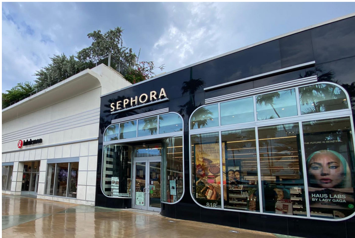
3 818 LINCOLN RD. BUILDING NORTH FACADE
