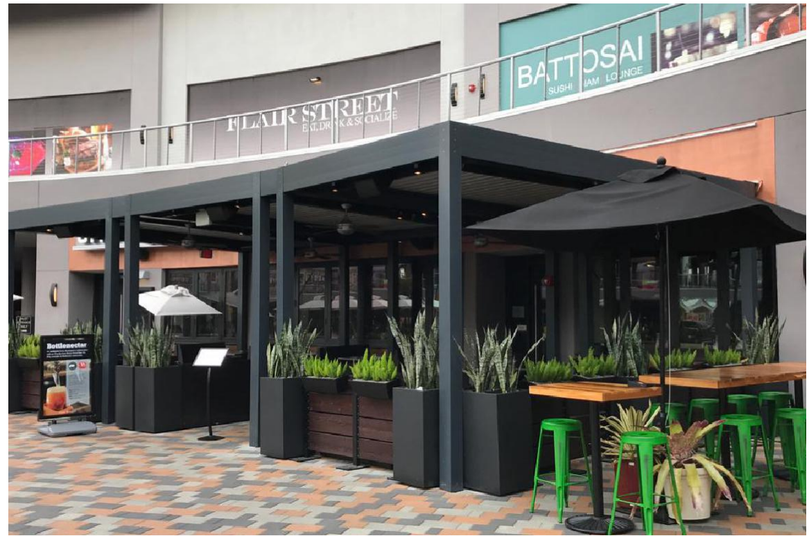
1 RETRACTABLE LOUVERED SYSTEM INSTALLED IN DORAL CITY PLACE
