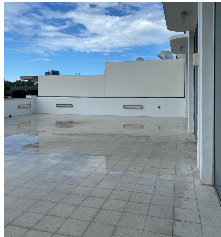
4 818 LINCOLN RD. BUILDING 3RD FLOOR LEVEL TERRACE
