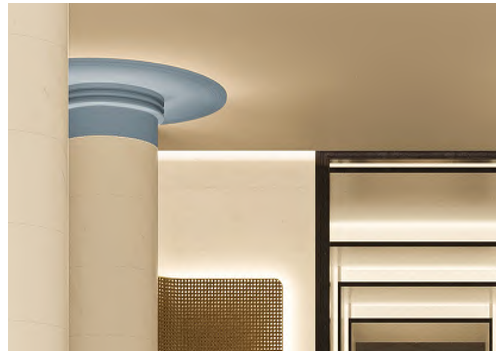
Cove lighting at perimeter interior walls
