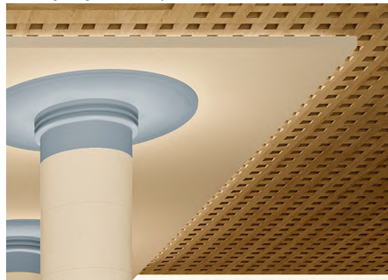
Cove lighting at drop ceiling
