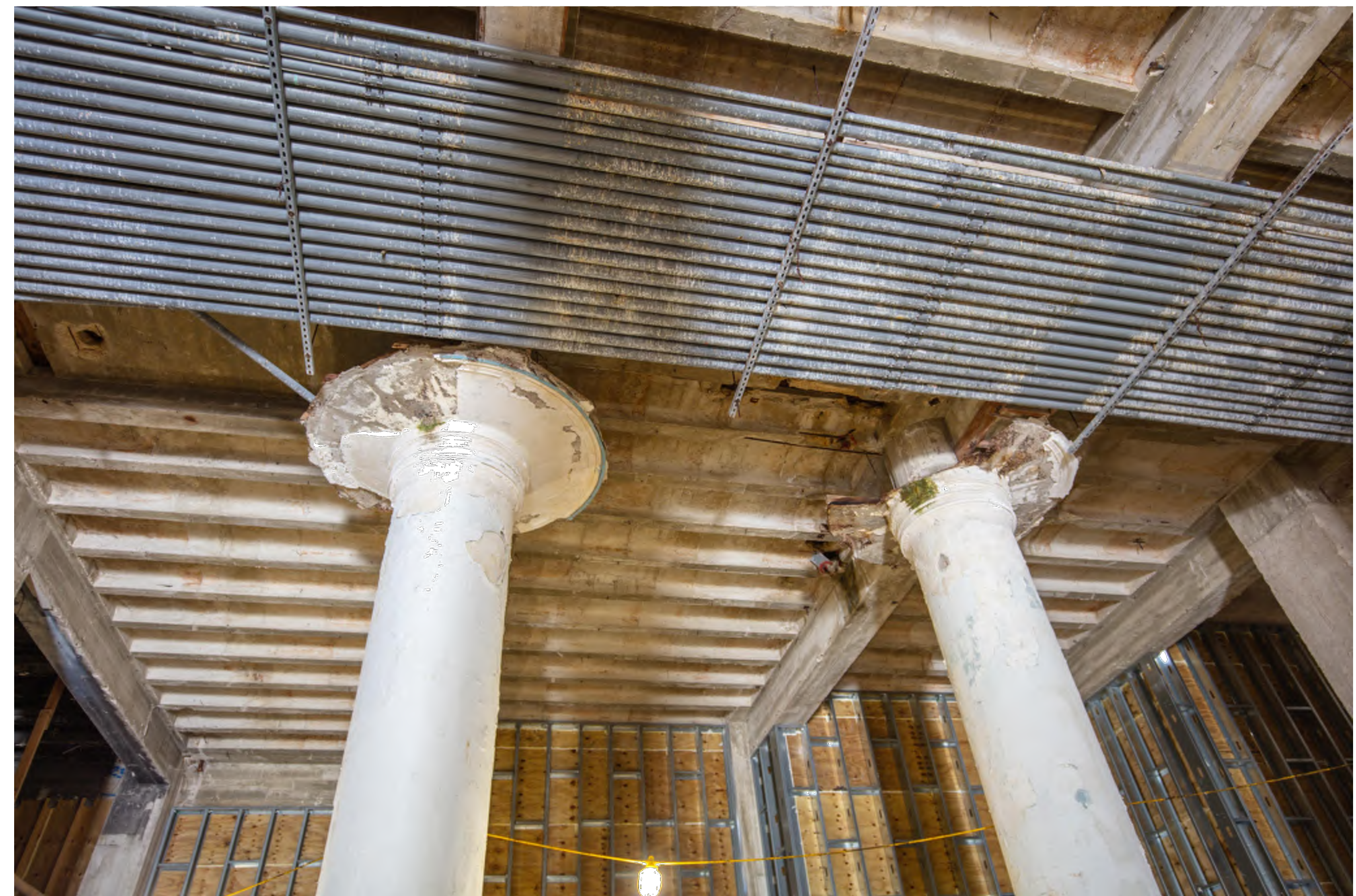
INTERIOR - EXISTING CONDITIONS
