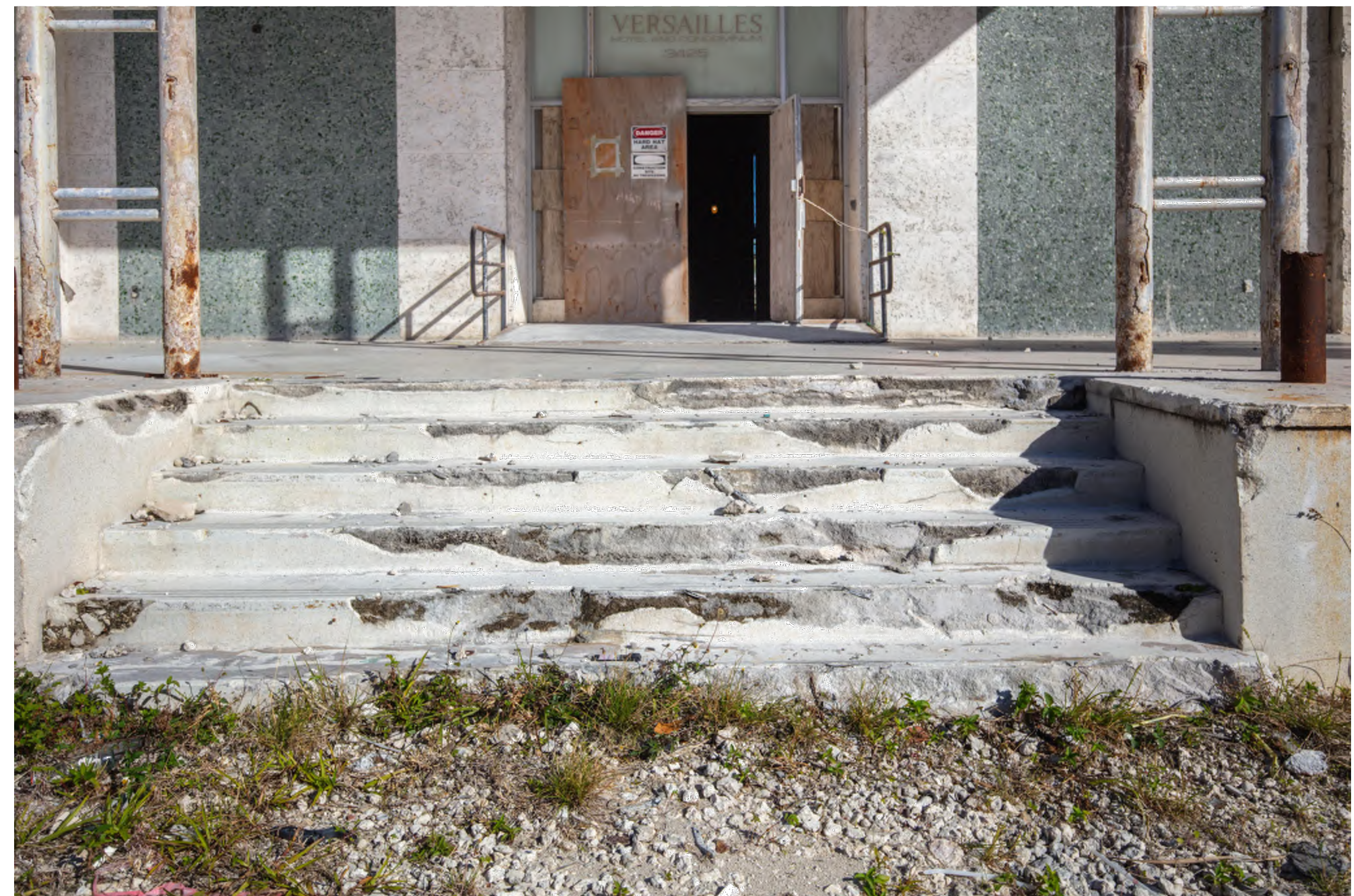
EXTERIOR - EXISTING CONDITIONS
