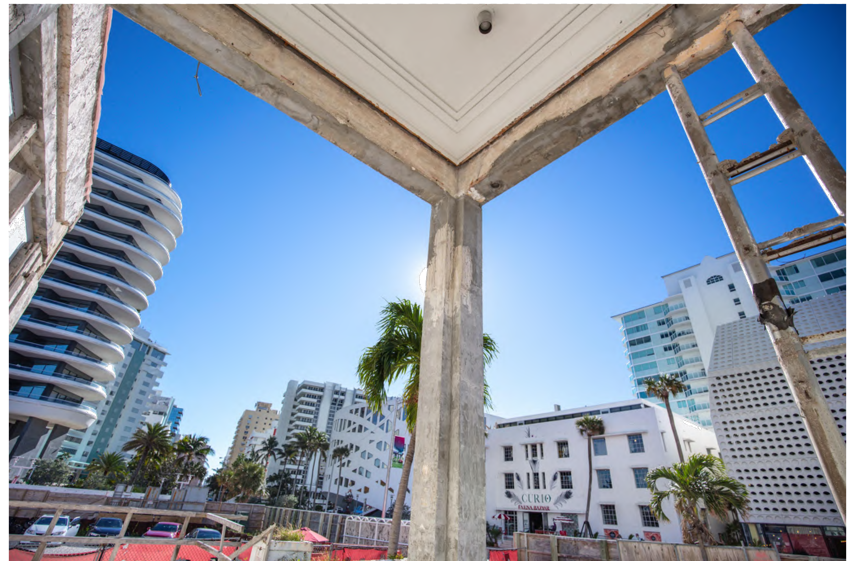
EXTERIOR - EXISTING CONDITIONS
