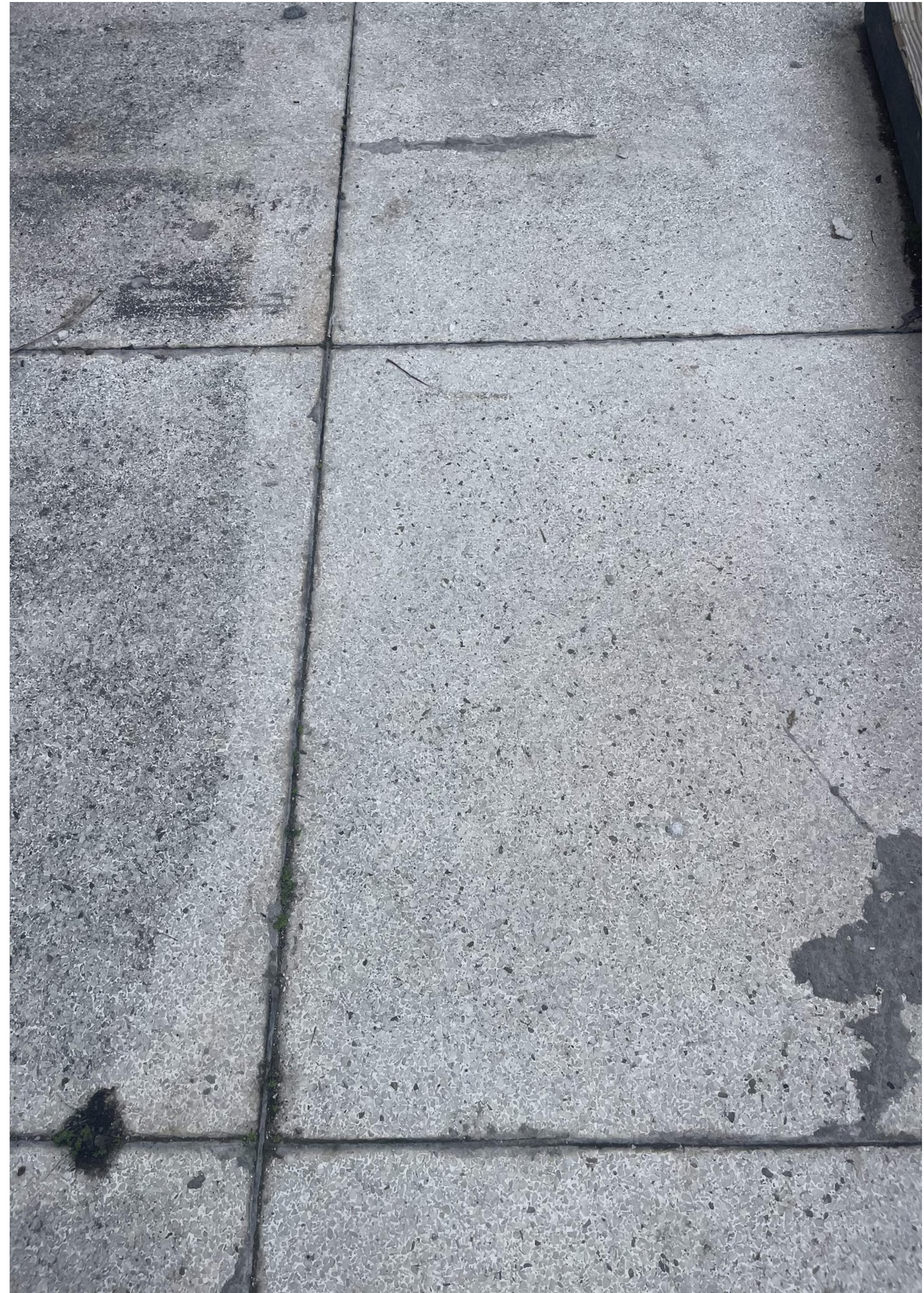
PORCHE - EXISTING CONDITIONS
