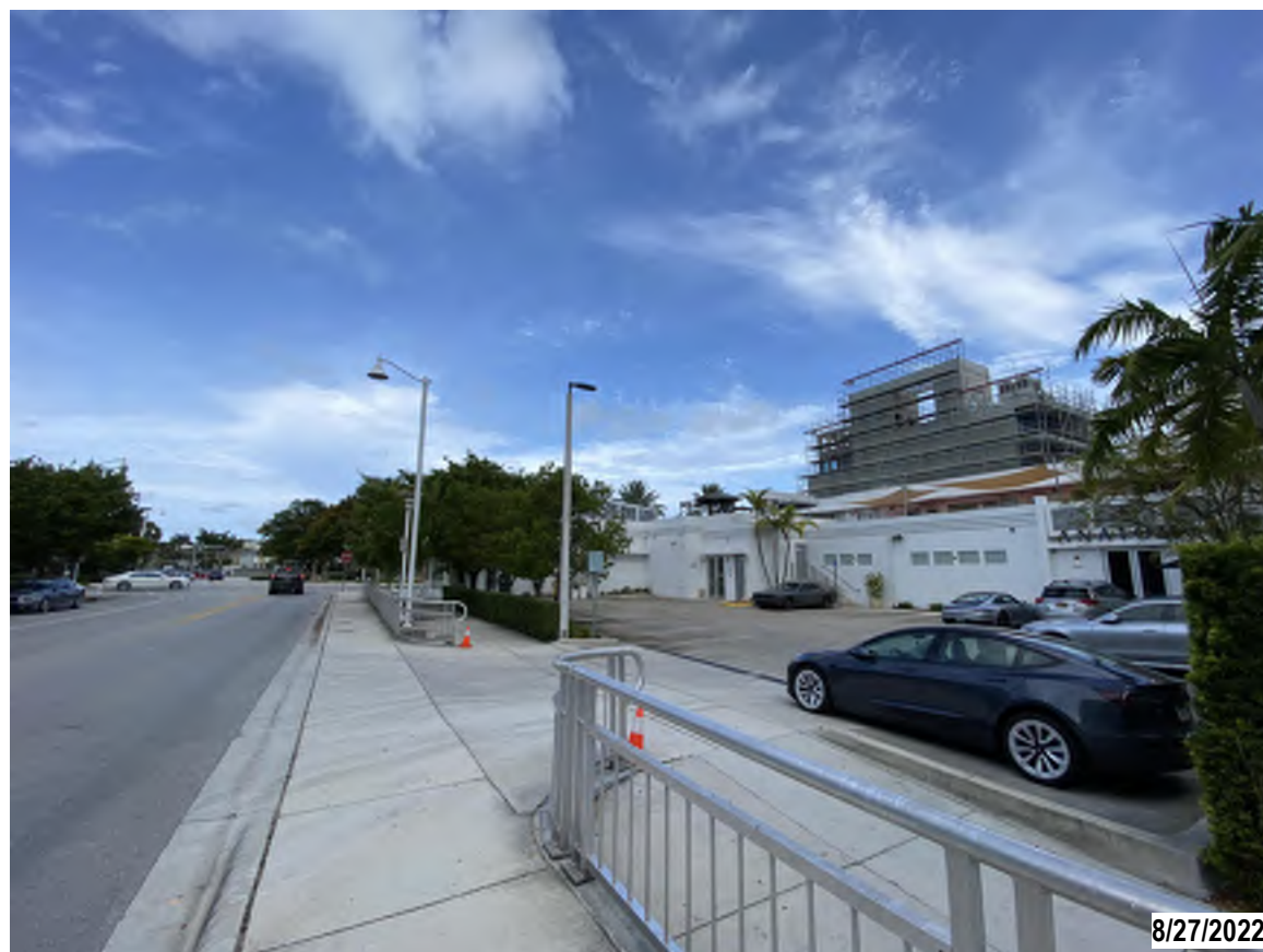
3. VIEW OF SITE FROM WEST AVENUE
