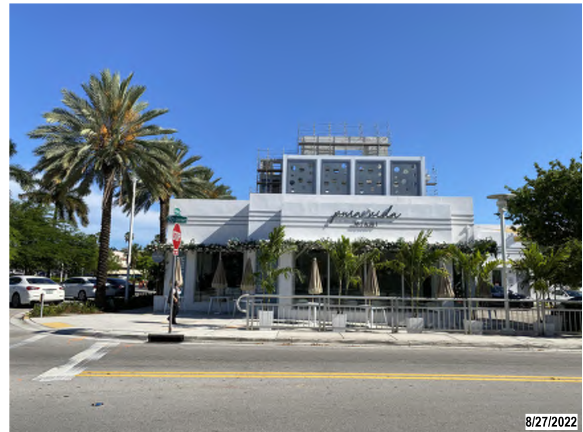
2. VIEW OF EXISTING STRUCTURES FROM 20TH STREET
