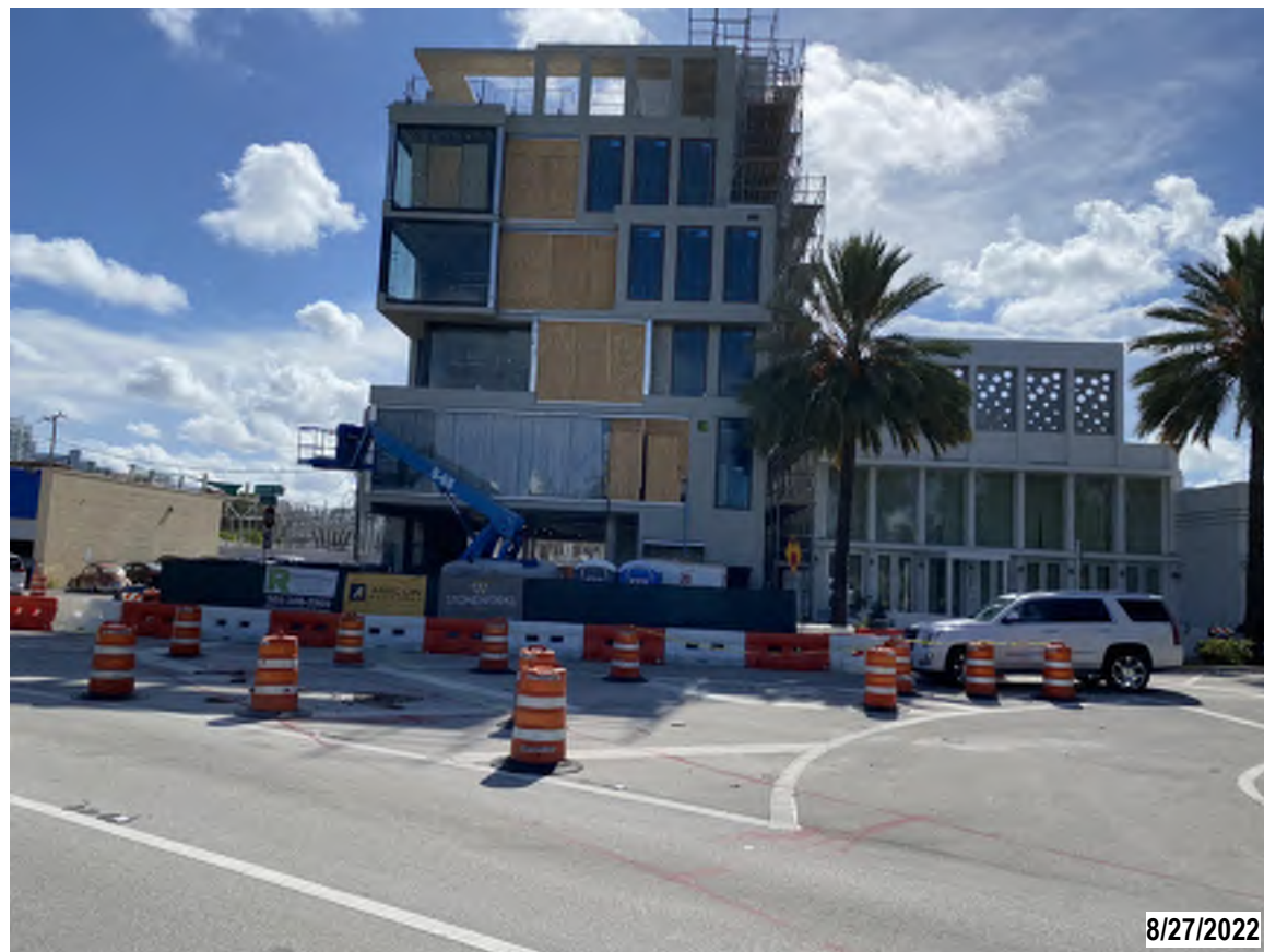
1. VIEW OF EXISTING STRUCTURES FROM ALTON ROAD
