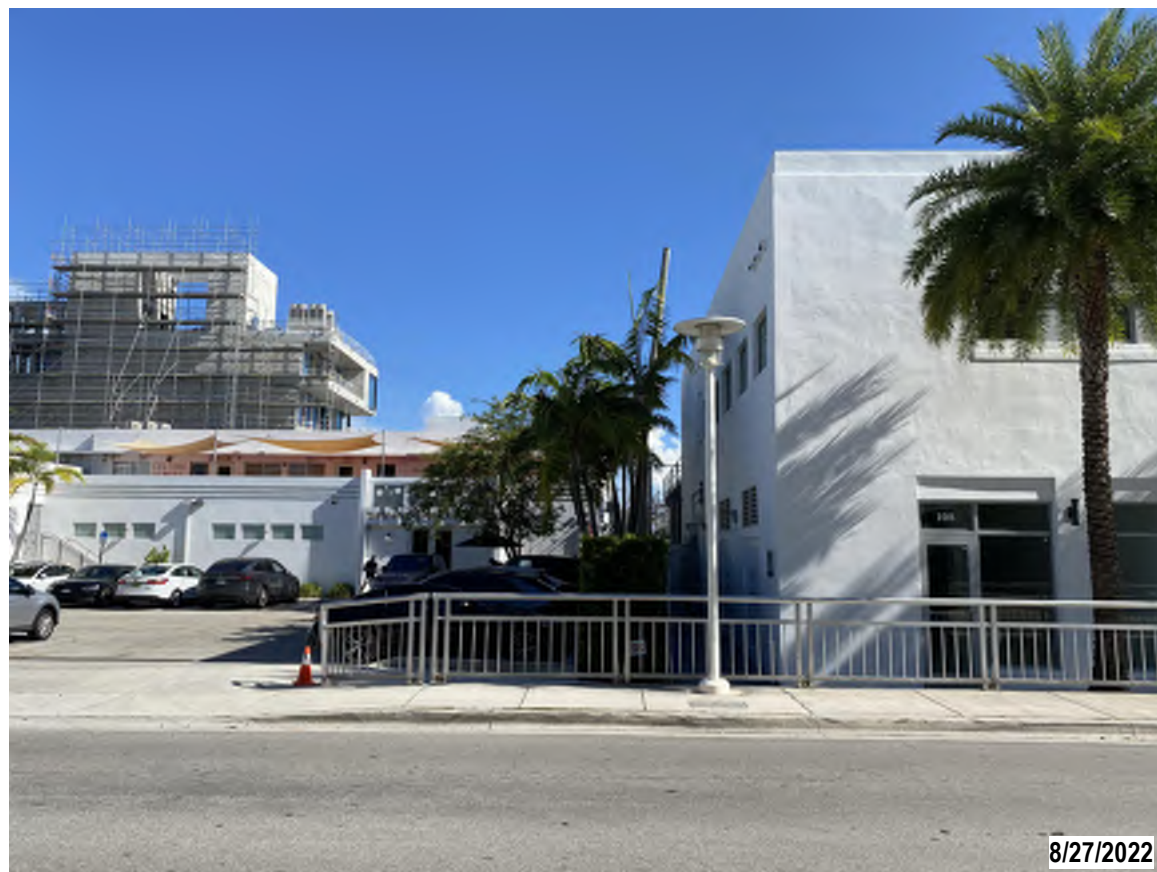
3. VIEW OF EXISTING STRUCTURES FROM WEST AVENUE
