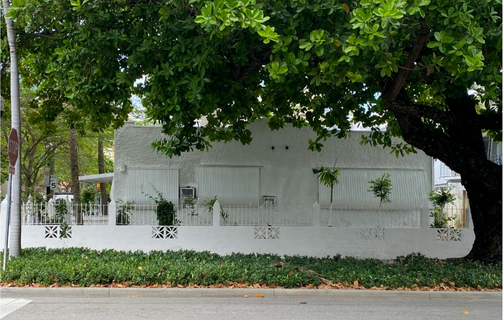
TOP PHOTO: VIEW OF SIDE (EAST) ELEVATION FROM MERIDIAN AVENUE
