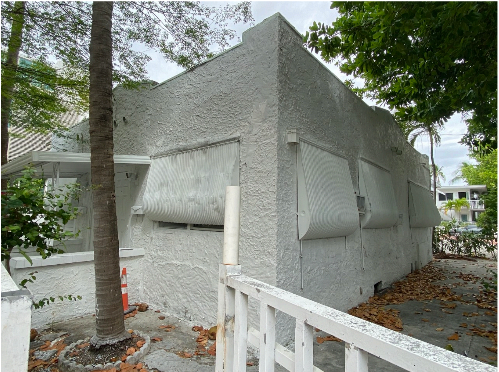
ER PHOTO: CORNER VIEW OF SOUTH (FRONT) AND EAST (SIDE) ELEVATIONS
