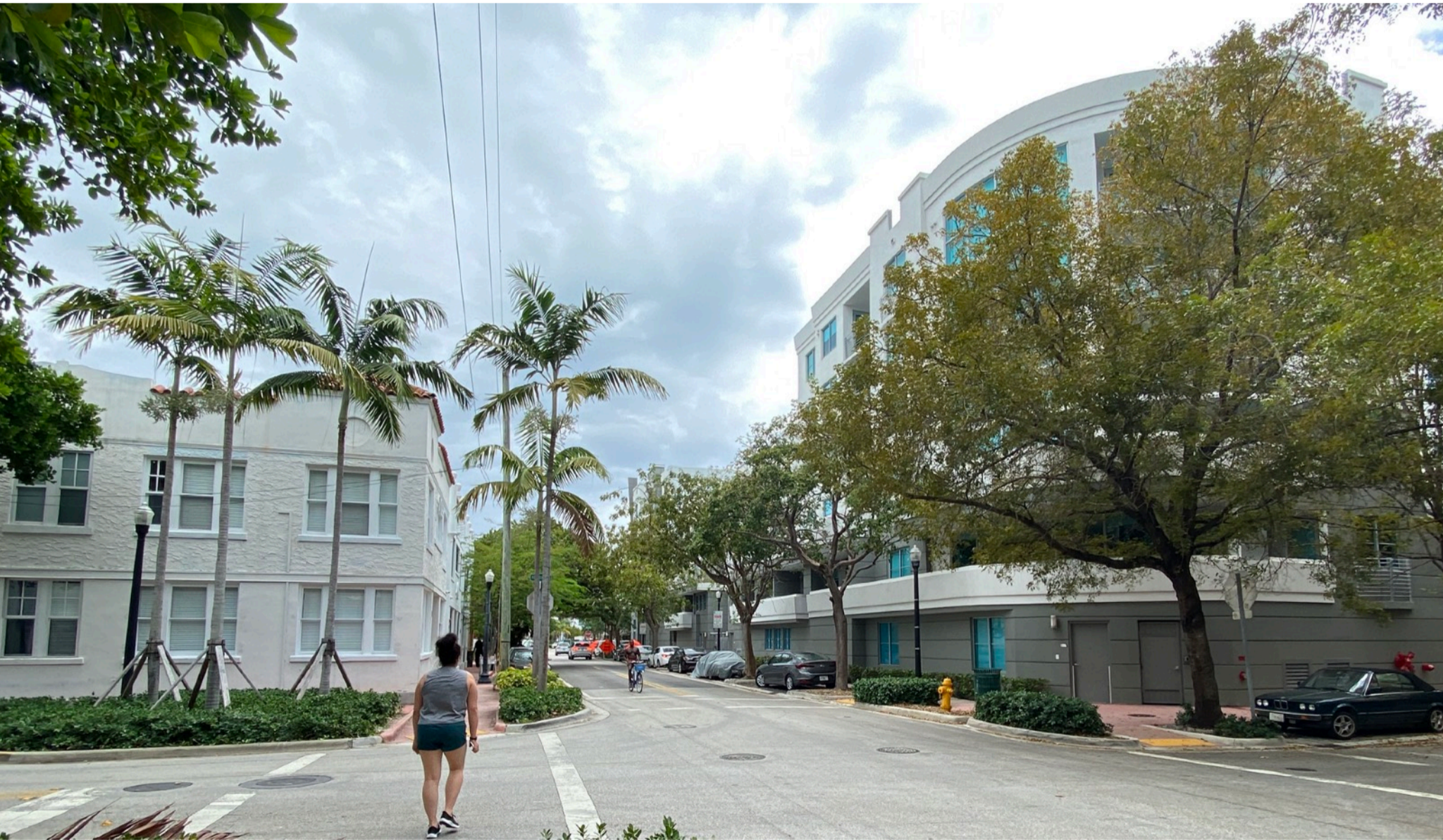
TOP: 2021 VIEW LOOKING NORTH ON MERIDIAN AVENUE FROM 2nd STREET
