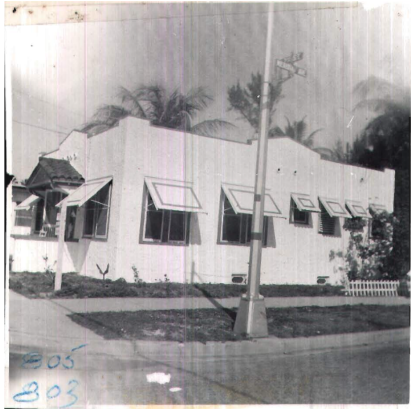
1973 PHOTOGRAPH of 803 / 805 2nd STREET
