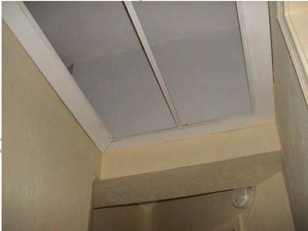
Interior view of original entrance header above the front porch.
