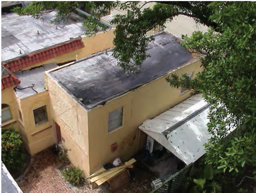
Aerial south view of La Corona Annex residence
