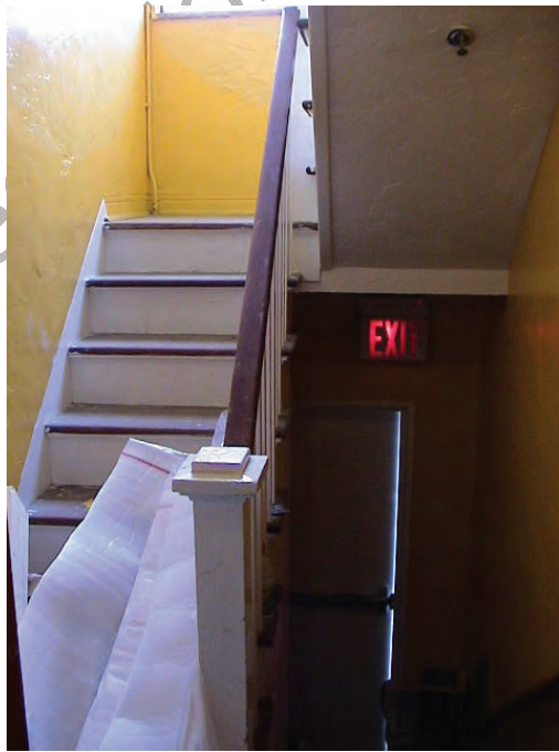
Interior view of South Stair at ground level.
