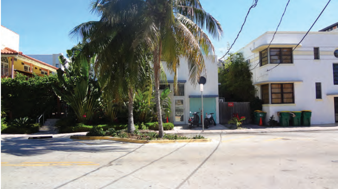
North view of kitchen east of Pancoast Residence.
