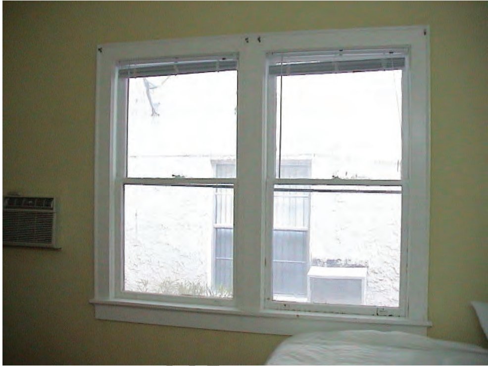
Interior view of original window frame at east facade.
