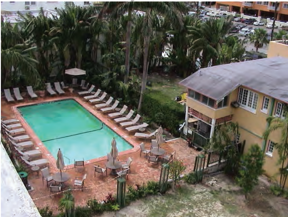
Aerial southeast view of swimming pool, deck and Pancoast Residence
