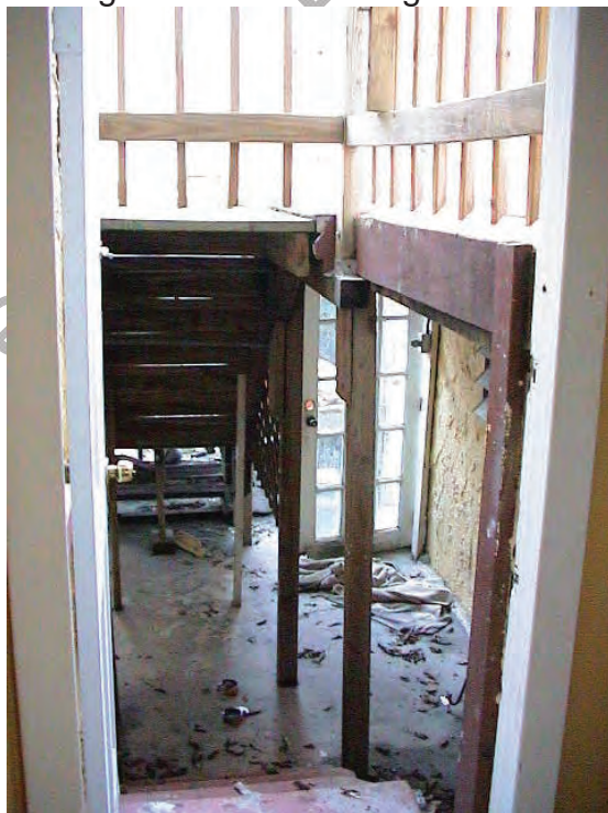
View of non-original door, and wood deck looking south.
