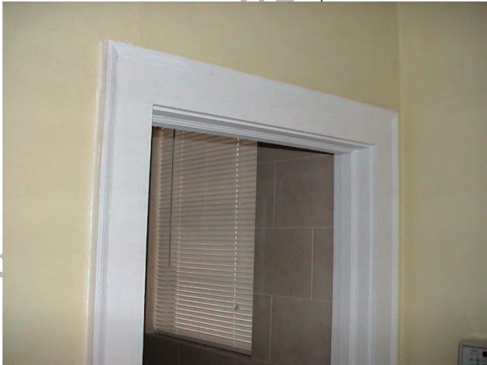
Interior view of original door frame towards the north.
