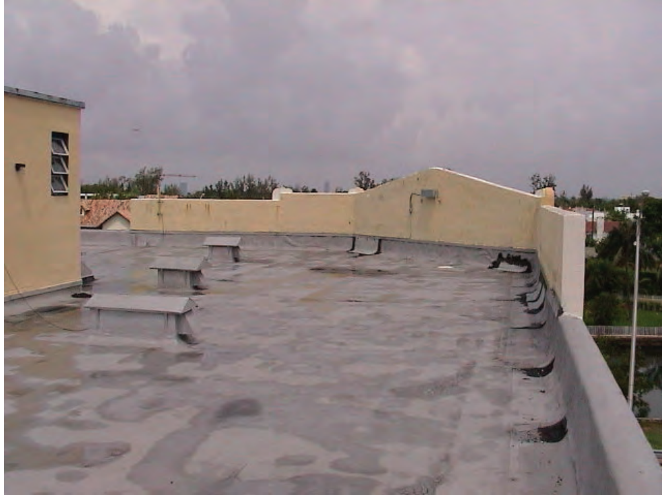
View from the roof of the northwest parapet.
