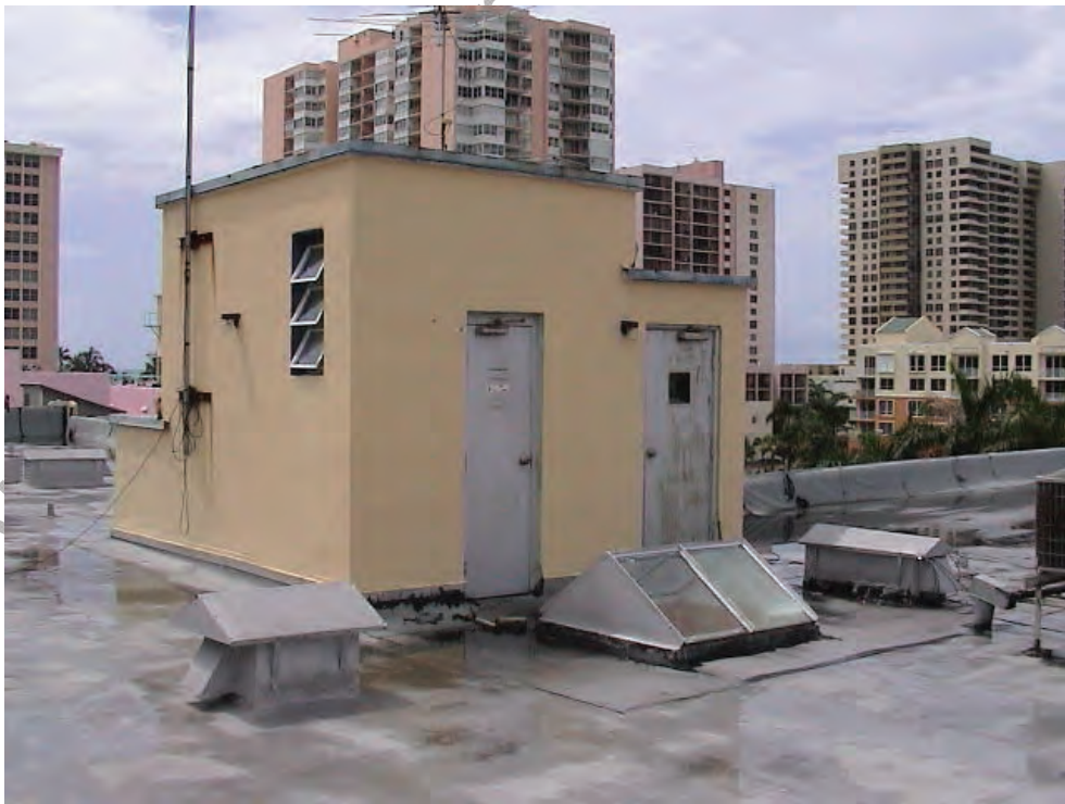
Northeast elevation of elevator machine room & stair door.
