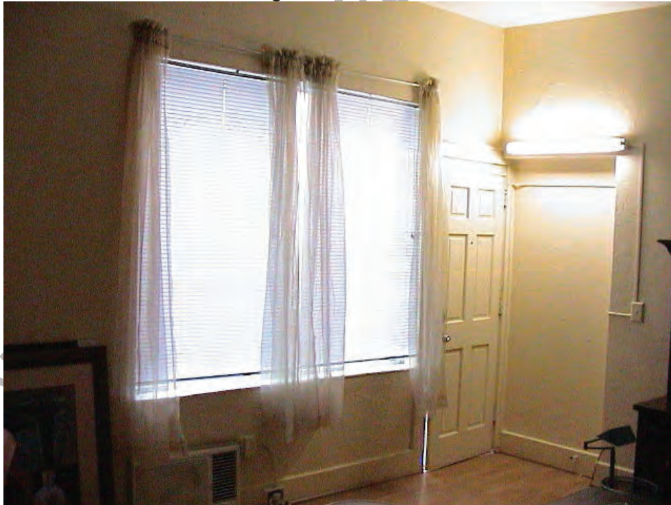
Interior view of non-original window & door looking west
