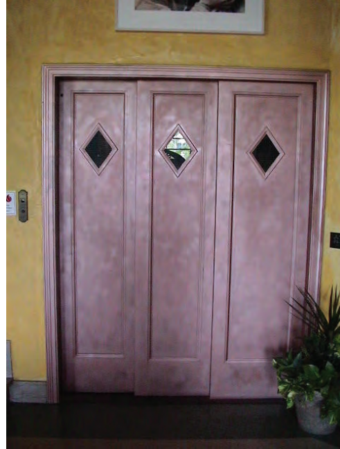
Interior view of Elevator Lobby door.
