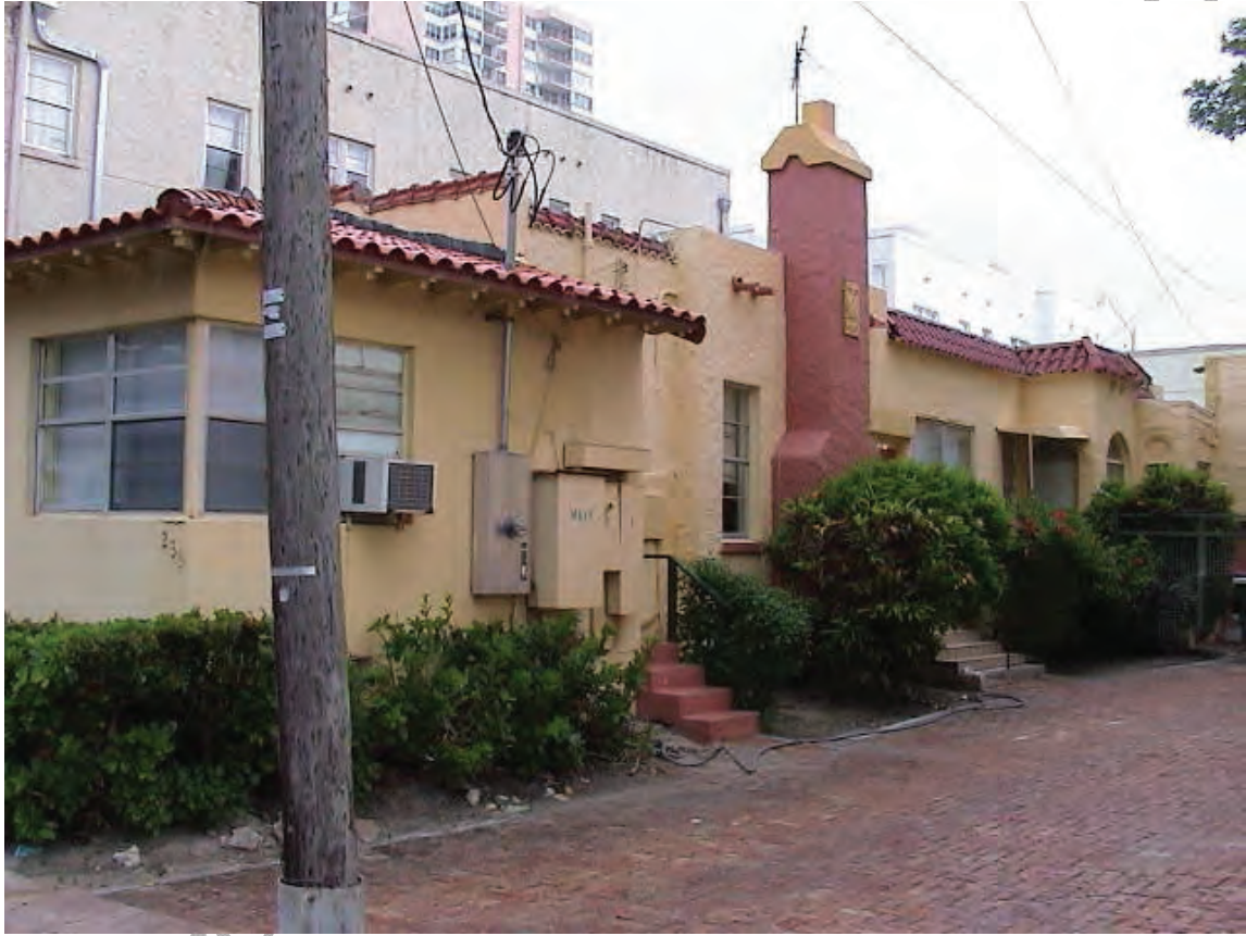
West Elevation of La Corona Annex Residence.
