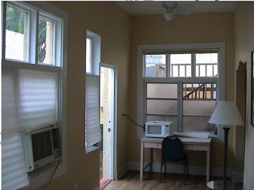
Interior southwest view of rear porch and non-original glass.
