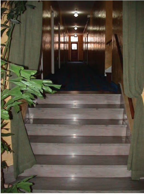
Interior view of west corridor from lobby.
