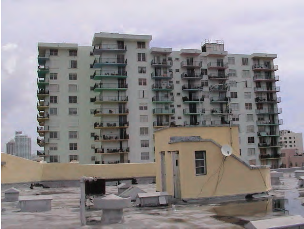
Southwest view of elevator machine room & stair door
