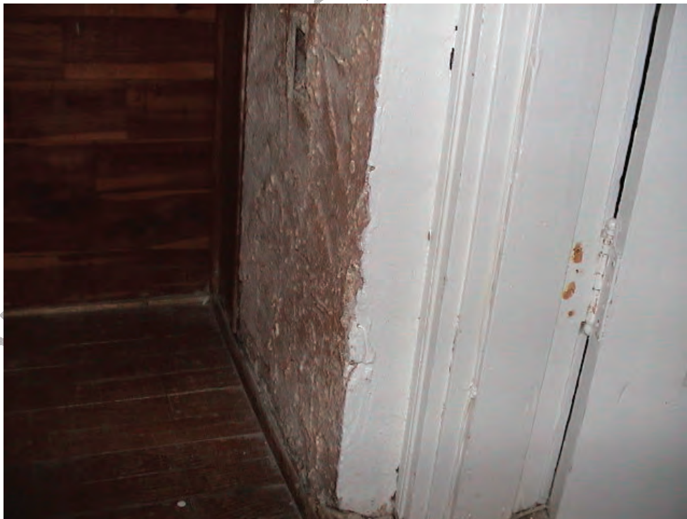
Interior view of original stucco from the front porch.
