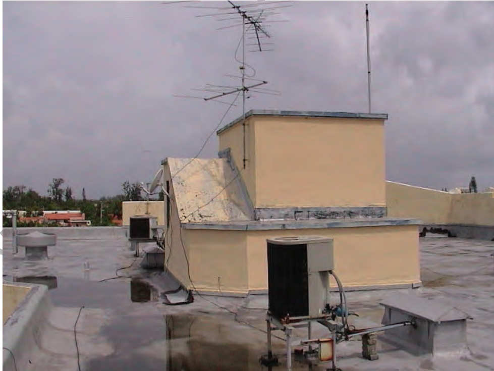
View from the roof to the west.
