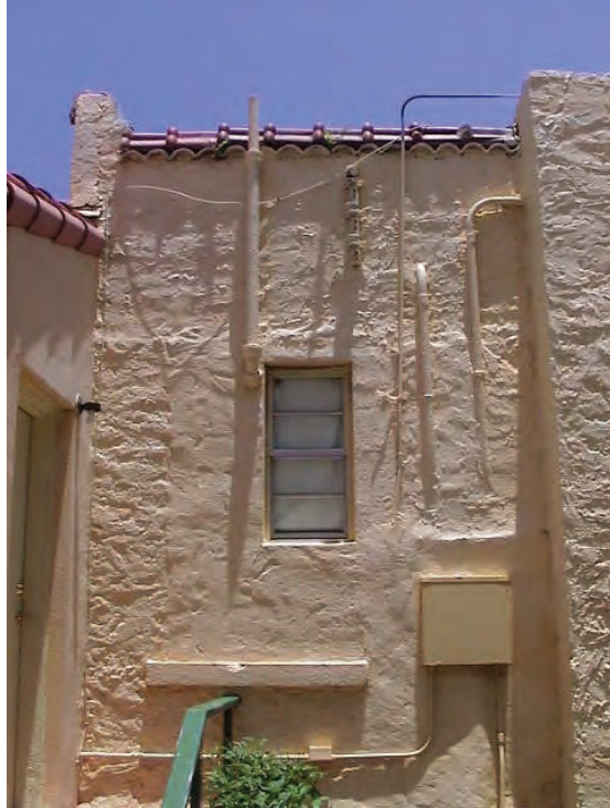
Tiles at the west façade & blocked in original porch.
