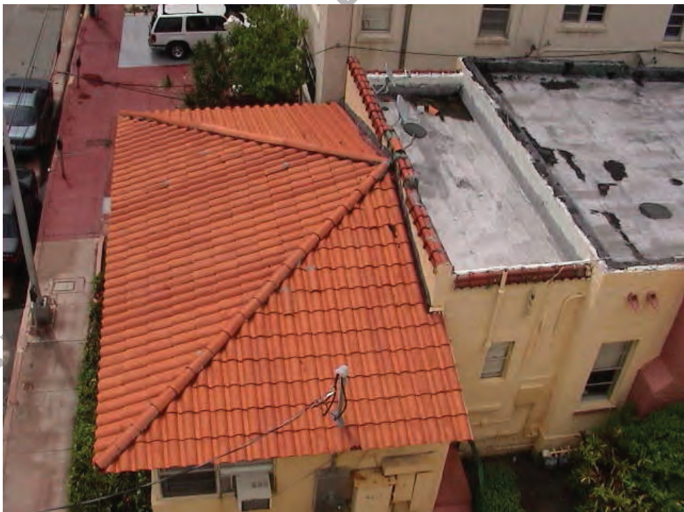
Aerial northeast view of La Corona Annex residence.
