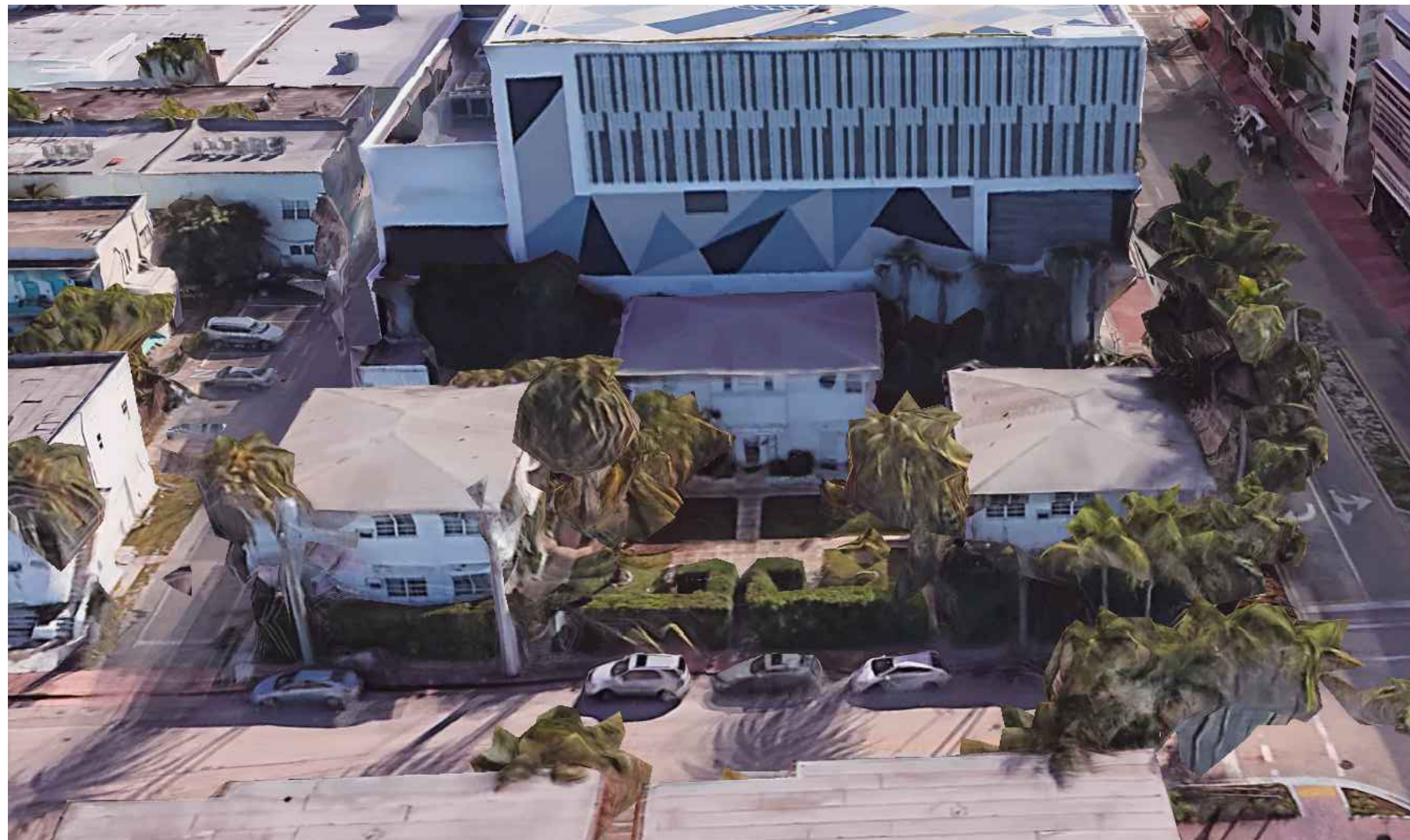
AERIAL VIEW OF COURTYARD
