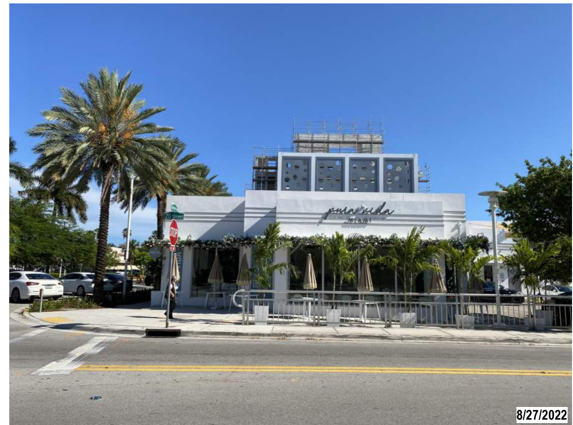
2. VIEW OF EXISTING STRUCTURES FROM 20TH STREET
