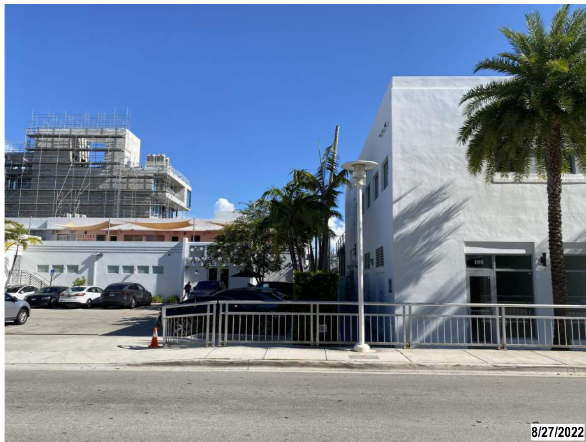
3. VIEW OF EXISTING STRUCTURES FROM WEST AVENUE
