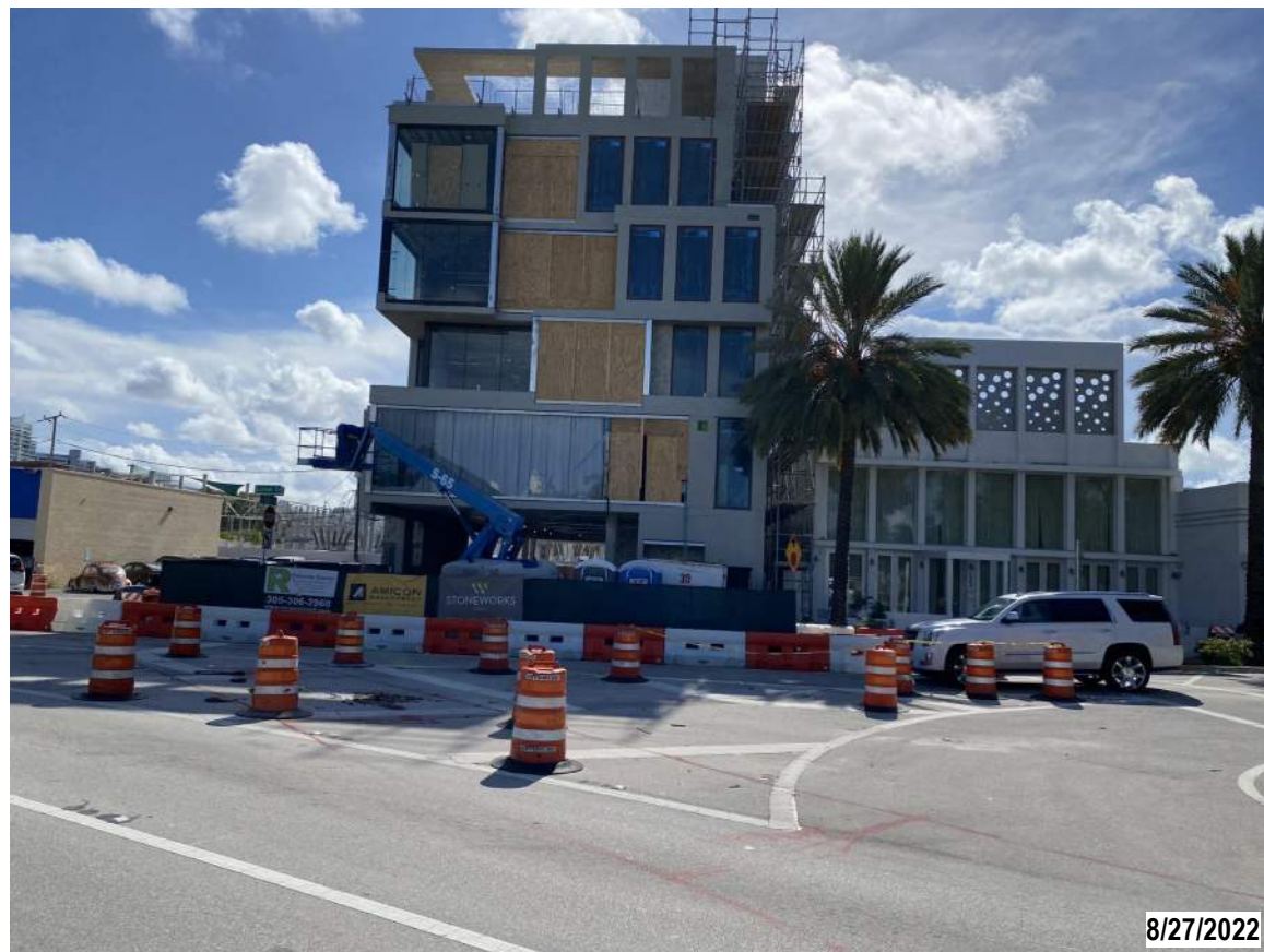
1. VIEW OF EXISTING STRUCTURES FROM ALTON ROAD
