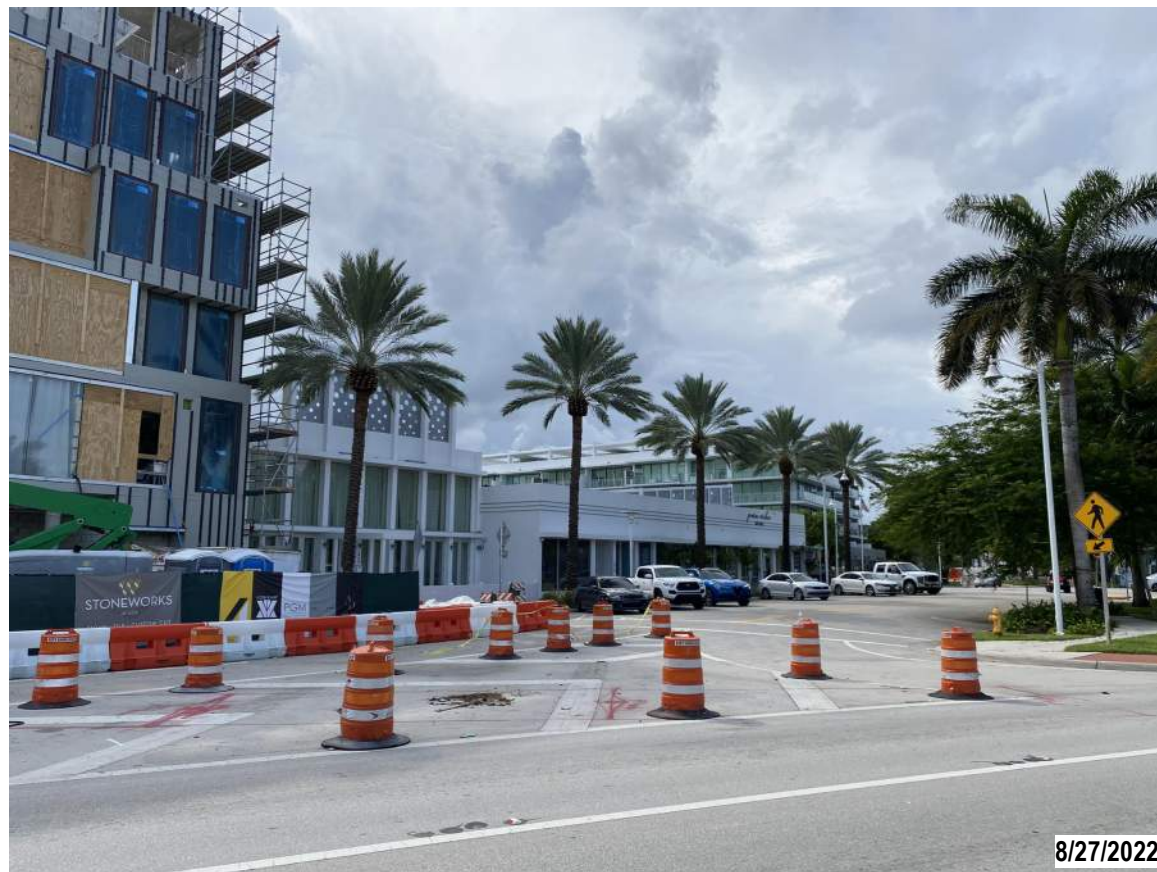
1. VIEW OF SITE FROM ALTON ROAD
