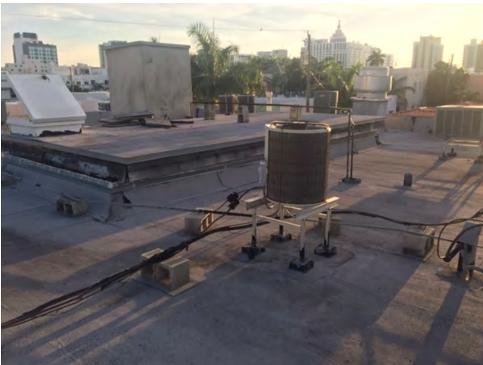
Roof North view
