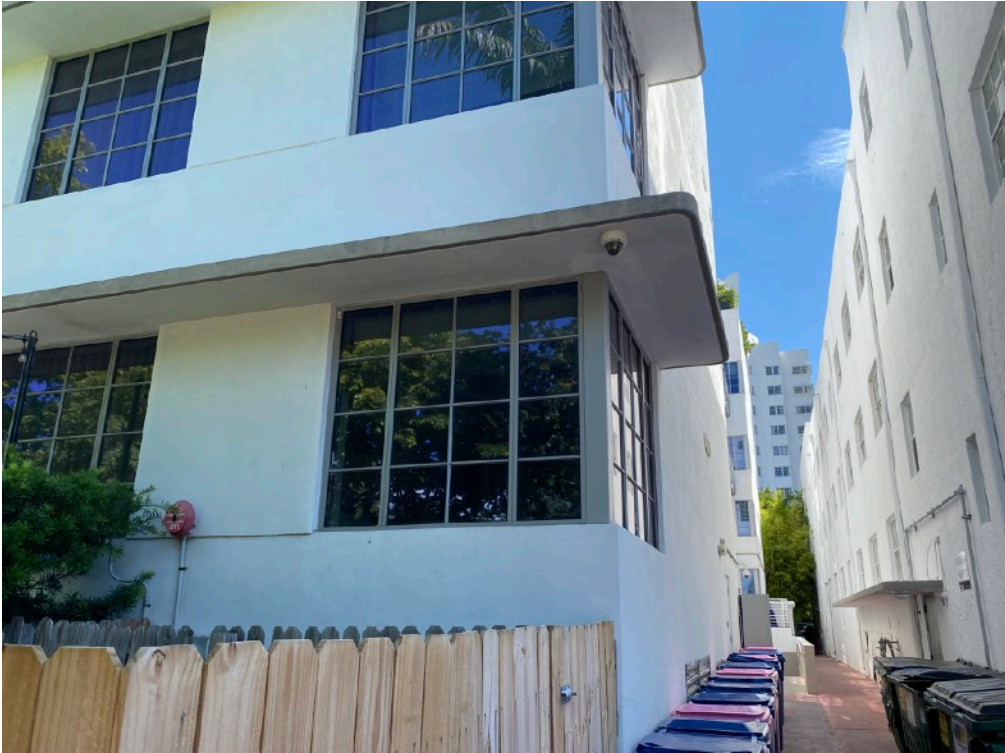
View of SW Corner of Regent Building
