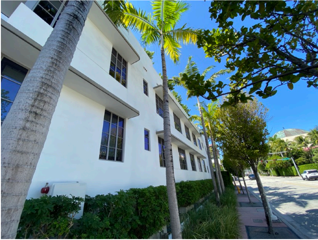
View of North Facade of Regent Building
