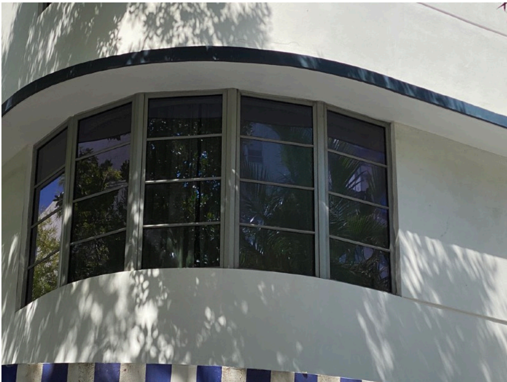
Detail of SE Corner Facade of Gale Hotel
