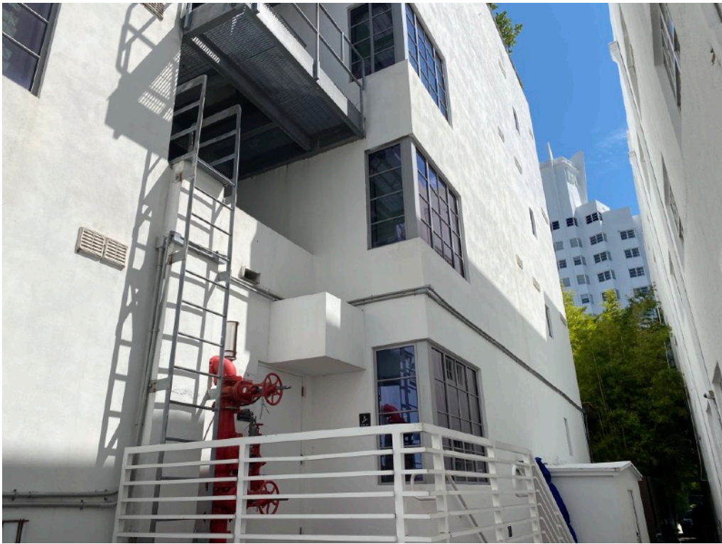
View of South Facade – Gale Side
