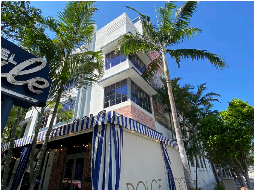
View of NE Corner of Gale Building
