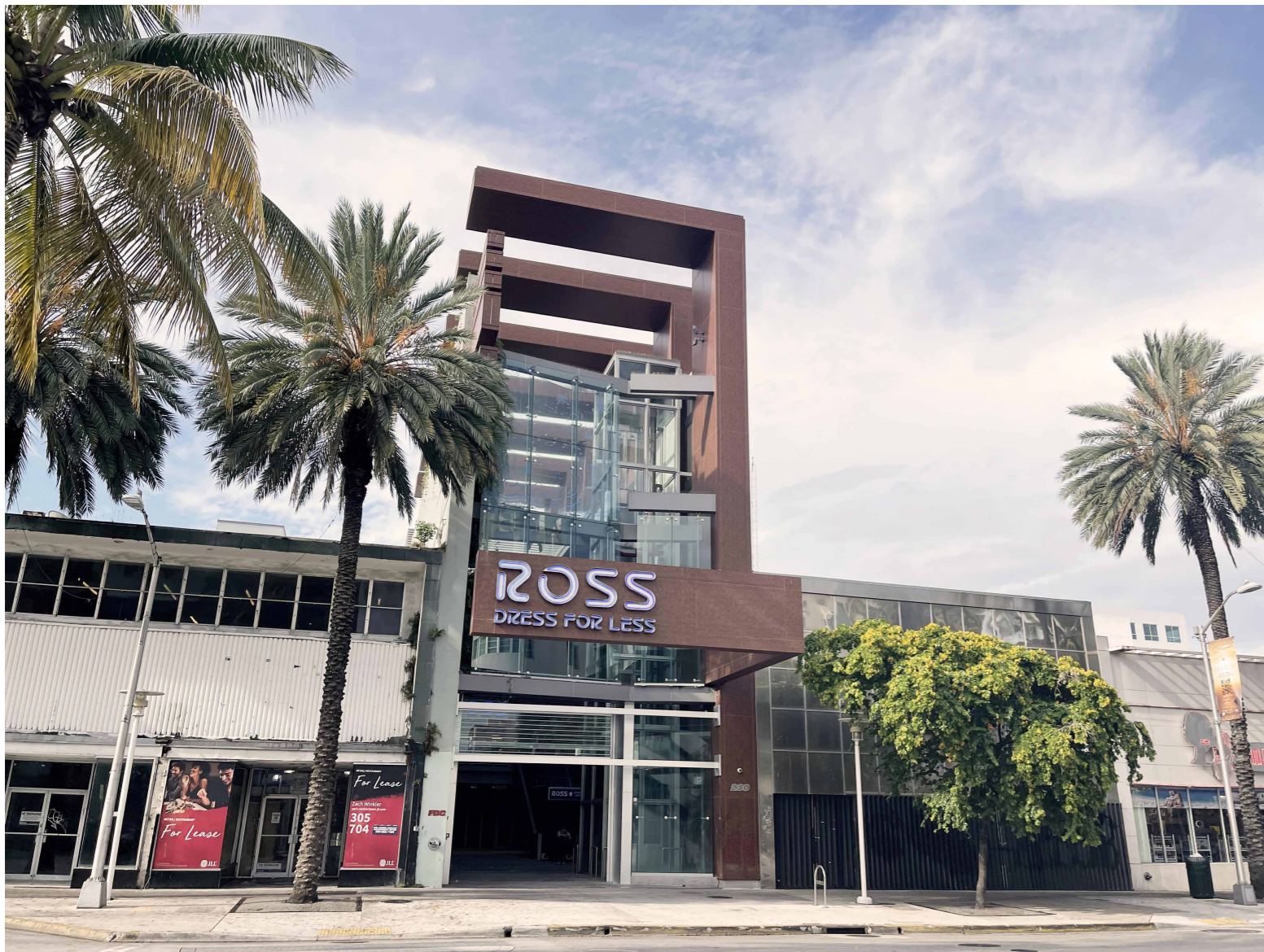
13. RETAIL SHOPS - VIEW FROM JAMES AVE & LINCOLN RD
