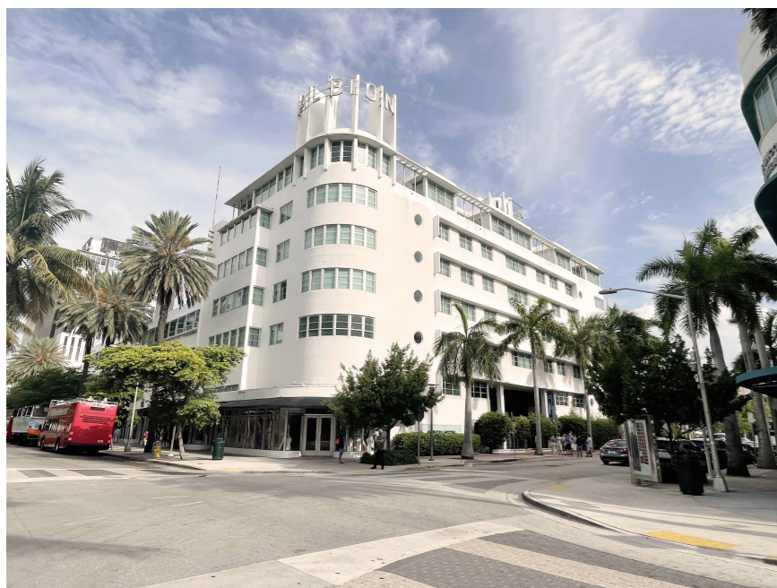
14. ALBION HOTEL - VIEW FROM LINCOLN RD
