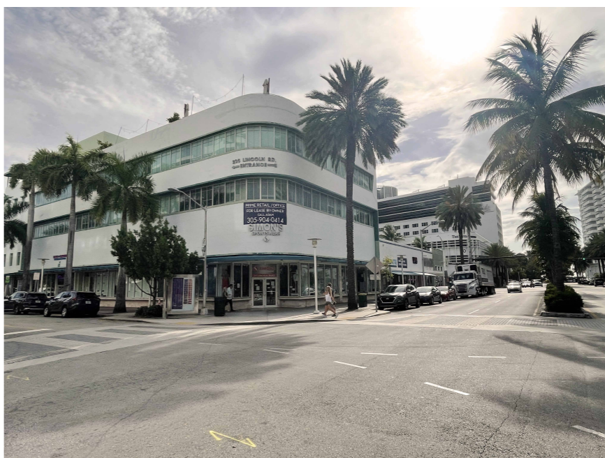
16. RETAIL / OFFICE BUILDING - VIEW FROM LINCOLN RD
