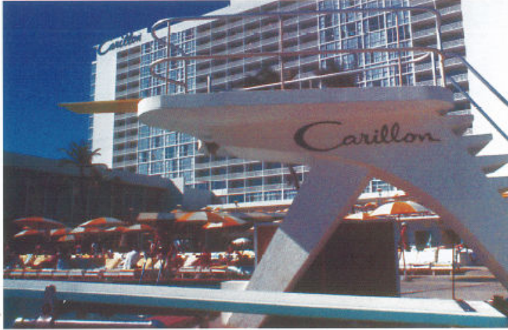
Carillon Hotel, Miami Beach, 1957–58 (altered). View of the guest tower, as seen from the pool area. Since the façade's glass walls were not load-bearing, I was free to place them wherever I liked. Recessing the wall created a balcony space, while placing it flush enabled sun to directly stream into the room for a longer period of time. By alternating recessed and flush sections, I was able to create a simple pattern.
