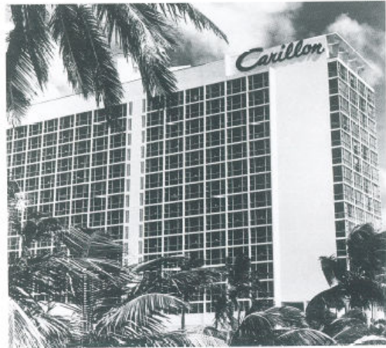
Carillon Hotel, Miami Beach, 1957–58 (altered). North elevation. True to modernist form, I used the structural grid pattern as a decorative element. The horizontal lines, for instance, are the six-inch concrete slabs that support each floor. I used aluminum window frames to create a secondary grid, reinforcing the rhythm of the first.
