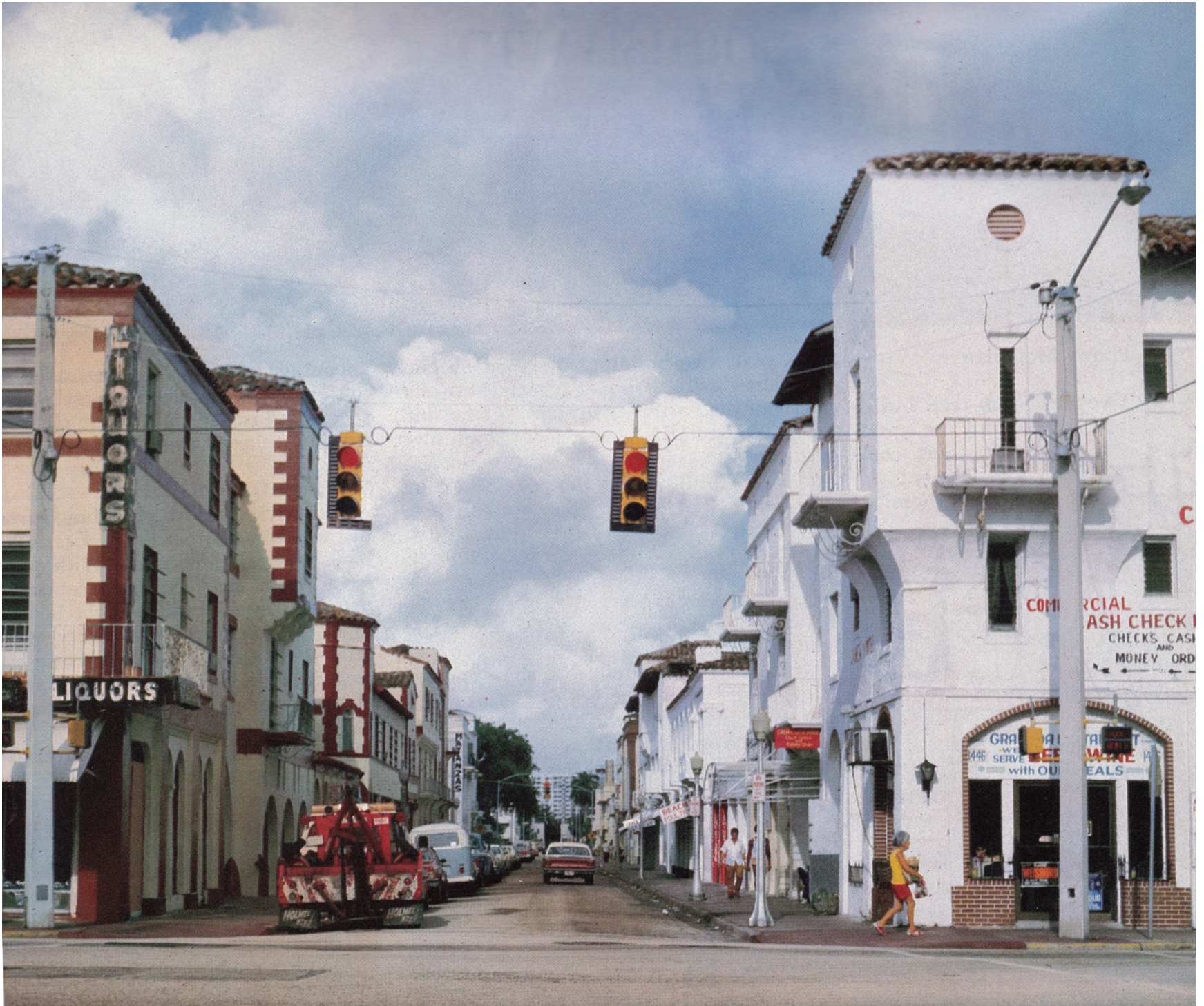
1980 PHOTOGRAPH LOOKING WEST ON ESPANOLA WAY WITH CLAY HOTEL AT LEFT (5)
