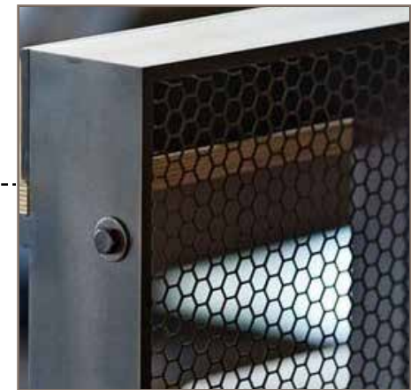
MESH AT BLACK STEEL HEADER
