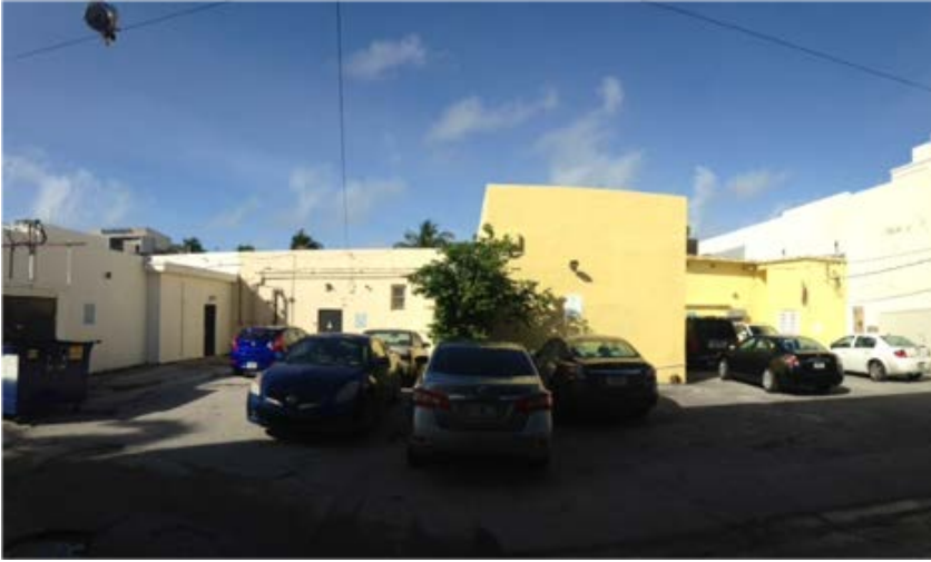
TOP: 2016 PHOTOGRAPH OF REAR (EAST) ELEVATION (3)
