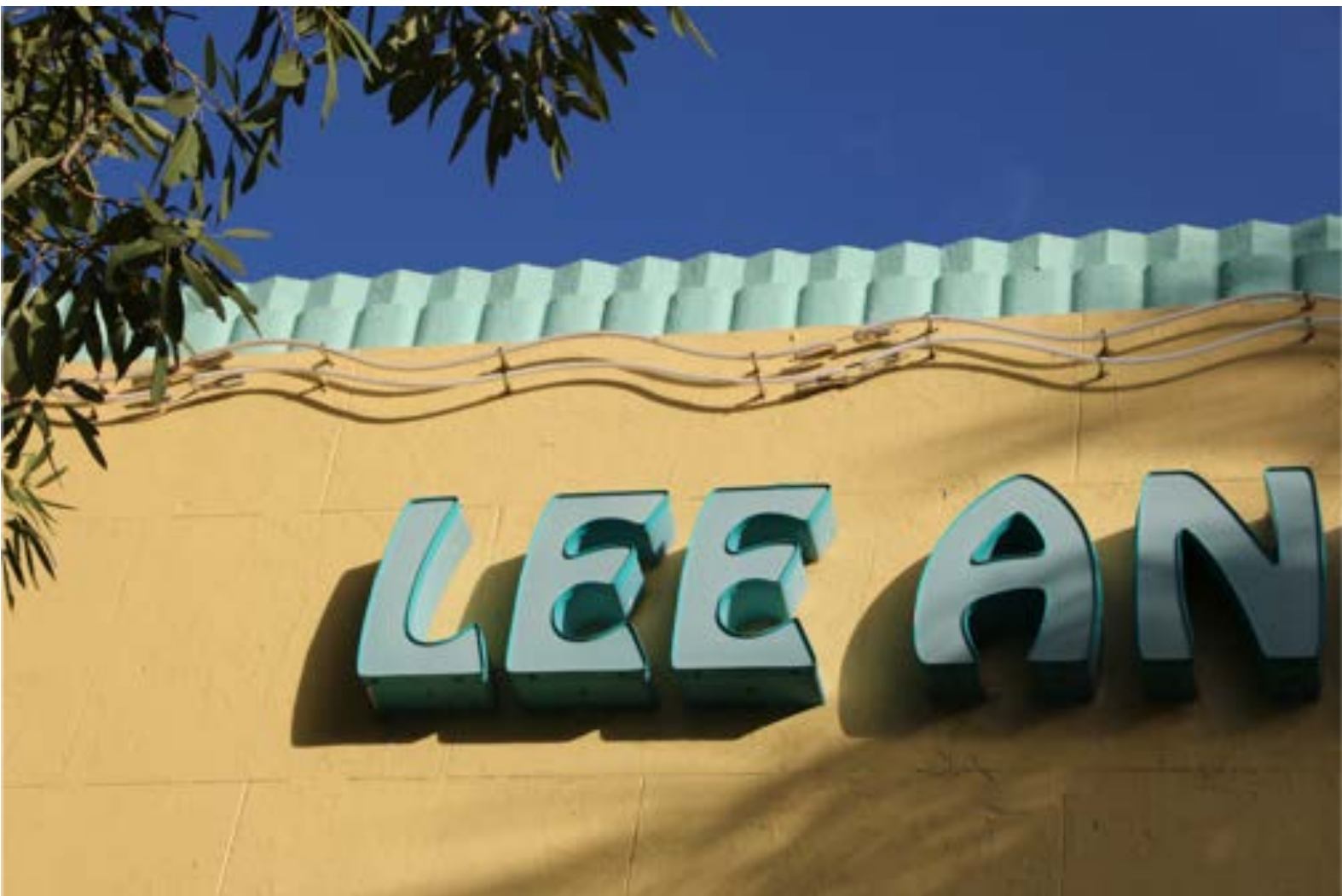
2016 PHOTOGRAPHS of PARAPET DETAIL AT 955 WASHINGTON AVENUE (3)
