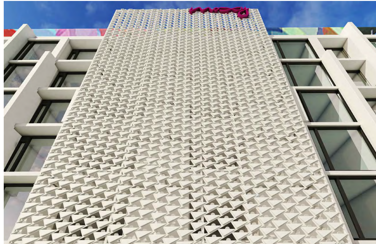
VIEW UPWARD FROM COURTYARD
