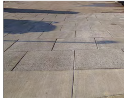
07 | Loading & Parking Pervious Concrete
