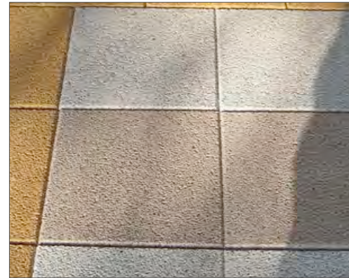
08 | Loading & Parking Pervious Concrete
