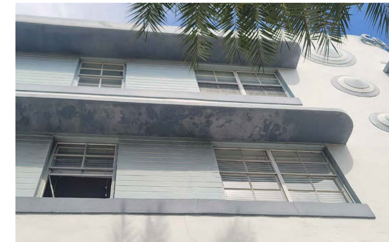
EXISTING STUCCO BAND TO BE RESTORED
