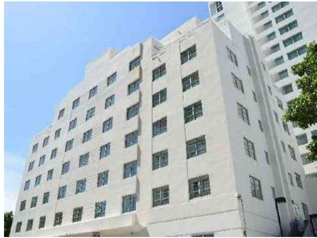
VIEW OF NORTH ELEVATION OF FORMER CROMWELL
