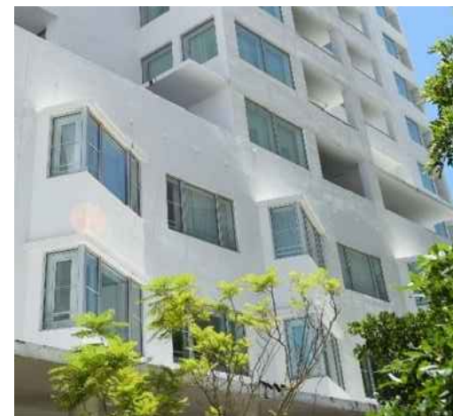
DETAIL ANGLED WINDOWS UNDER TOWER
