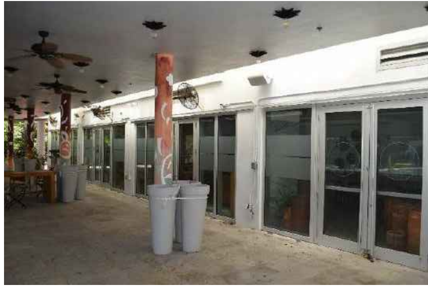
DETAIL OF STOREFRONT AT EAST ELEVATION
