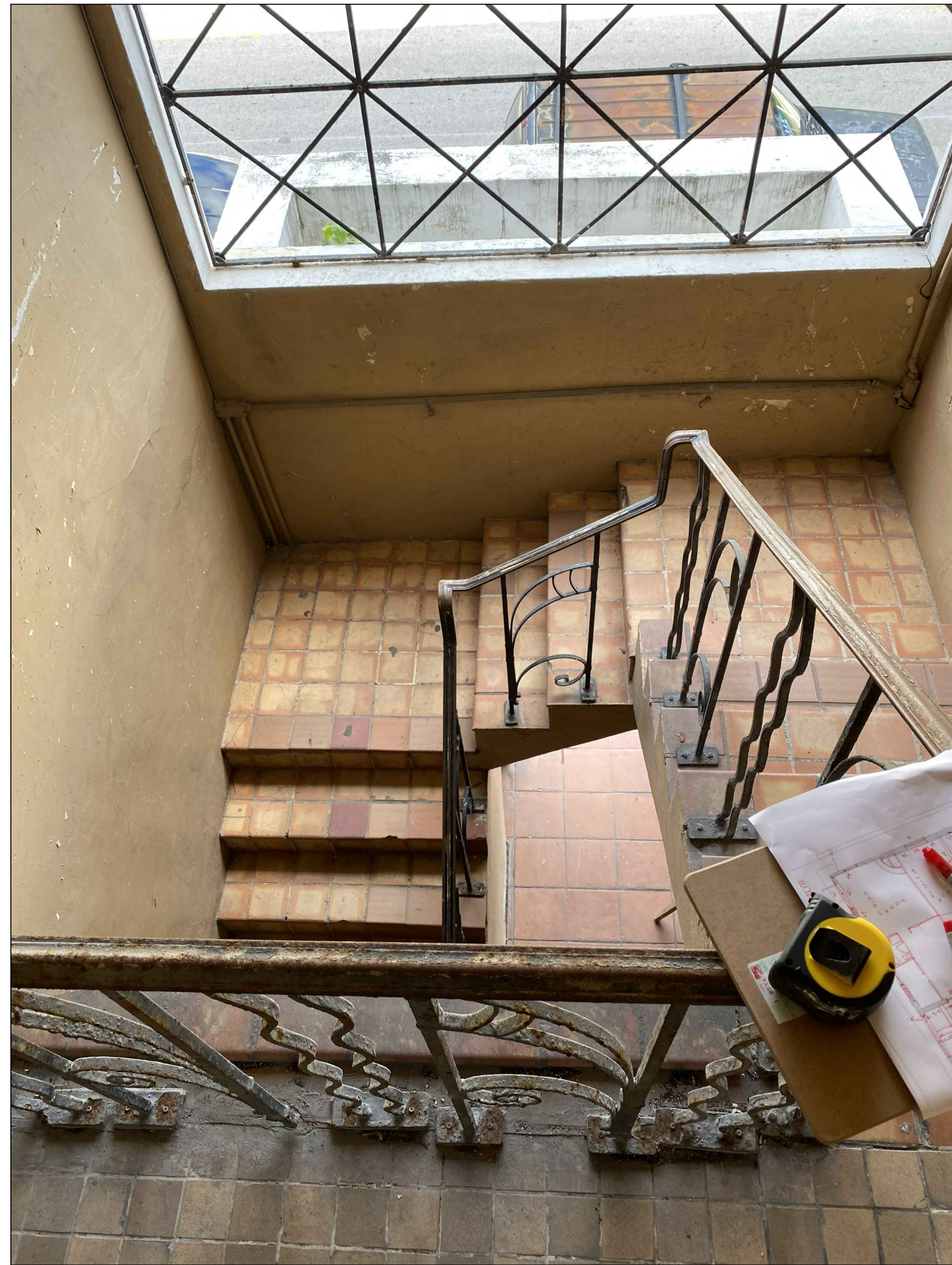
VIEW 4 STAIR WEST VIEW
