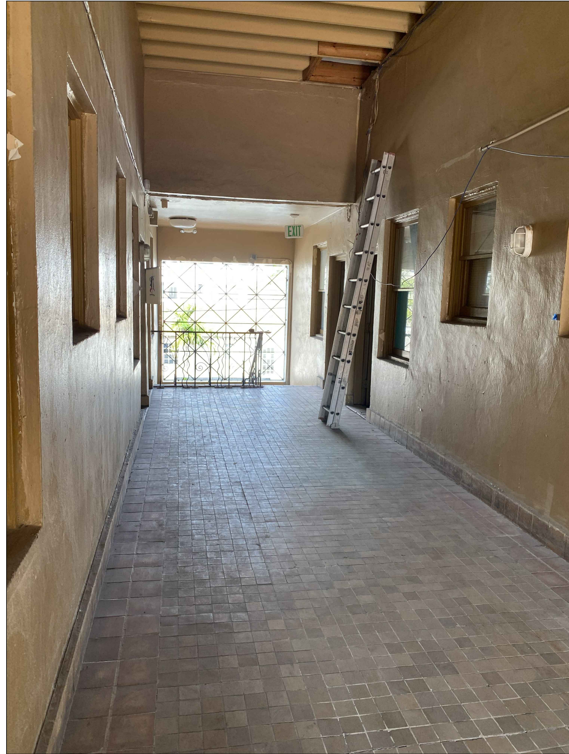
VIEW 1 CORRIDOR WEST VIEW
