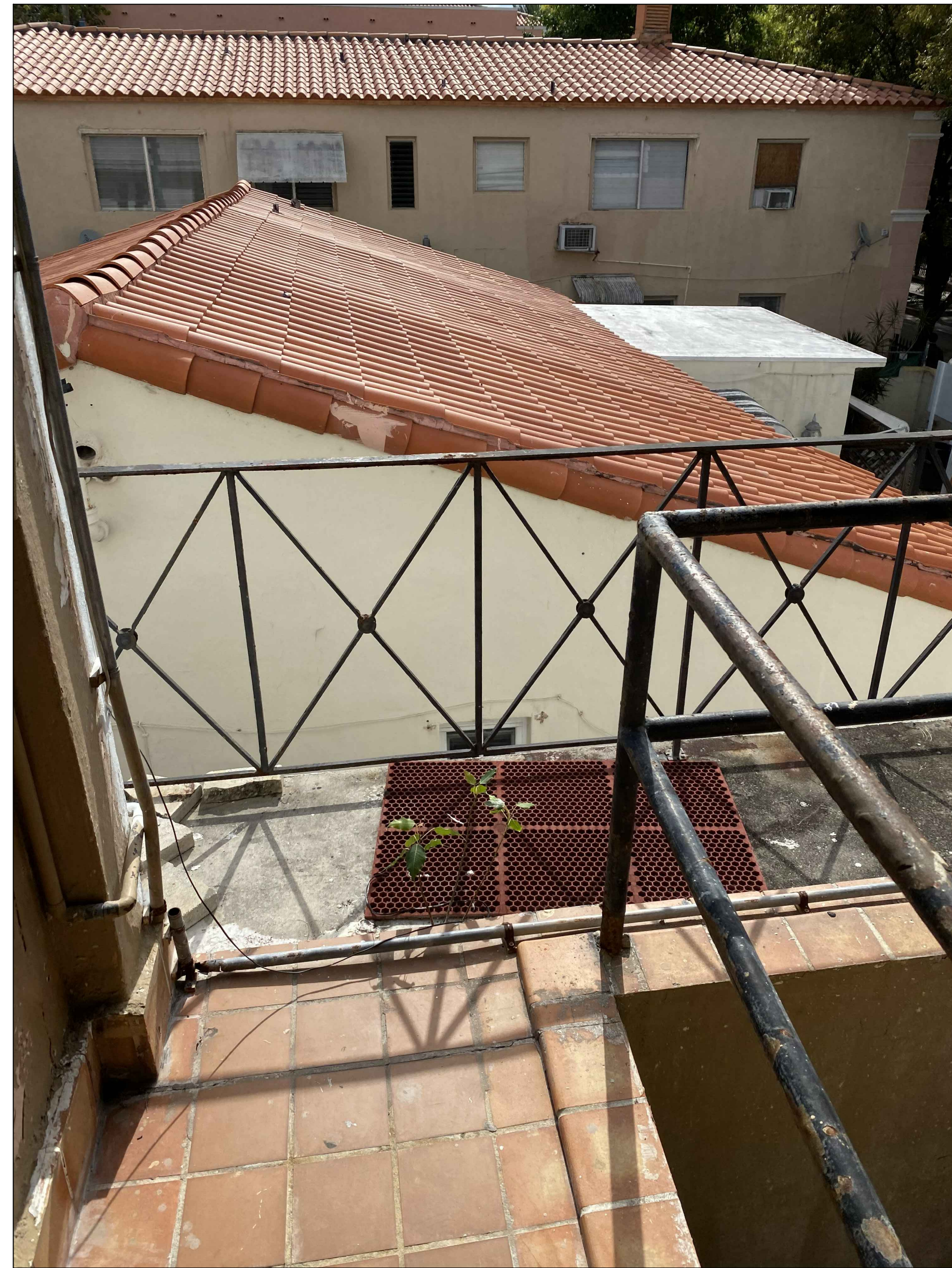
VIEW 5 BALCONY EAST VIEW
