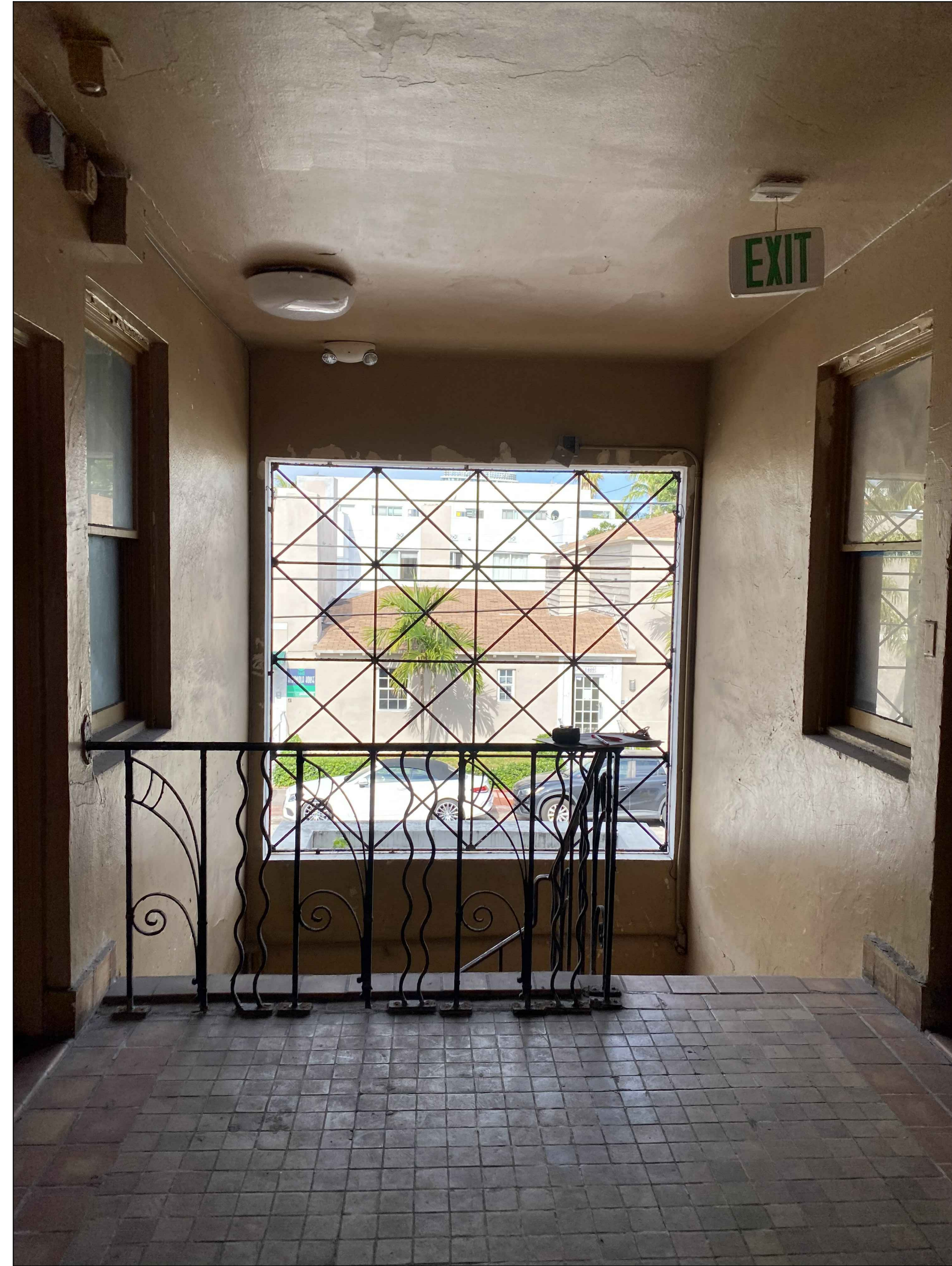
VIEW 2 CORRIDOR WEST VIEW
