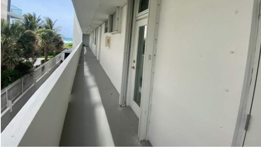
Existing catwalk prior to restoration
