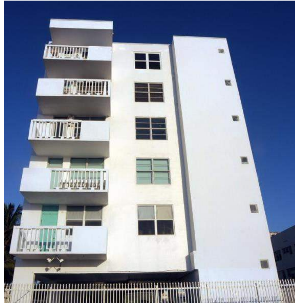
Existing Balcony Guardrails
