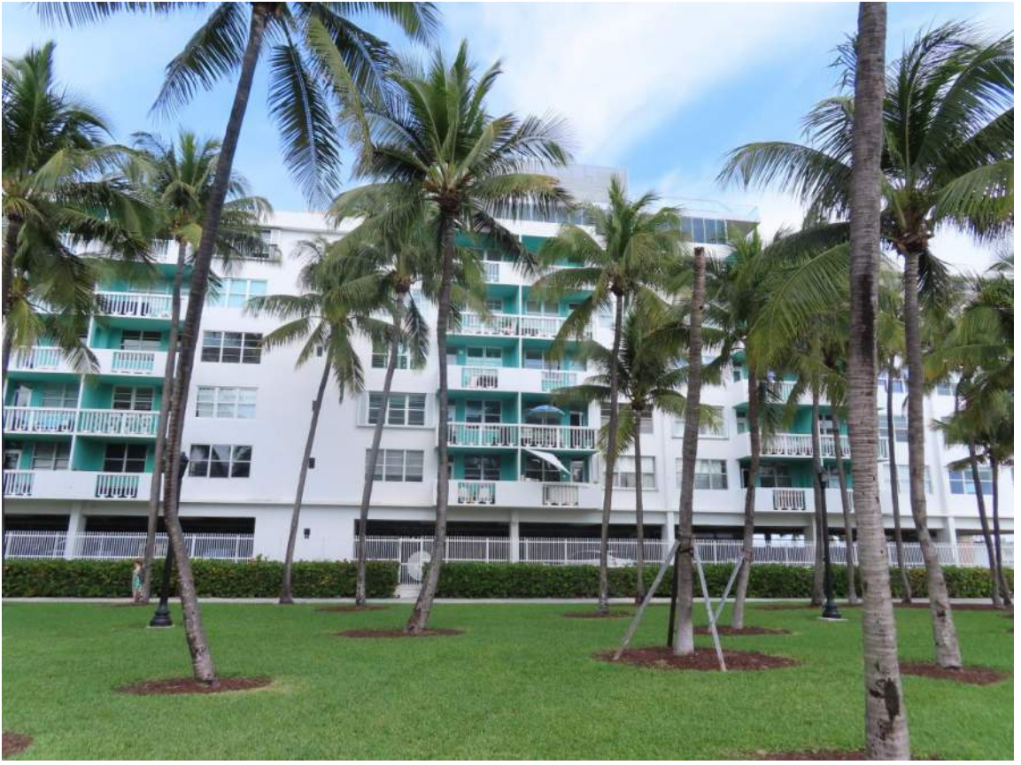
Existing Balcony Guardrails
