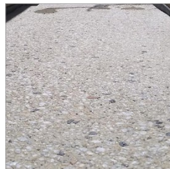
Acid Etch Concrete Finish
