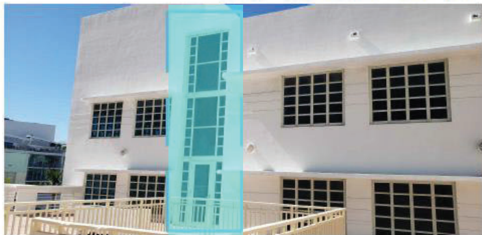
VIEW OF AREA TO REMOVE AT LEVEL 3 TO BE REMOVED
