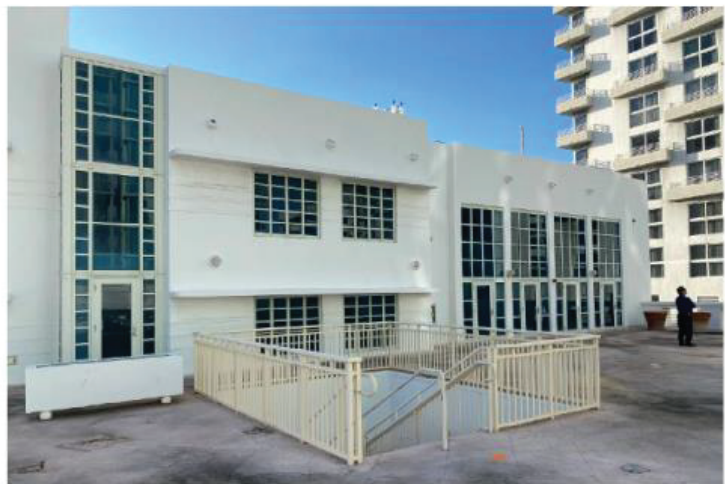
PHOTOS OF LEVEL 3 TERRACE EXISTING CONDITIONS
