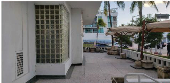
REFERENCE VIEW OF EXISTING GLASS BLOCK AT GROUND LEVEL (TO REMAIN)
