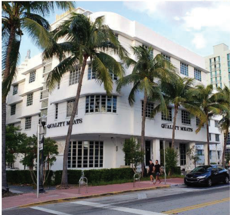
EXISTING CORNER FACADE
