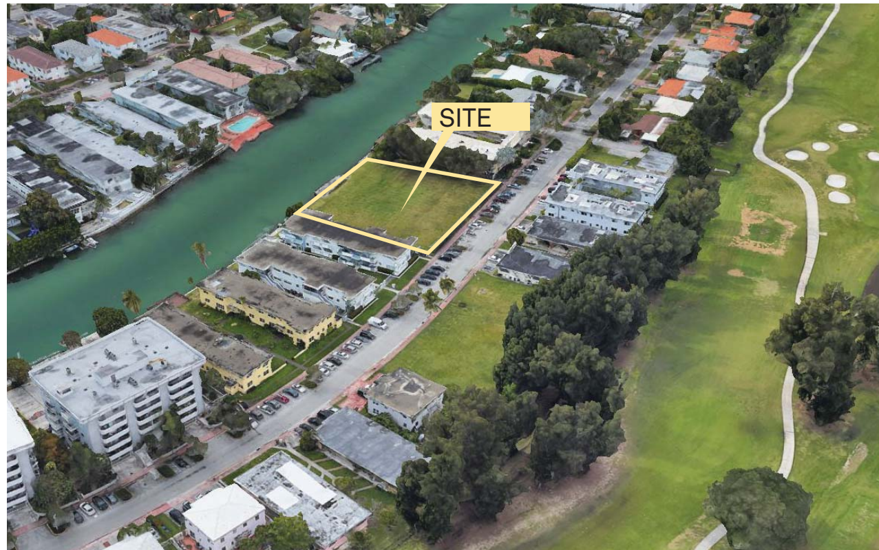
AERIAL VIEW / FROM NORTHEAST
