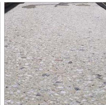
Acid Etch Concrete Finish
