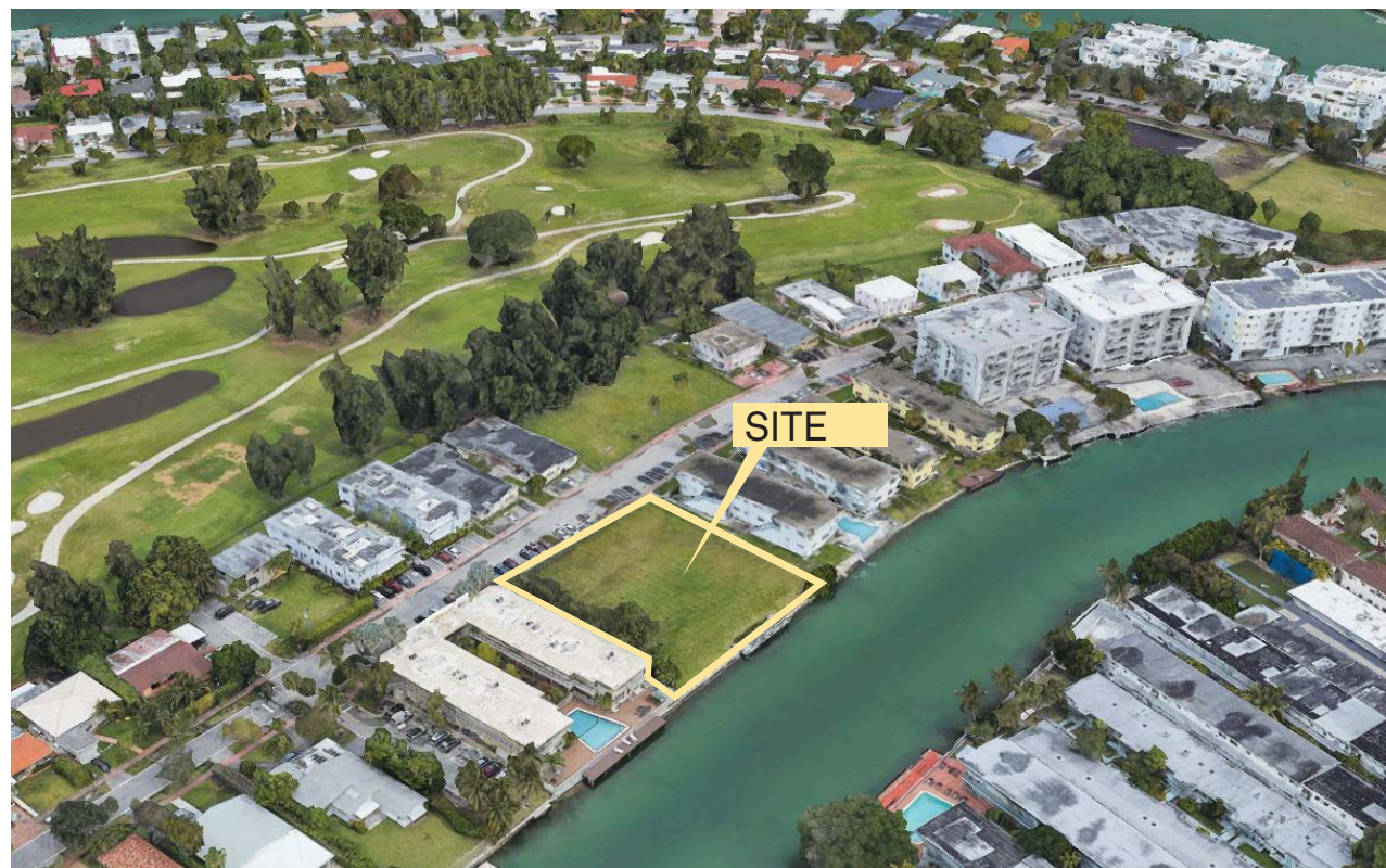
AERIAL VIEW / FROM SOUTHWEST
