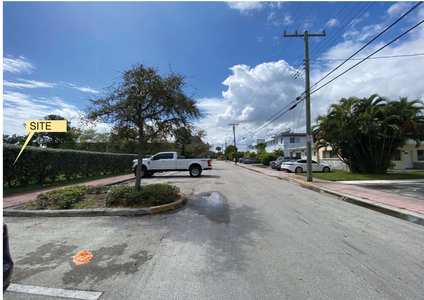
S. SHORE DRIVE, LOOKING WEST
