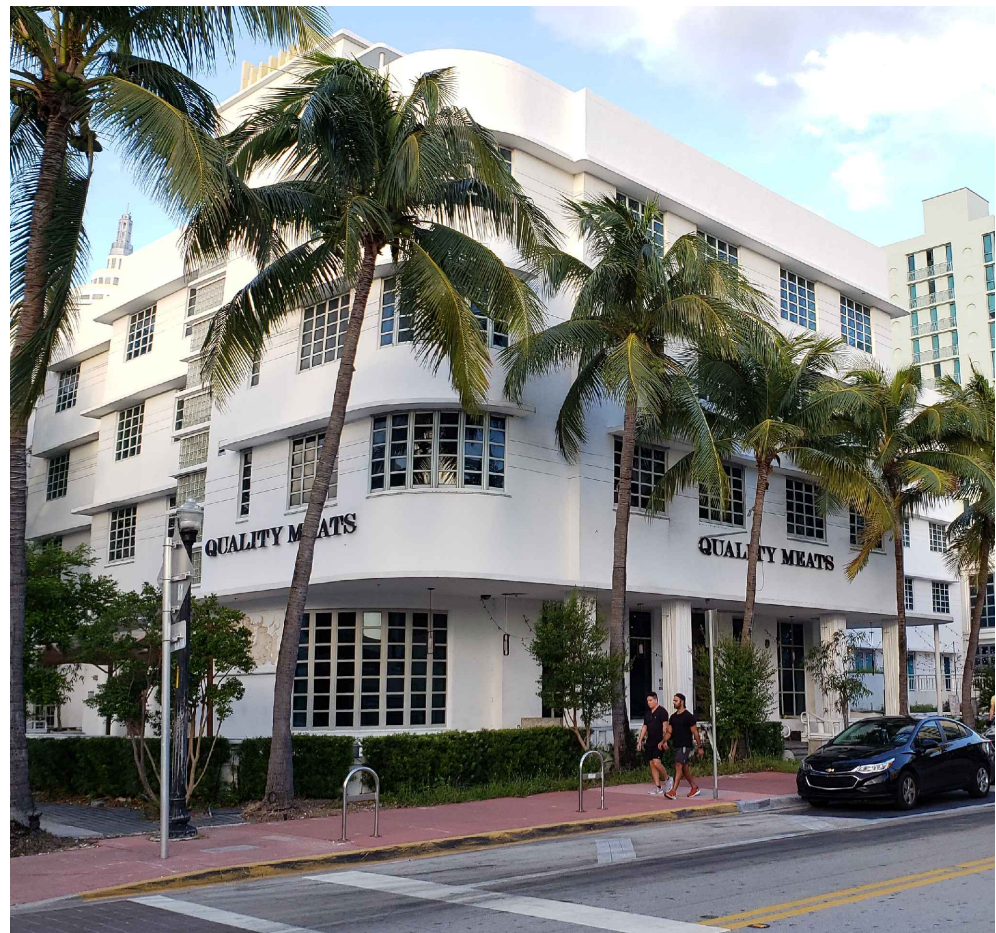
EXISTING CORNER FACADE
