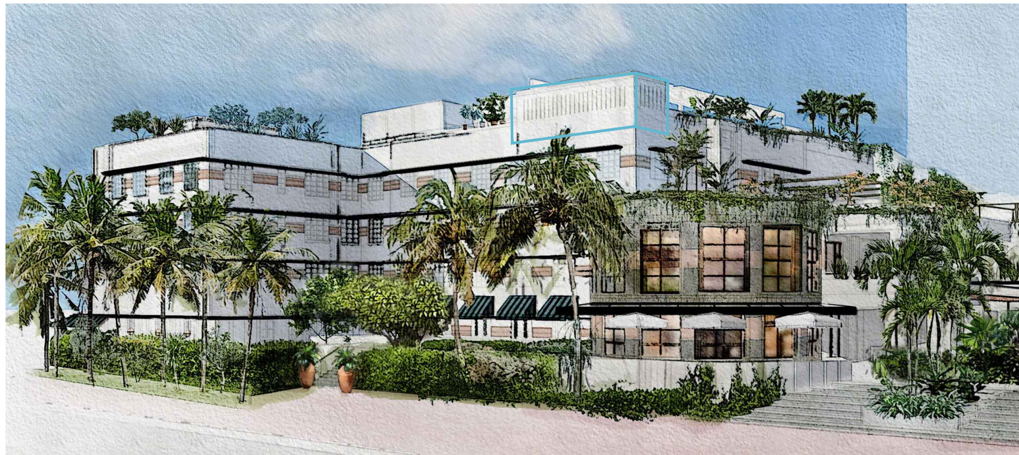
EXTERIOR VIEW FROM 15TH STREET
