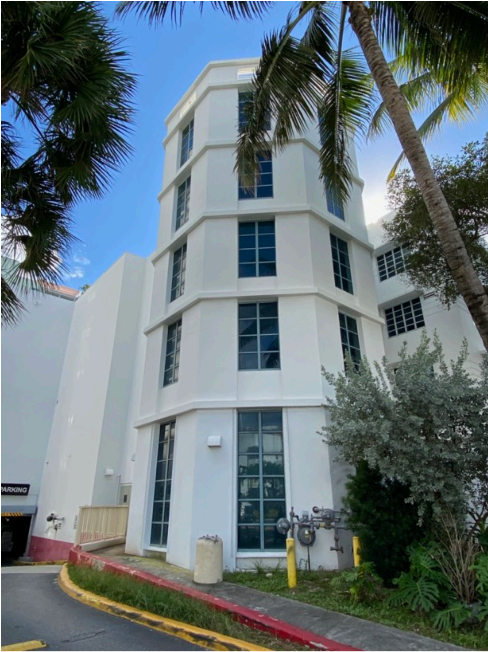
PHOTO of the OCTAGONAL TOWER AT NORTH END OF HISTORIC BUILDING ALONG COLLINS AVENUE.
