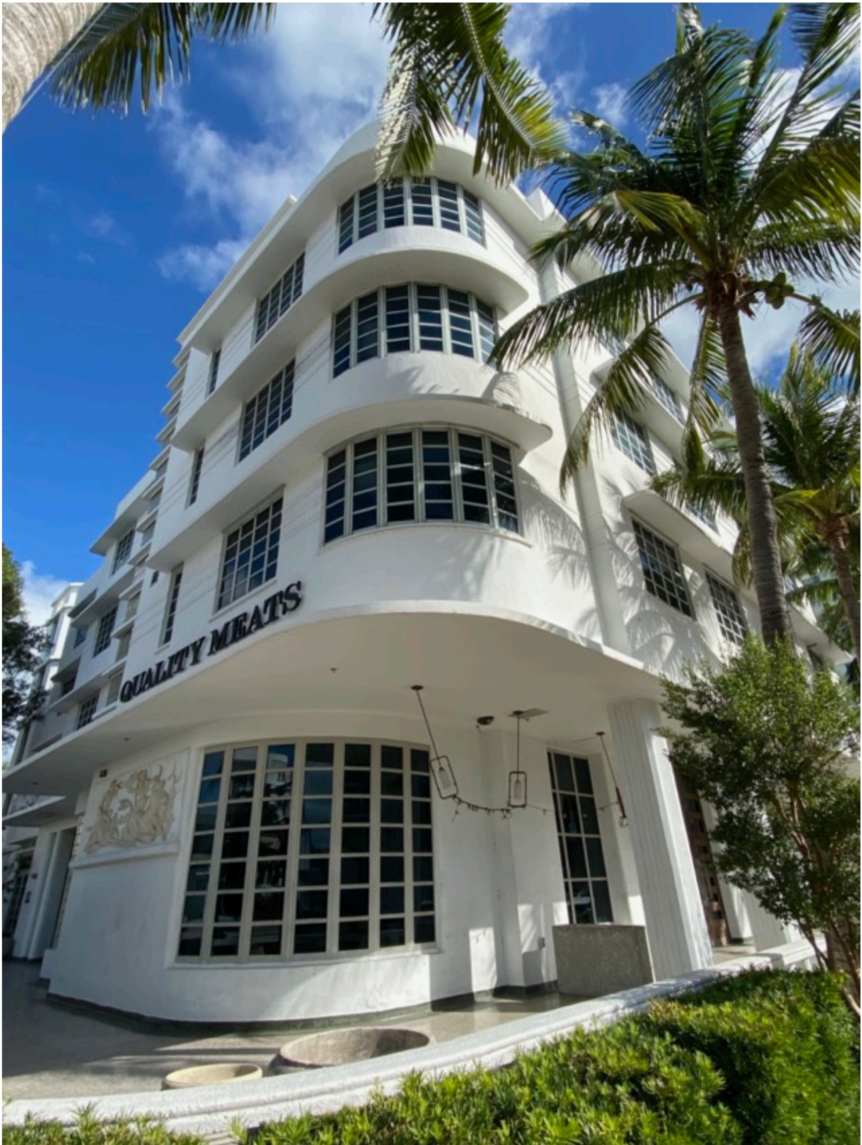
2020 CORNER VIEW SHOWING CONCRETE SUNSHADES AND THE EARL LE PAN MURLA AT THE FIRST FLOOR FACING COLLINS AVENUE.
