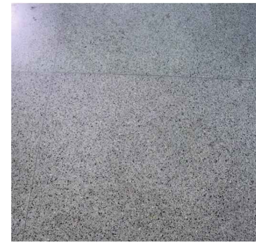
DETAIL TERRAZZO PAVING AT ENTRANCE WEST ELEVATION
