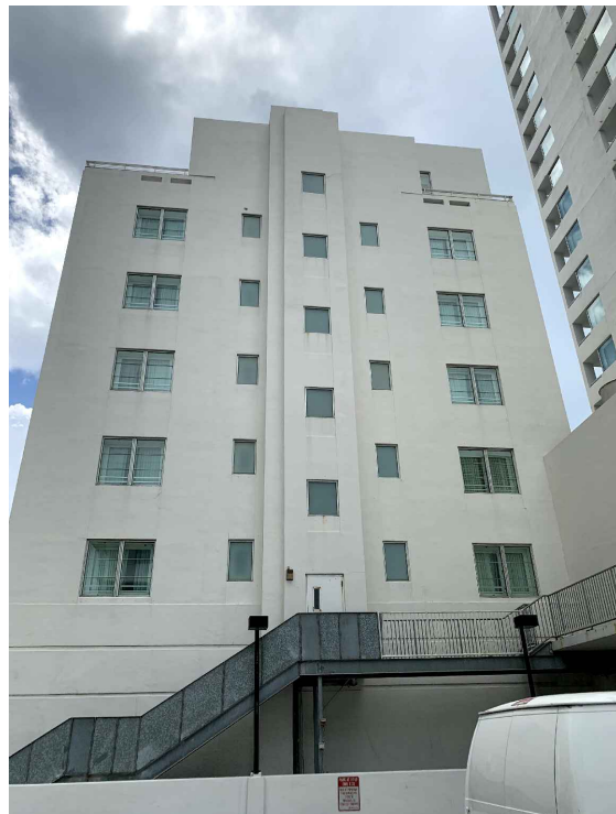
DETAIL OF FENESTRATION PATTERN AT WEST ELEVATION
