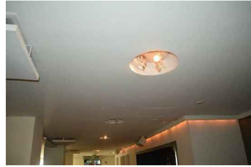
DETAIL OF CEILING FINISH AND RECESSED LIGHT FIXTURE AT LOBBY
