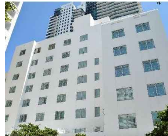
DETAIL OF FENESTRATION PATTERN AT SOUTH ELEVATION
