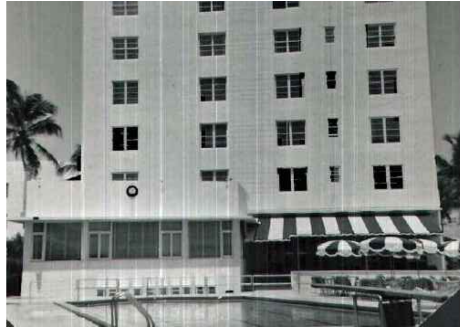
DETAIL OF HISTORIC AWNING AT EAST ELEVATION, c. 1956
