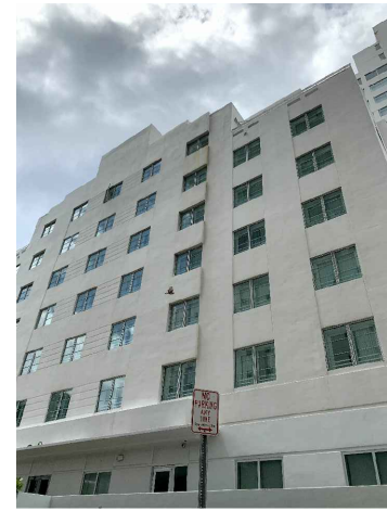
VIEW OF NORTH ELEVATION OF FORMER CROMWELL
