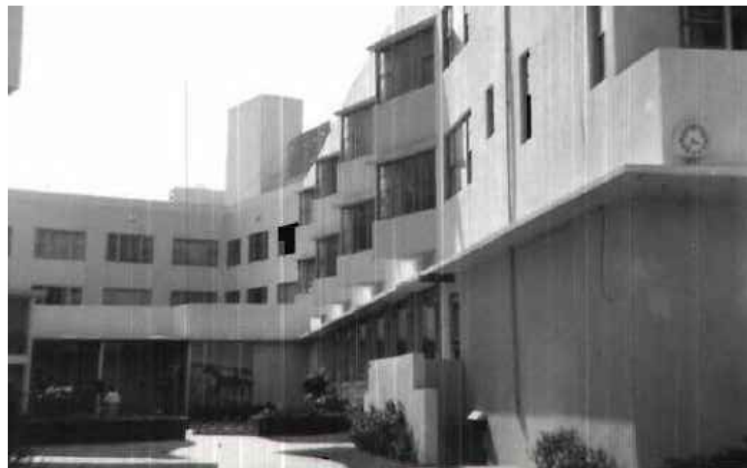
VIEW OF COURTHYARD AREA, c. 1951
