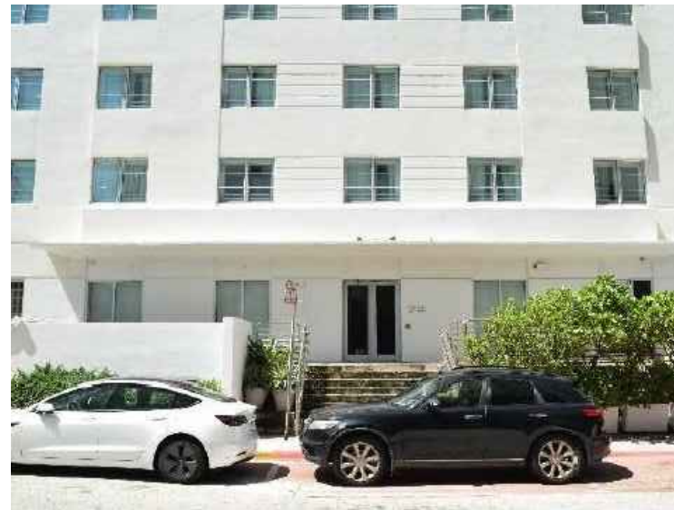
DETAIL OF BASE AT NORTH ELEVATION ENTRANCE
