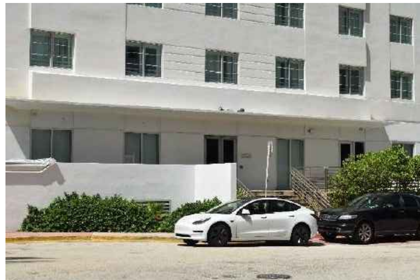
DETAIL OF FRONT WALL AT NORTH ELEVATION
