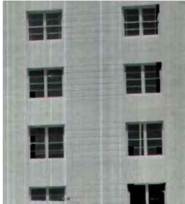
DETAIL OF ORIGINAL WINDOW MUNTING PATTERN, c. 1951
