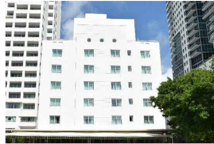
DETAIL OF FENESTRATION PATTERN AT EAST ELEVATION
