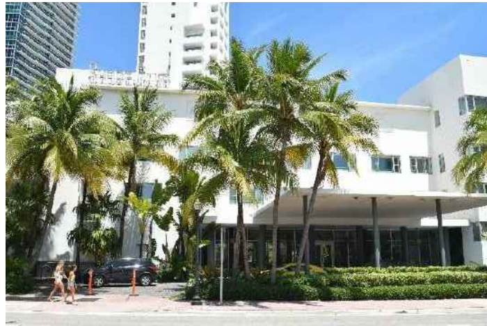
VIEW OF 3-STORY HORIZONTAL BLOCK, WEST ELEVATION, SHORE CLUB
