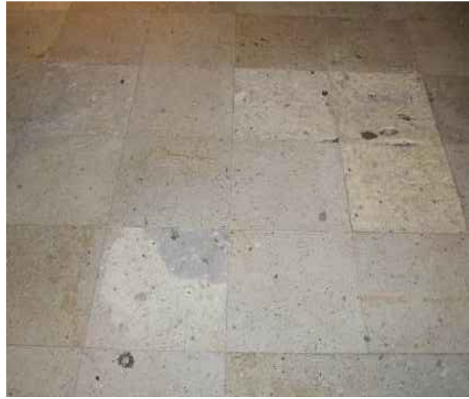
DETAIL OF FLOORING IN LOBBY
