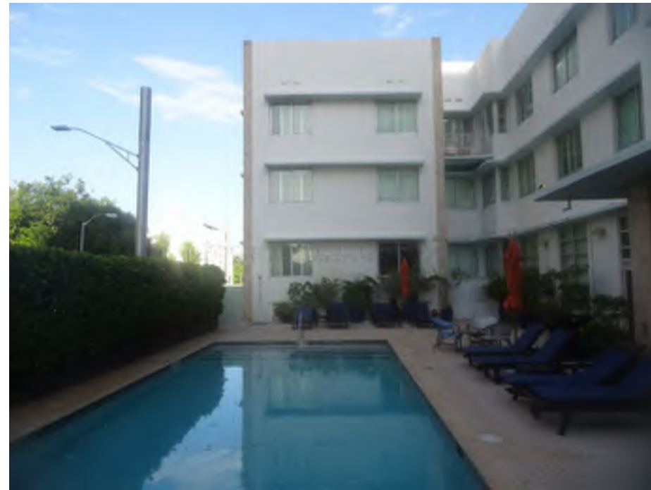
INTERIOR COURTYARD LOOKING WEST- 01.14.2022
