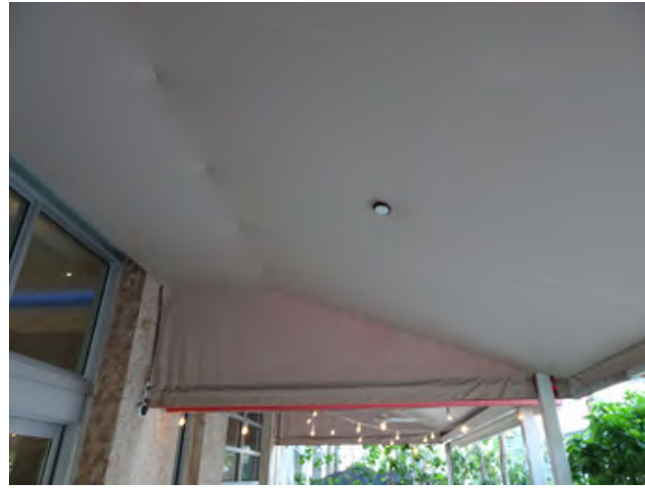
FRONT PORCH FABRIC AWNING- 01.14.2022
