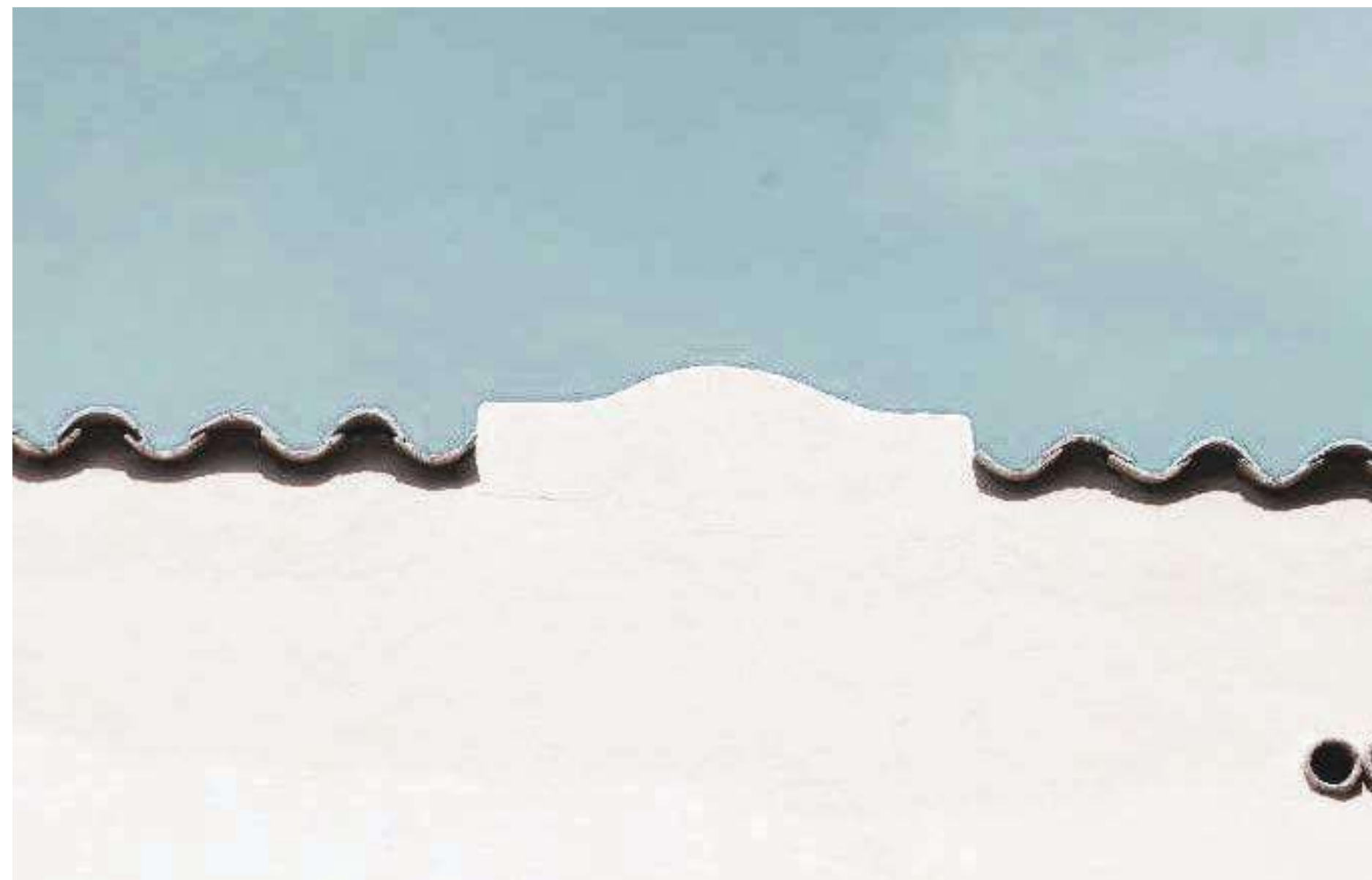
Front Facade Detail SCALLOPED PARAPET
