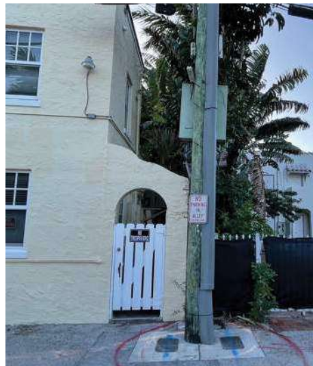
EXISTING VIEW FROM ALLEY LOOKING TOWARDS 927 4TH ST.
