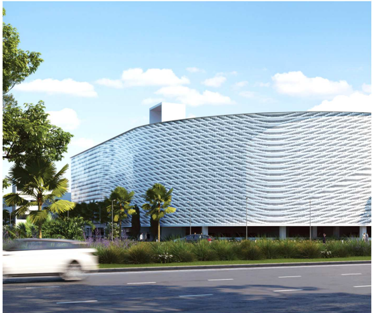
Optical Surface Depth: From a distance the perforated pattern retains 3-dimensional legibility
