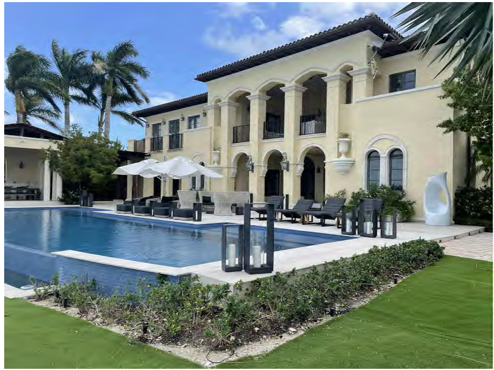
16 4580 PROPERTY - VIEW AT REAR TOWARDS HOUSE (SW CORNER) 2021-11-19
