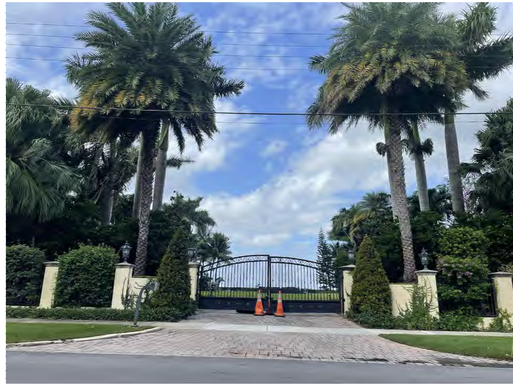
13 VACANT PROPERTY - VIEW AT FRONT GATE 2021-11-19
