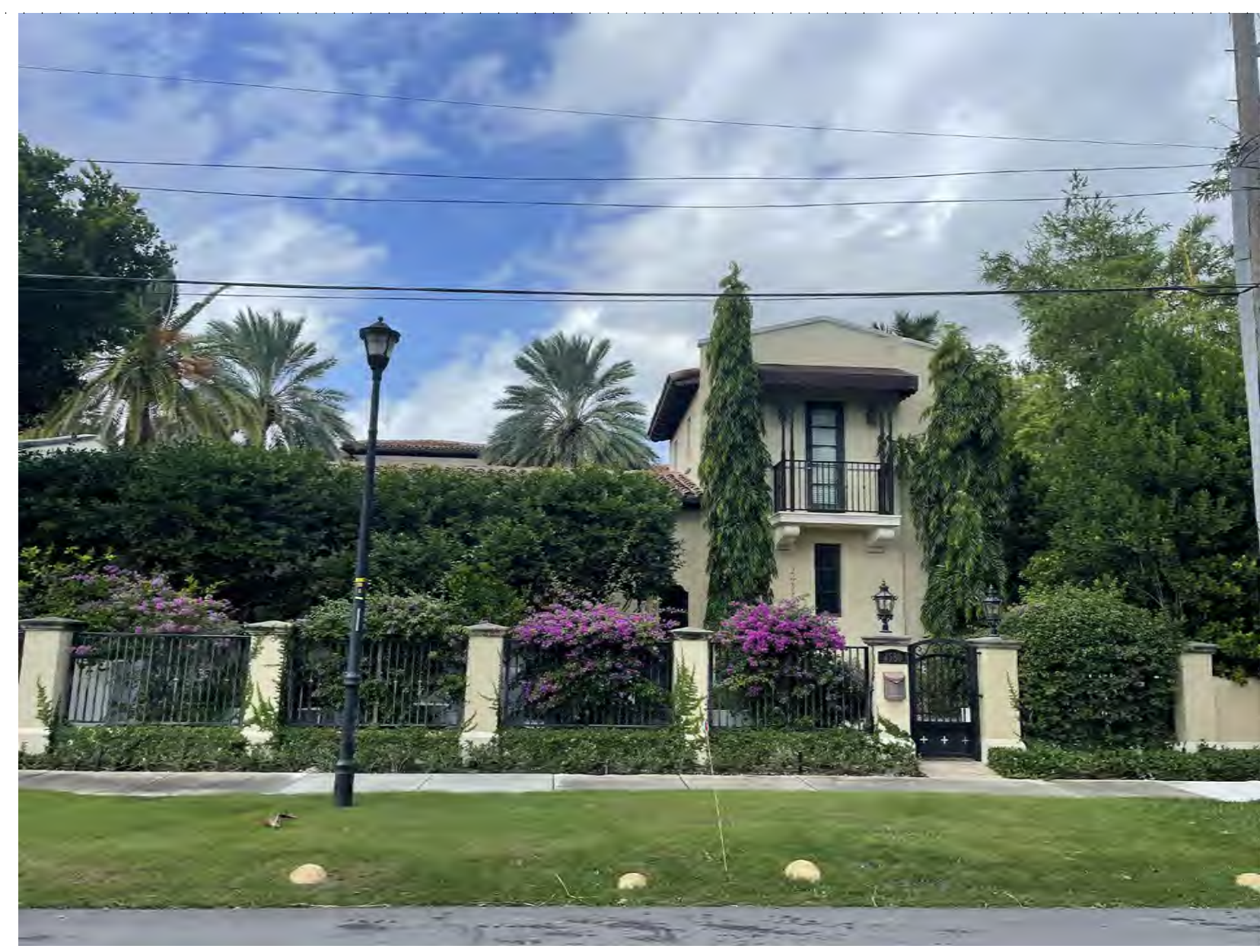
11 4580 PROPERTY - VIEW AT FRONT SITE WALL 2021-11-19
