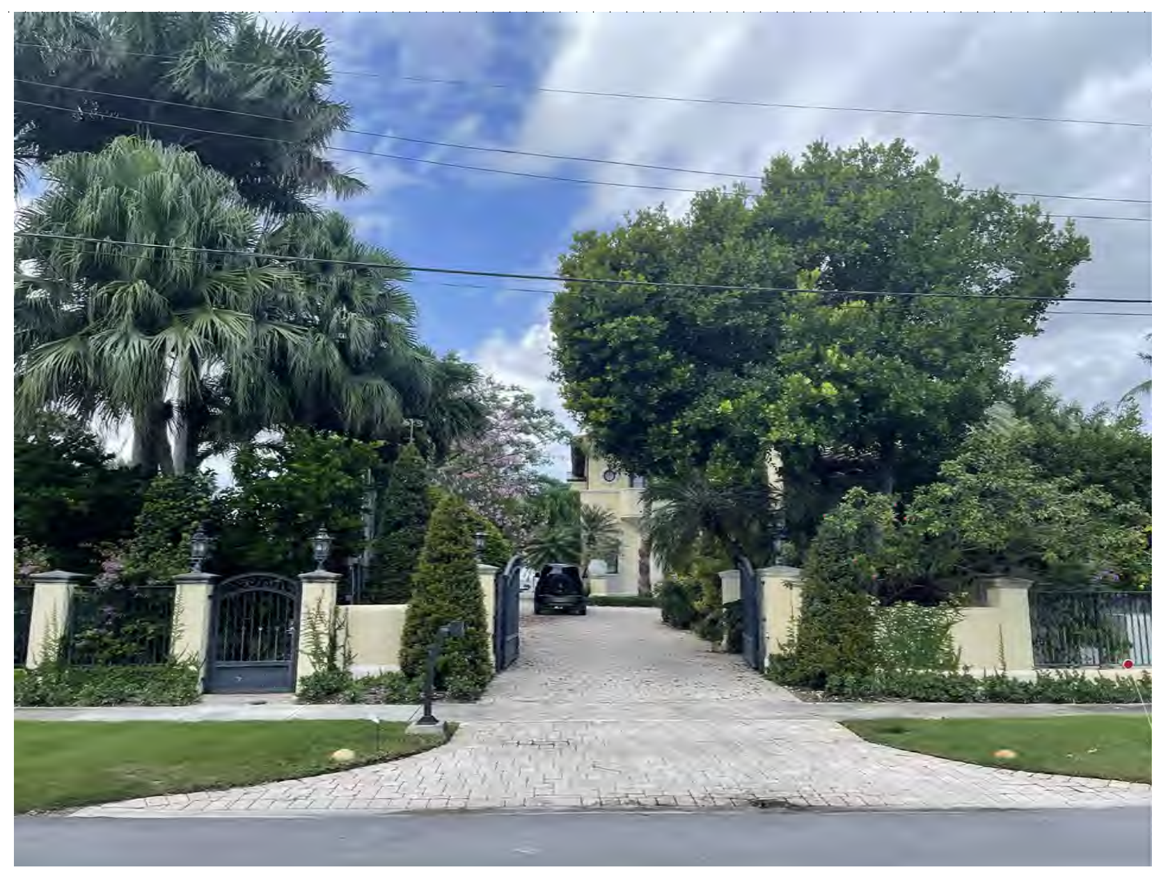
10 4580 PROPERTY - VIEW AT FRONT GATE 2021-11-19
