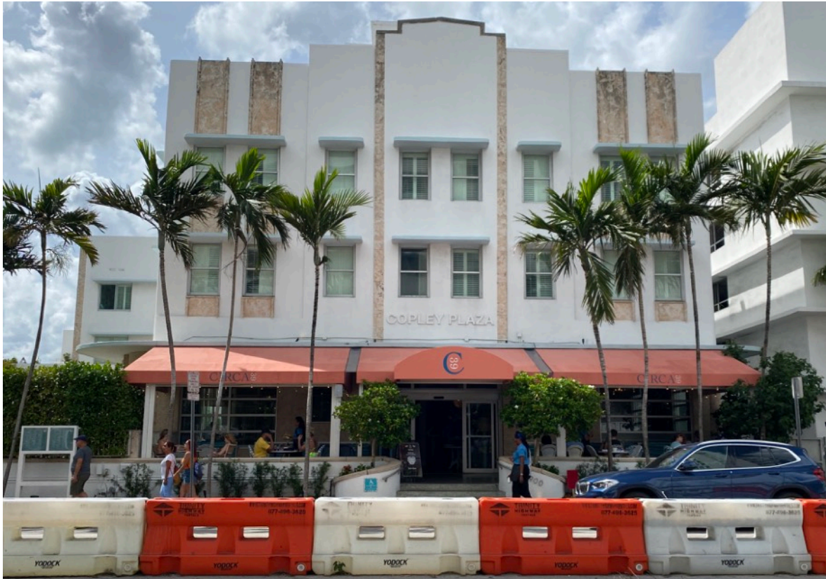
PHOTO ABOVE: FRONT (EAST) ELEVATION OF CIRCA 39 HOTEL FROM COLLINS AVENUE
