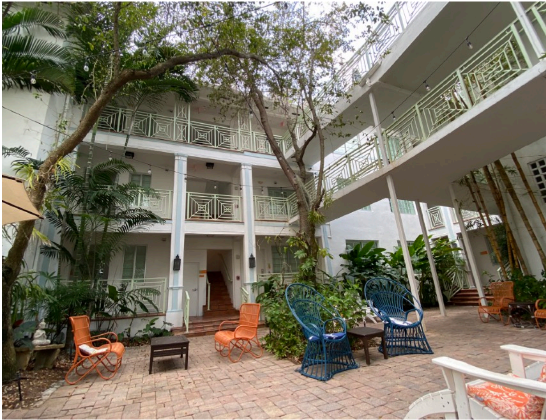
INTERIOR COURTYARD BETWEEN THE TWO BUILDINGS
