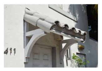
Fig. 18. Detail of pent roof with barrel tile and knee braces at entrance door, May 2021.
