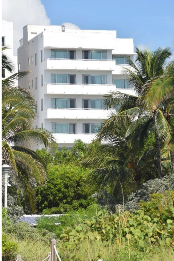
Fig. 182. View of east elevation, looking west, July 2021.
