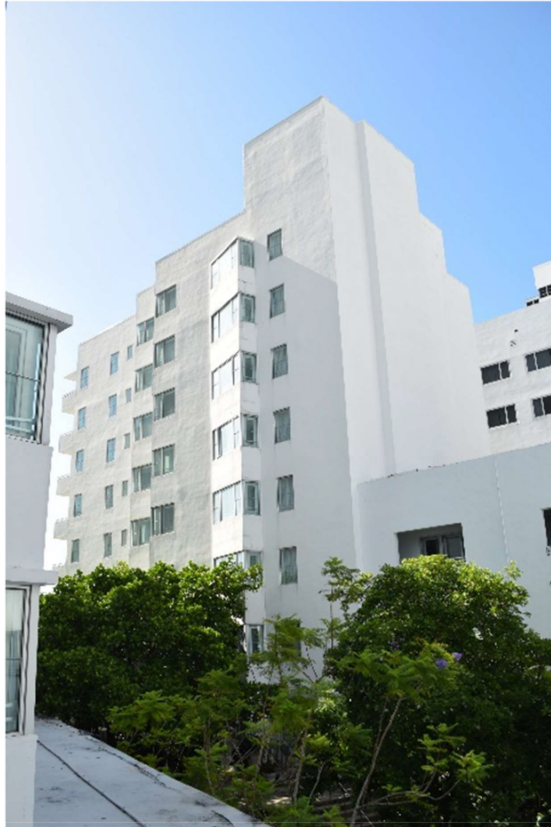
Fig. 179. View of north elevation of 1955 Shore Club Tower, looking southeast, July 2021.
