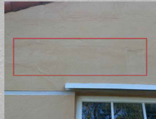
Wall Cracks
