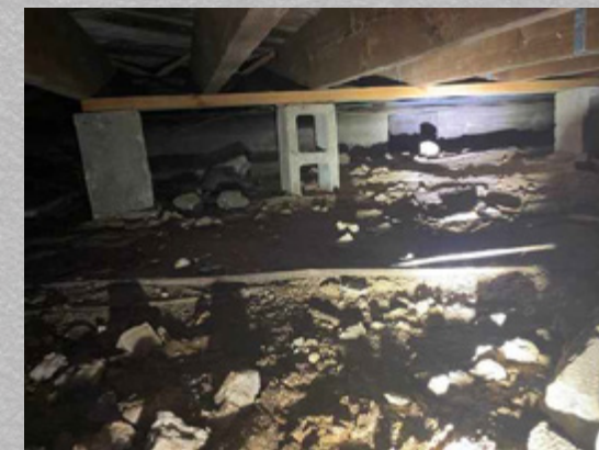
Improper Bracing
