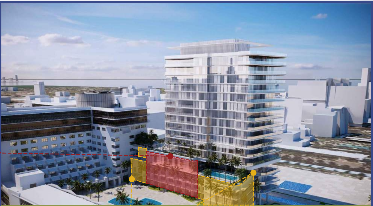
9. New Tower over existing cabana building.
